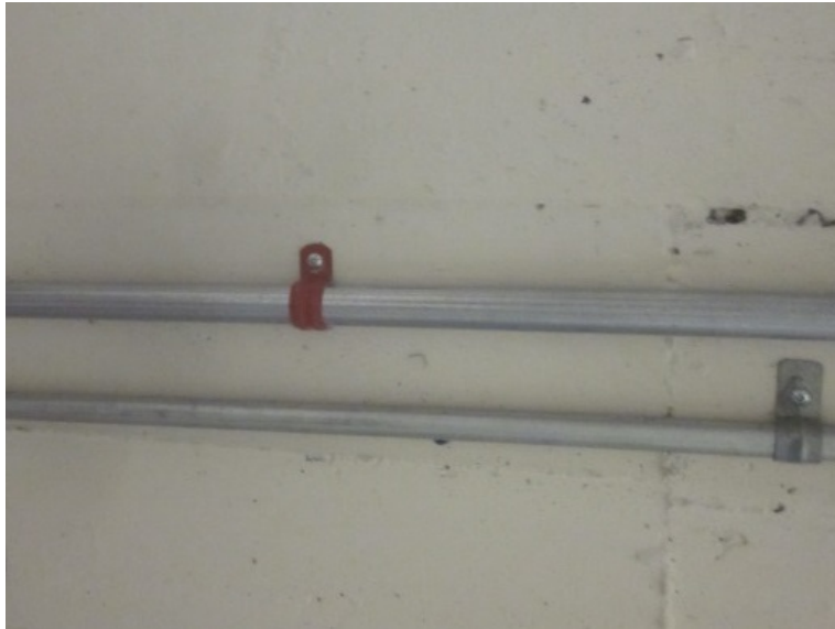
Figure A.1. Typical exempt wall or ceiling mounted conduit
