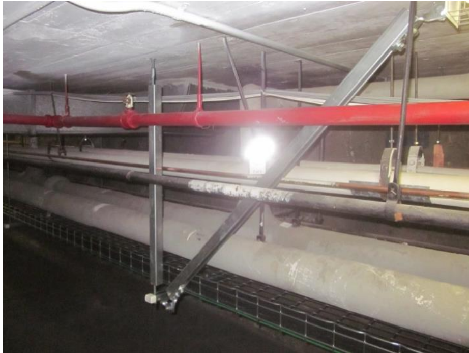
Figure A.29. Restrained cable tray in the basement
