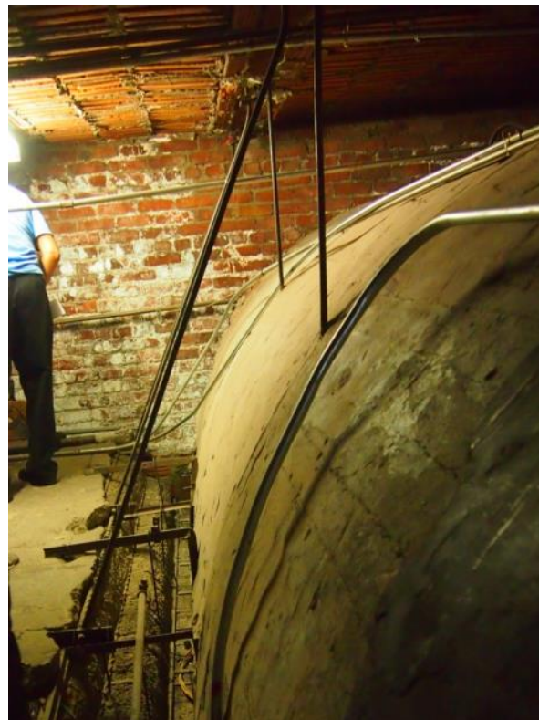
Figure A.12. Support for suspended arched ceiling over the hallway.
