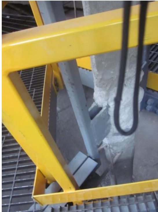
Figure A.15. Connection of attic catwalk around the skylights
