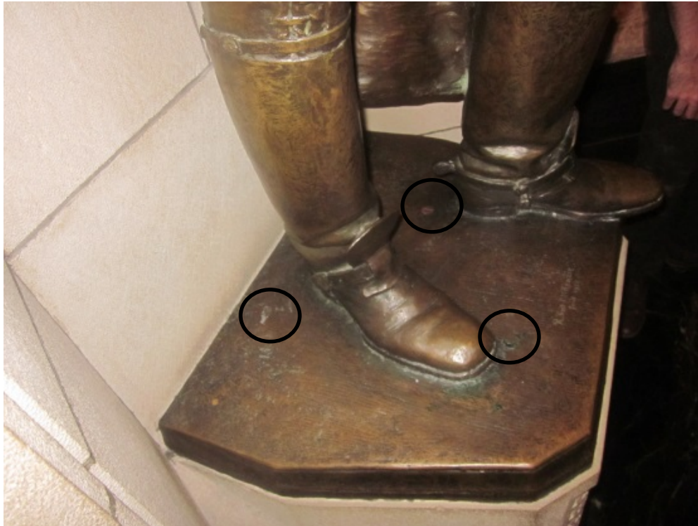
Figure A.23. Nominal connections between the statue and the base
