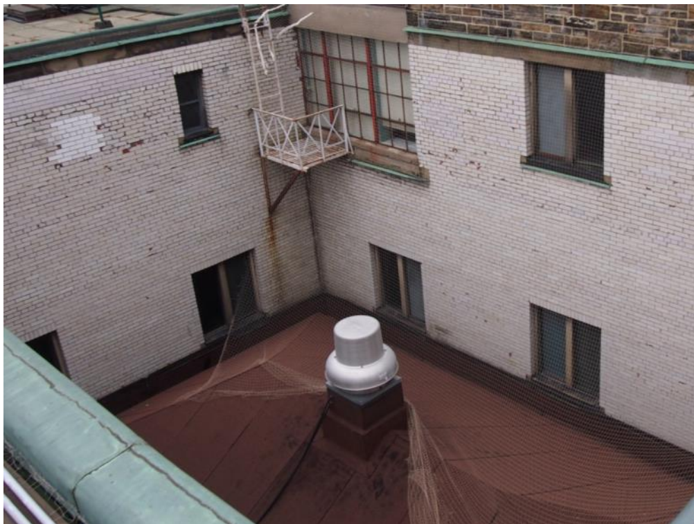
Figure A.6. Brick cladding at lightwells requiring seismic restraint
