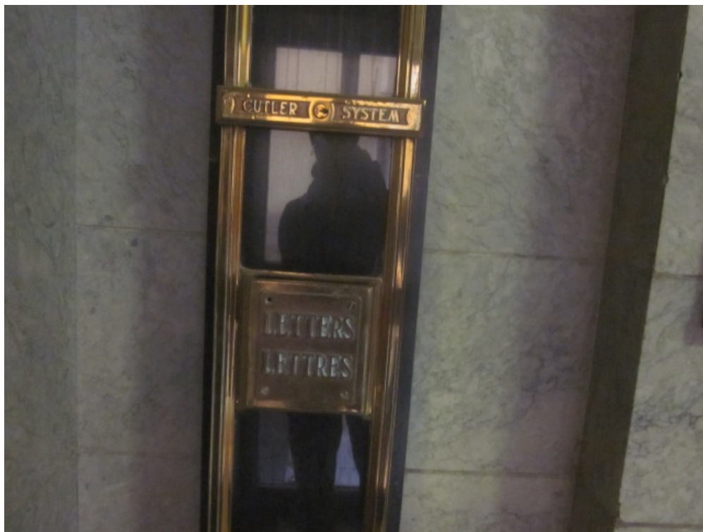
Figure A.24. Wall mounted letter chute requiring seismic restraint
