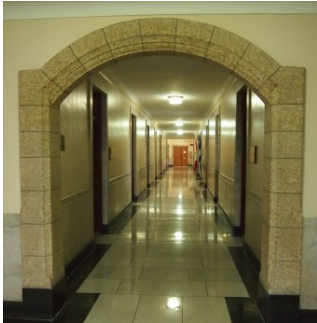
Figure A.19. Decorative arch suspended with the arched plaster ceilings
