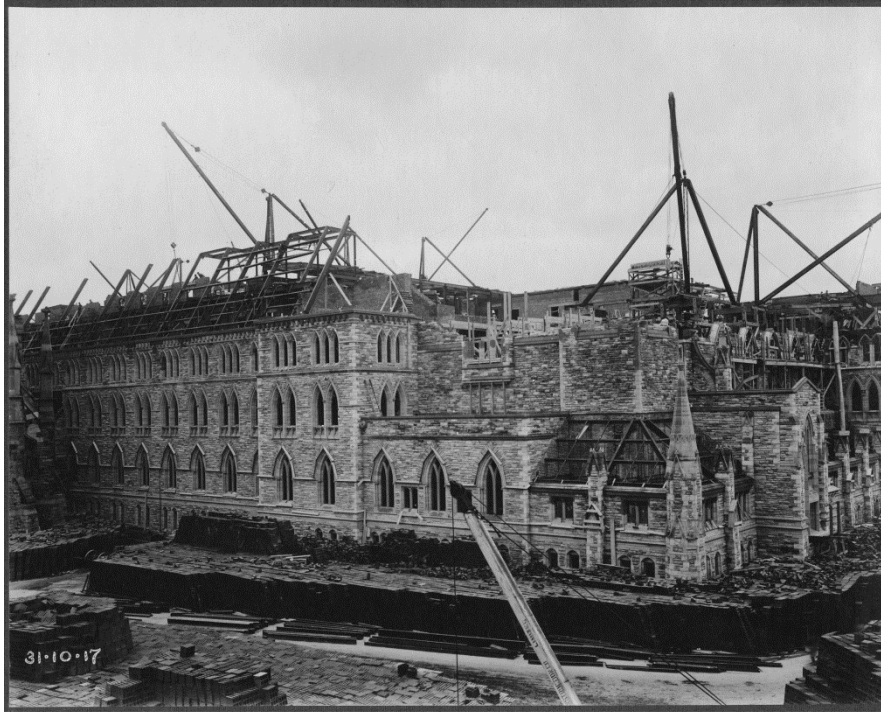
Figure 6.13: Sloped Roof Construction
