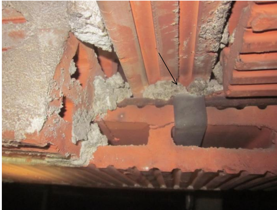
Figure A.9. Connection of fireproofing terra cotta tiles to the bottom flange of the steel beam
