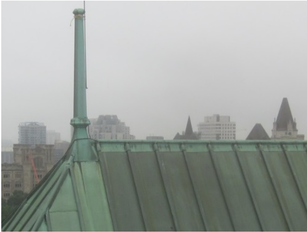
Figure A.5. Typical welded copper roof ornamentation
