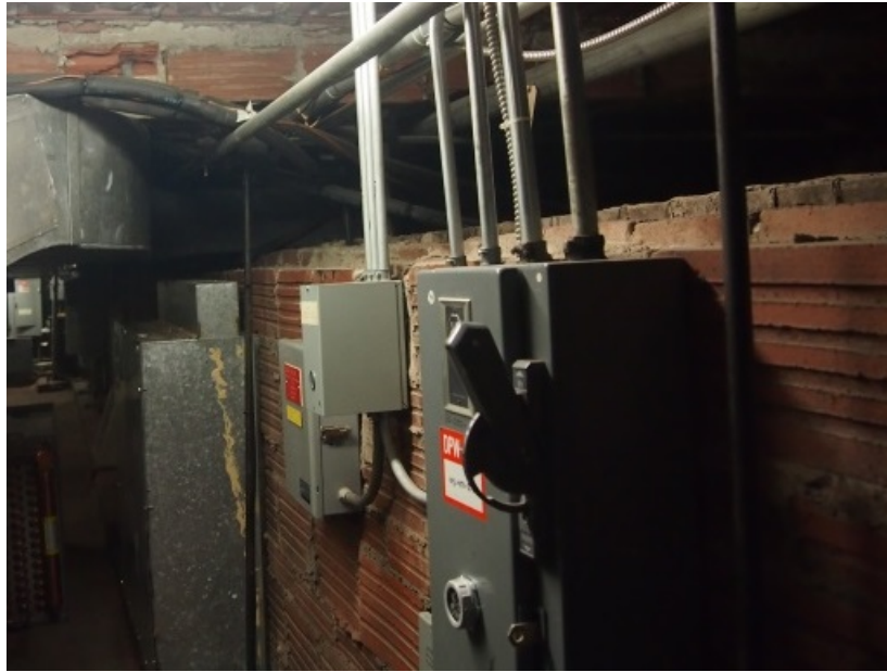
Figure A.21. Partial height terra cotta partition wall requiring seismic restraint
