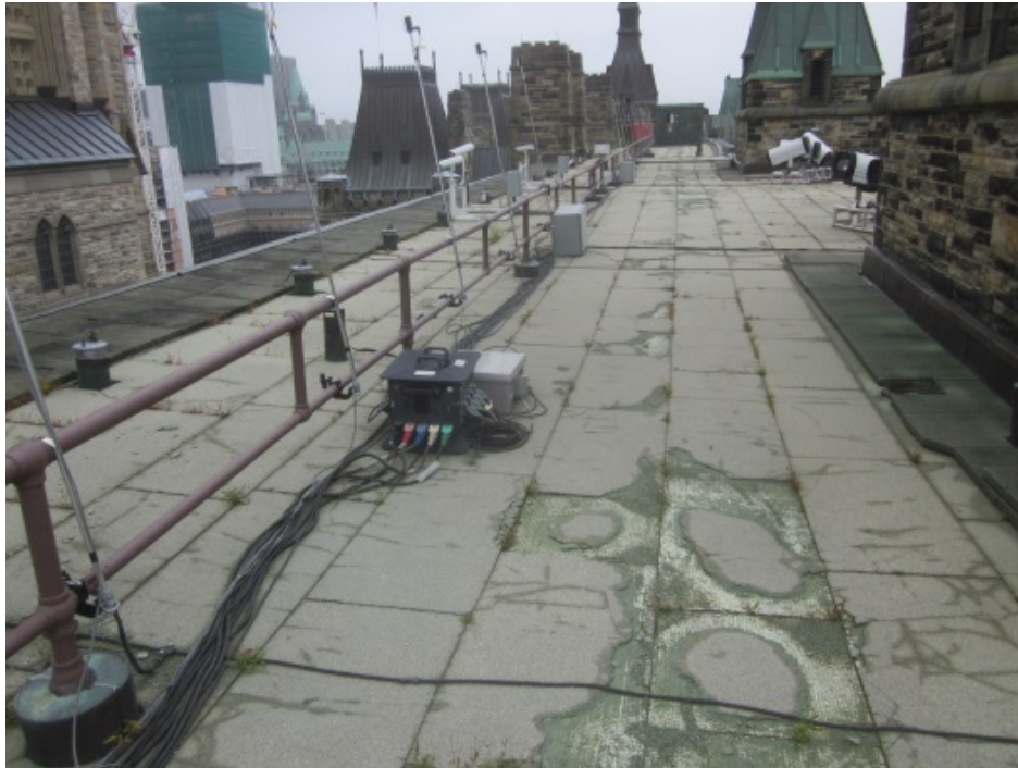
Figure A.3. Typical condition of roofing on the flat roof of the Centre Block
