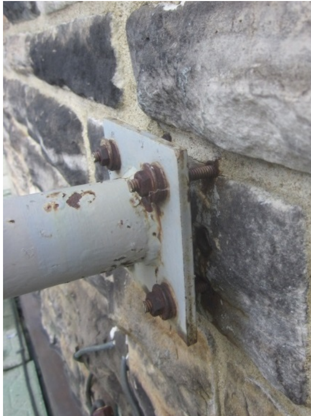
Figure A.7. Typical corroding connections into the wall on the exterior of the Centre Block
