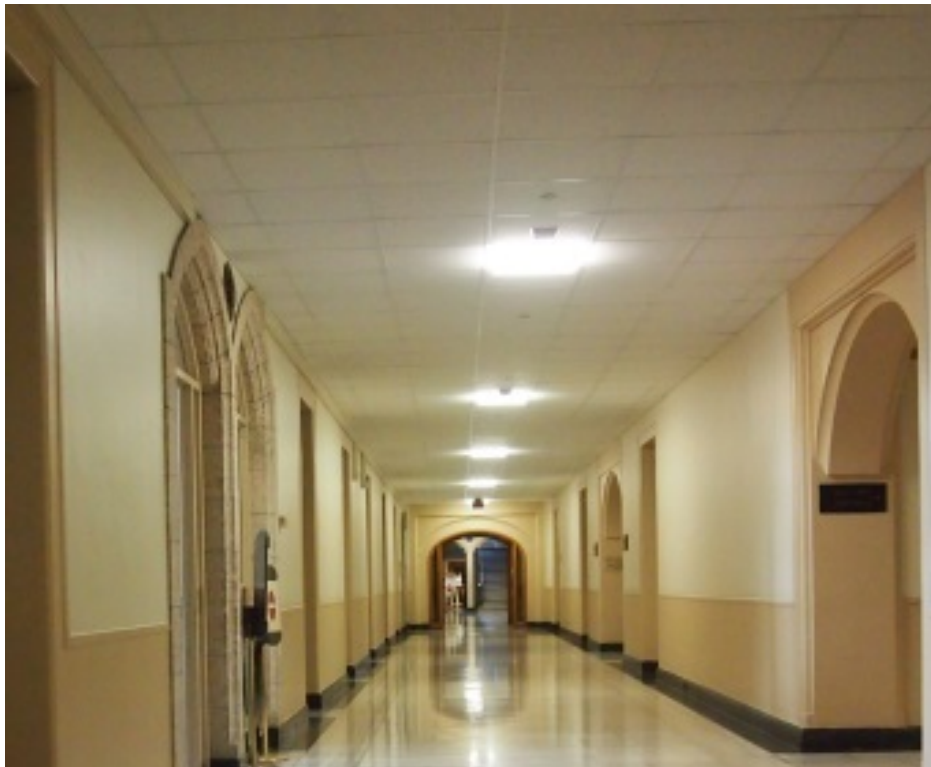
Figure A.18. Typical drop-in tile ceiling in the ground floor hallways
