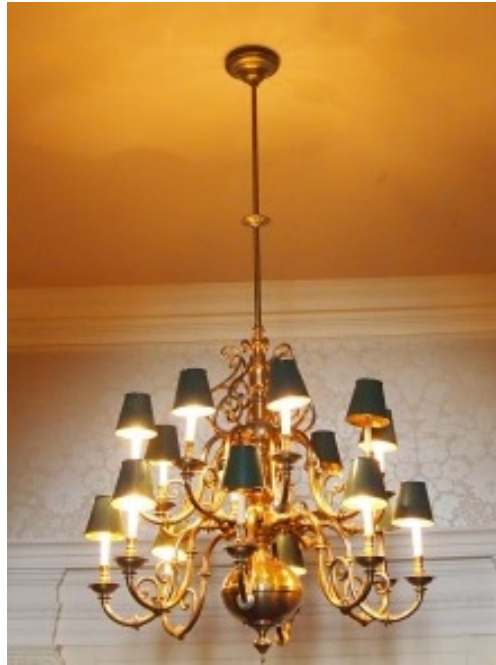
Figure A.25. Large chandelier requiring seismic restraint
