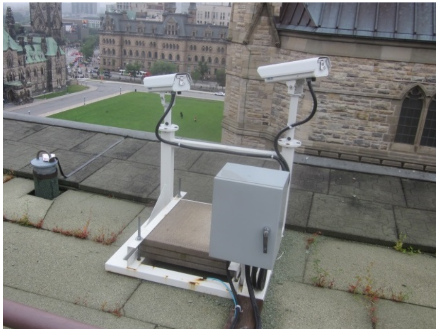
Figure A.8. Typical ballasted frame on the roof of the Centre Block which will require restraint
