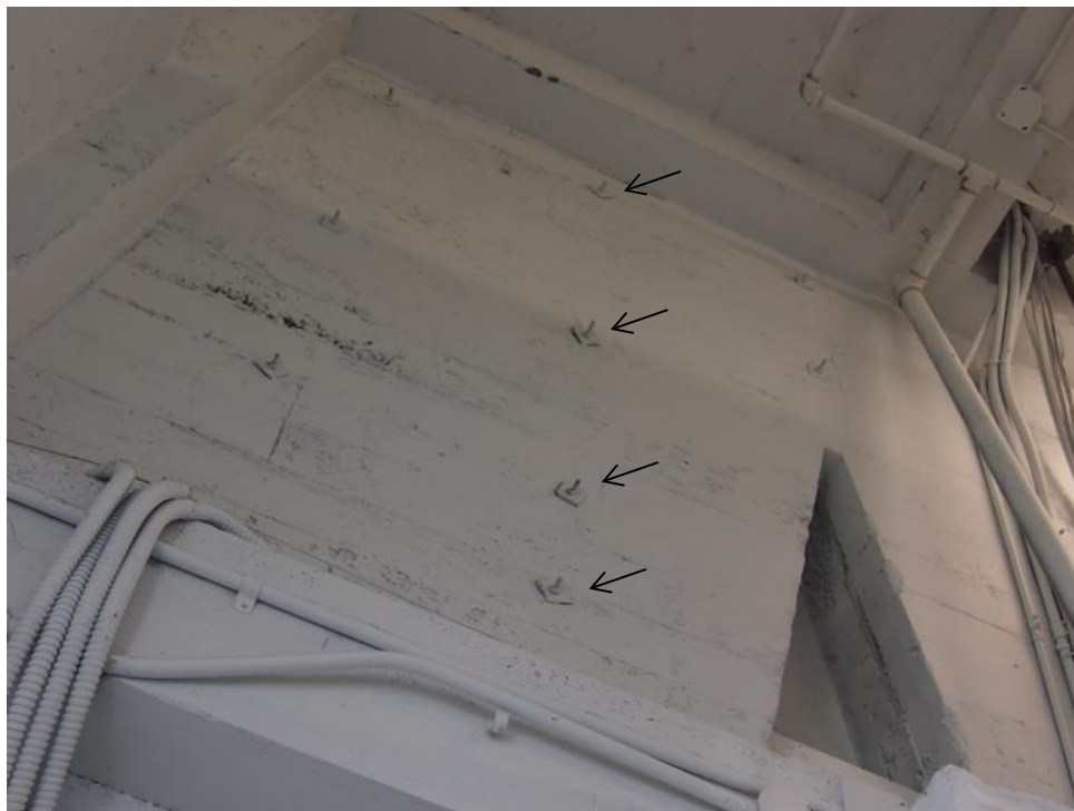
Figure A.4. Typical connections to the copper roofing in the Peace Tower
