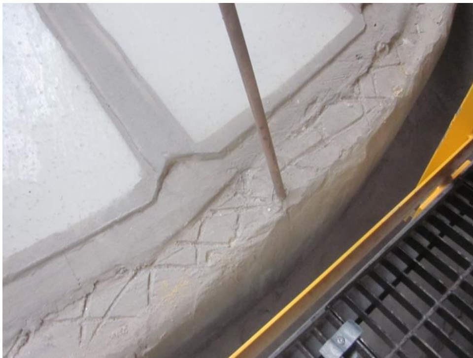
Figure A.14. Typical hanger rod, embedded in the cementitious material above the ceilings
