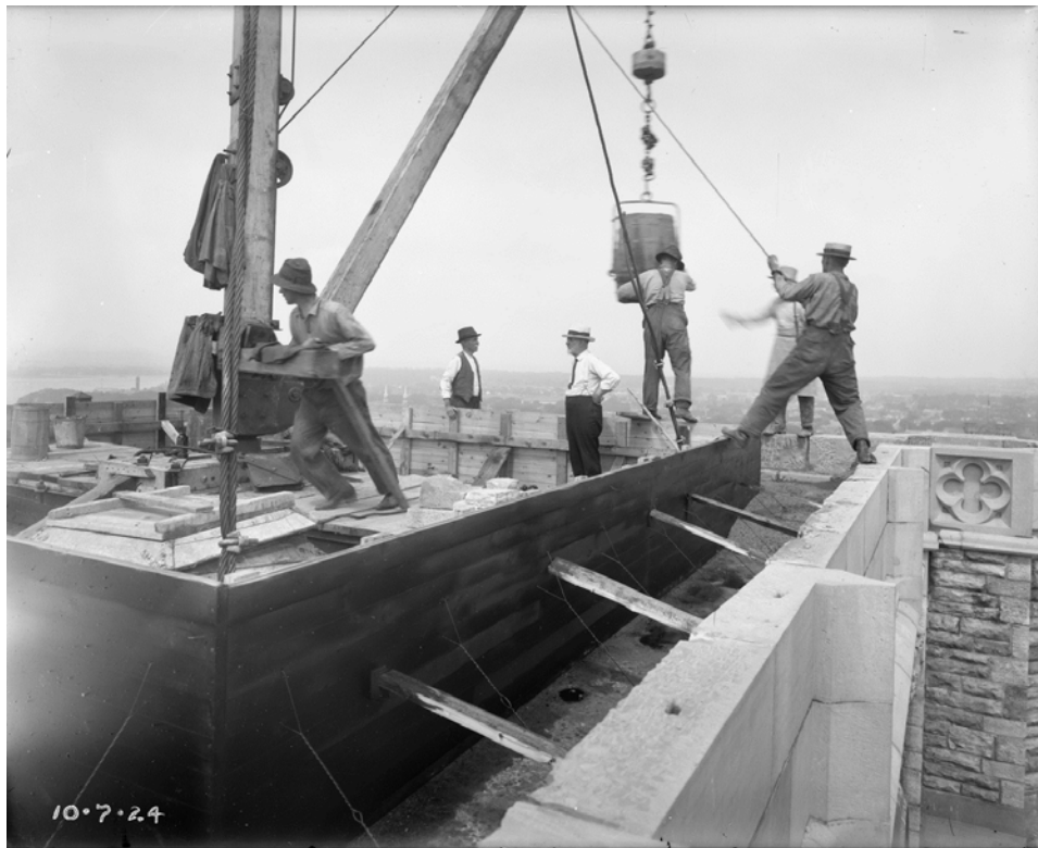
Figure 7.3: Historic photo of concrete being placed behind exterior stone wythe
