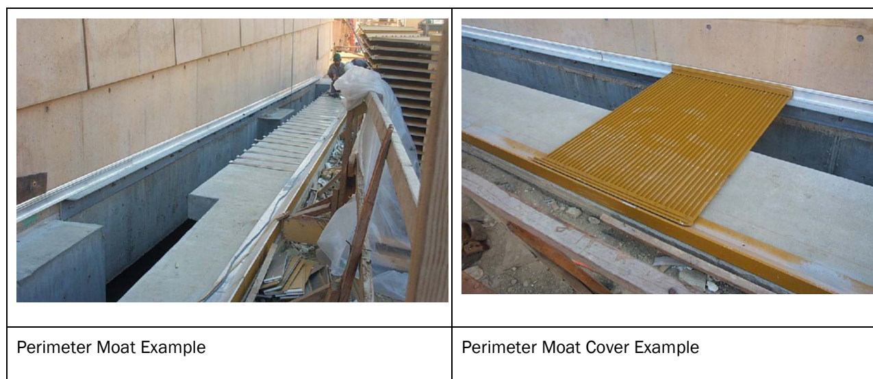
Figure 5-4: Example of Base Isolation Perimeter Moat Construction
