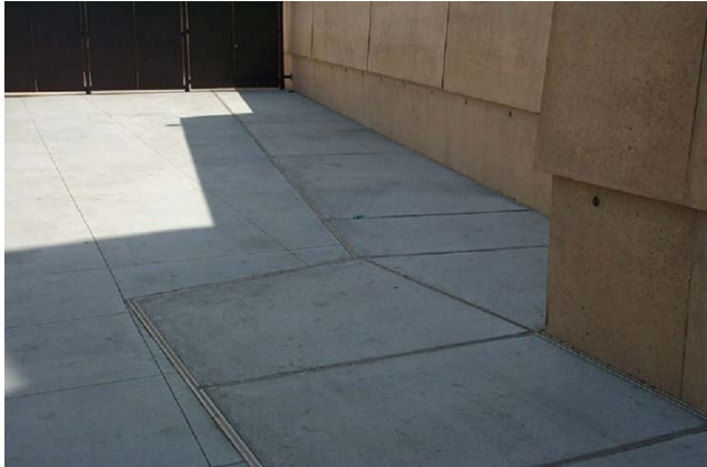
Figure 5-5: Example of finished base Isolation perimeter moat condition
