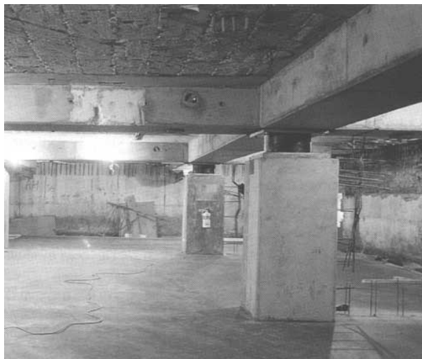
Figure 5-3: Example of seismic isolators at underside of a ground floor slab
