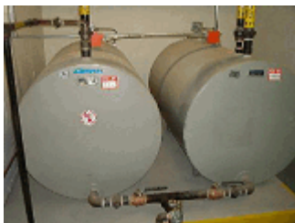
Diesel Storage Tanks.
