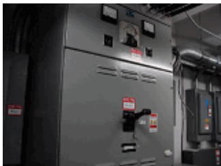
Secondary Switchgear - Panel Z - Main Breaker 400A
