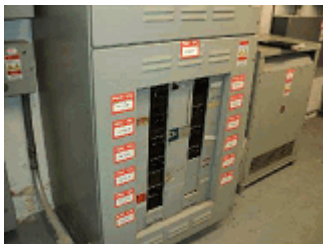
Secondary Switchgear - Panel Z Distribution breakers
