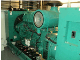
437.5kVA/350Kw Cummins diesel generator
