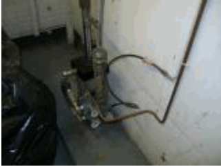
Pneumatic Control Damper
