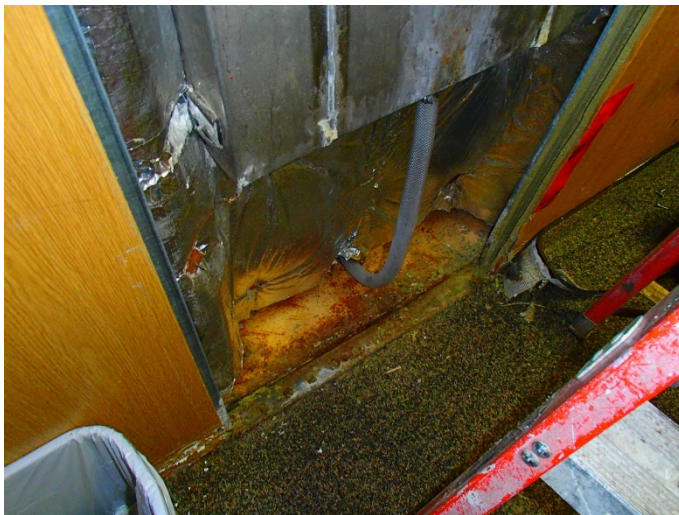
Figure 5: Flexible hose connection under reservoir
