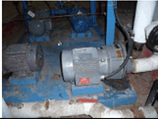
Vacuum Condensate Pumps
