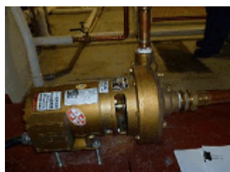
Domestic Hot Water Booster Pump.
