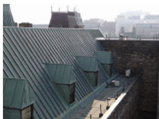
Copper roof on east side of centre block.
