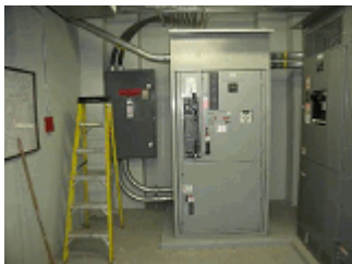
ATS switch located in CBUS.
