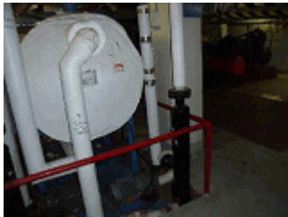
Condensate Vacuum Tank
