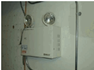
Typical newer model battery lighting.
