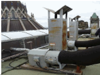
Kitchen exhaust fan on the roof
