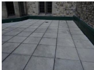
Inverted roof system on senate side at ground level.
