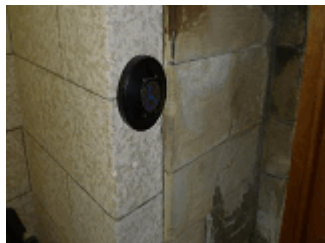
Typical Automated Door Push Button.
