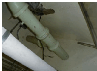
Sanitary drain & Vent piping
