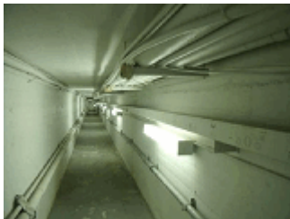
Typical wall mounted fluorescent lighting.
