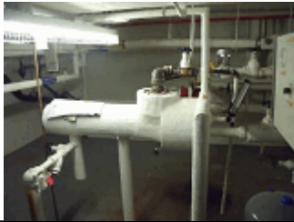
Basement Heat Exchanger
