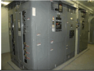
Primary Switchgear.
