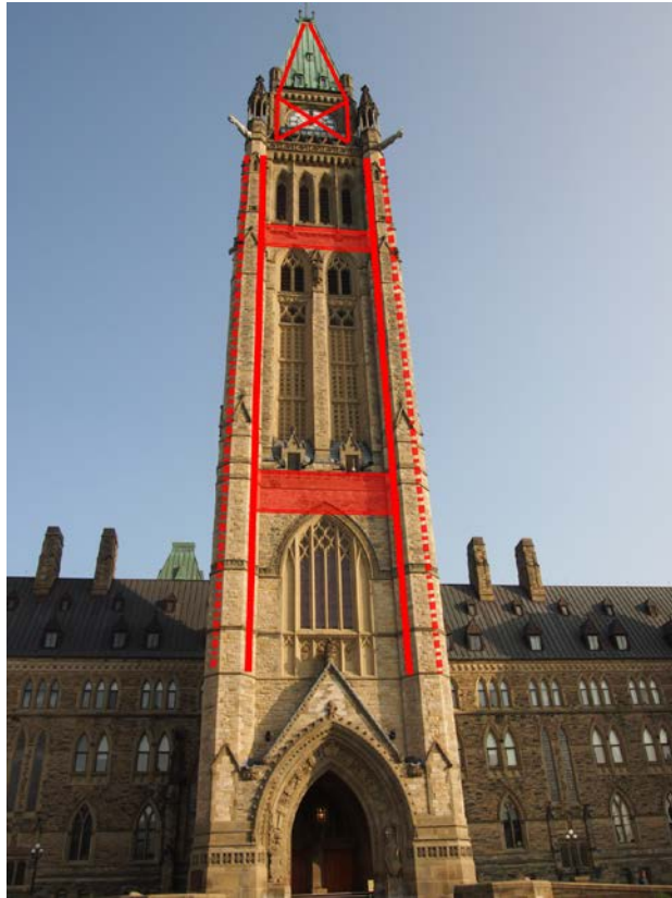
Figure 7 - Schematic layout of Peace Tower reinforcing
