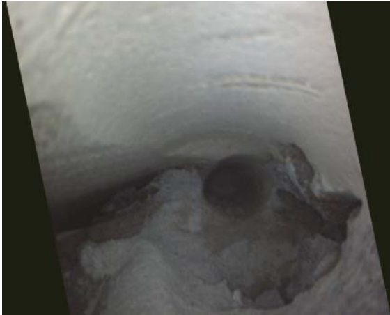
Figure 2-IV: Bore hole with significant voiding.
