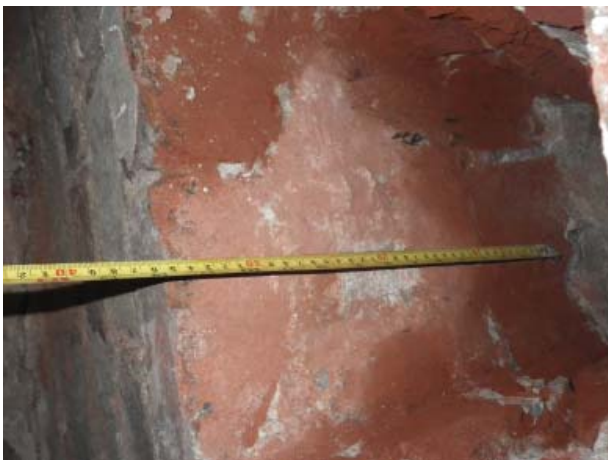
Figure 2-XII: Thickness of backwall at this location.
