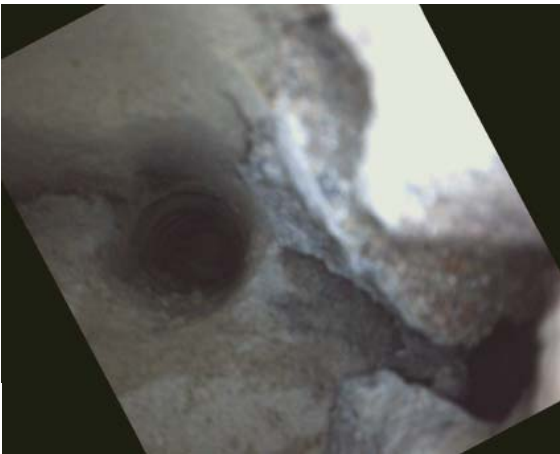
Figure 2-V: Voiding on right side.
