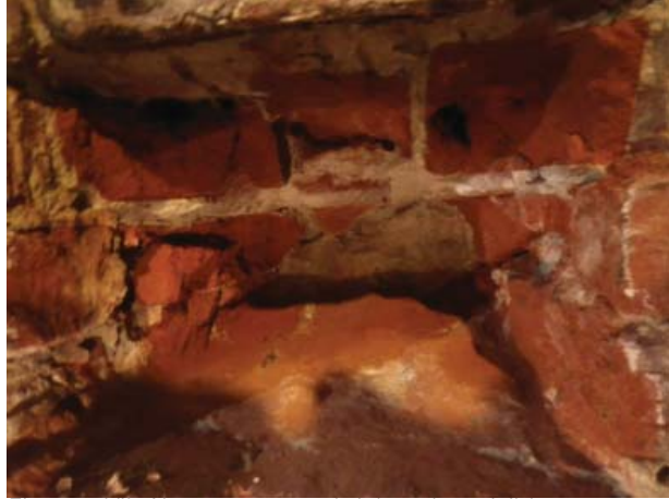
Figure 2-VII: Alternate course brick wythes visible.
