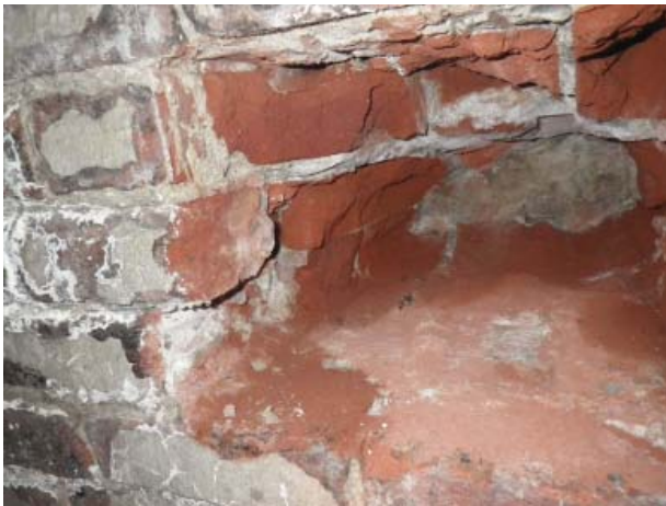
Figure 2-XI: Evidence of humidity towards the face stone.
