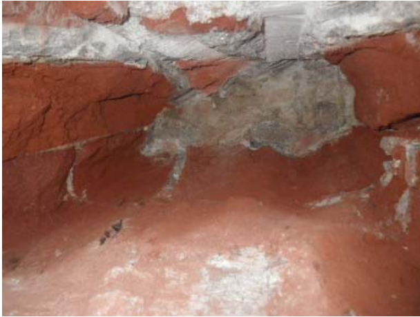
Figure 2-X: Evidence of humidity towards the face stone.
