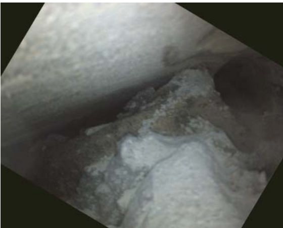
Figure 2-VI: Voiding on right side.
