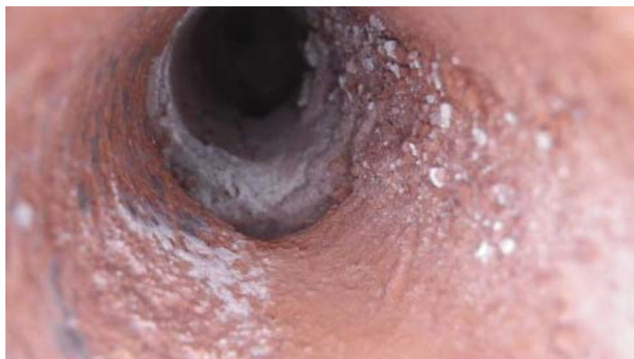
Figure 2-III: Bore hole showing minor voiding around mortar.
