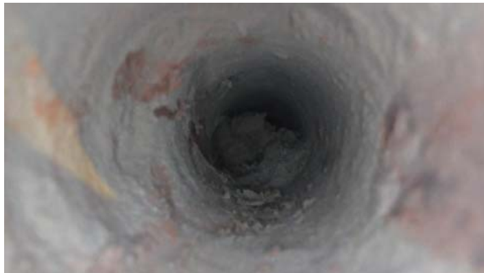
Figure 2-II: Bore hole into the back of face stone.
