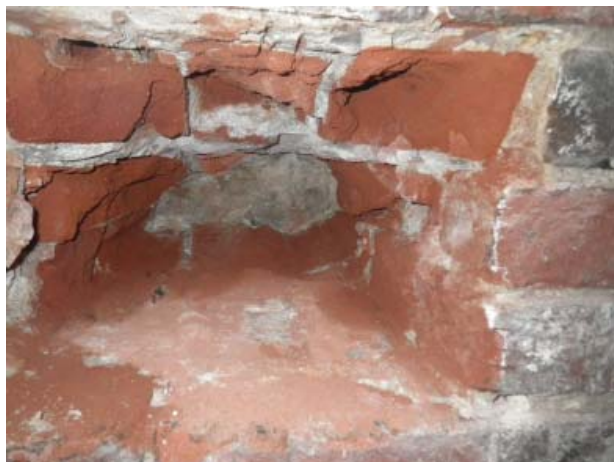
Figure 2-IX: Evidence of humidity towards the face stone.
