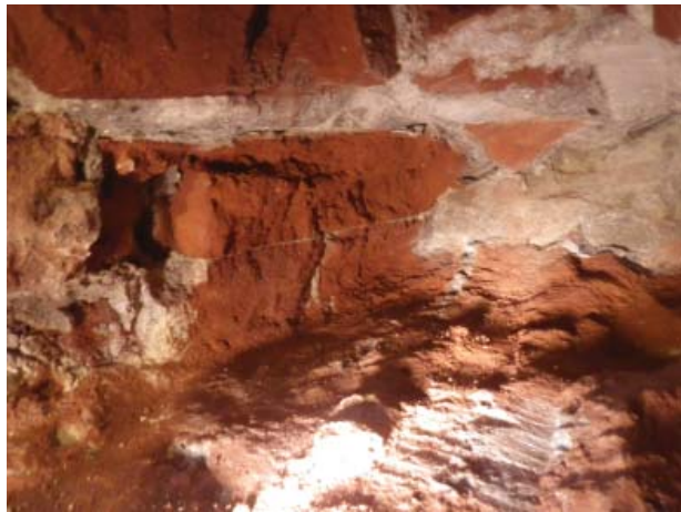
Figure 2-VIII: Excavated until the back of the face stone.
