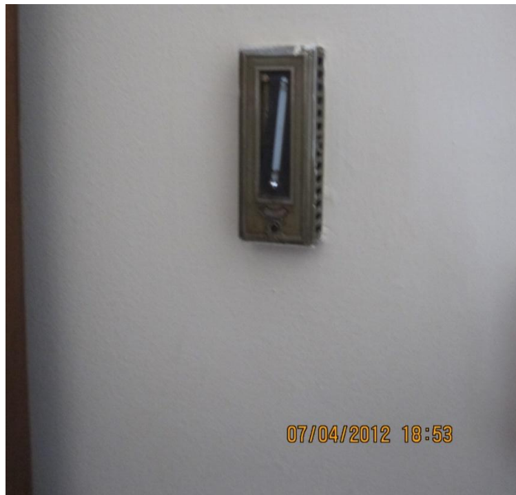
Photo 3: Mercury containing thermostats were observed in select rooms of the building. They were reportedly not in use and were left place following a retrofit of the building.
