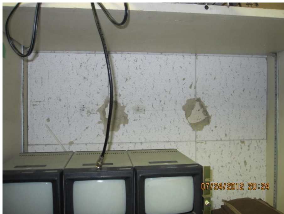
Photo 4: 1' x 1' Acoustic Wall Tiles, (previously sampled, 1998) observed in select areas on the first and third floor contains 0.5-5% Amosite and 5-25% Chrysotile.
