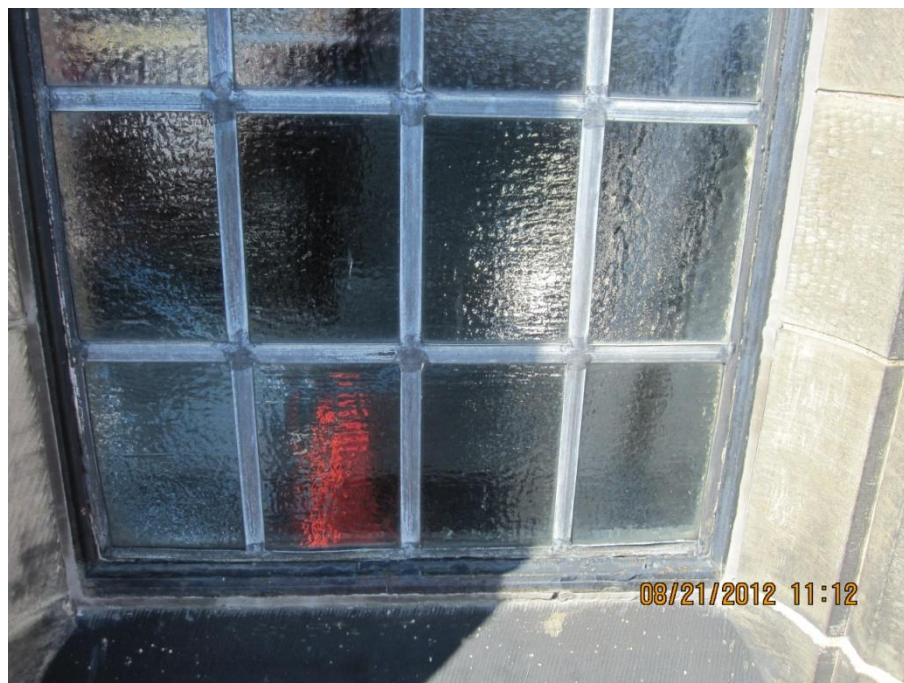
Photo 6: Exterior window, west face of building. Caulking from the outside of these windows was reportedly newer, and was sampled and found to not contain regulated amounts of asbestos.
