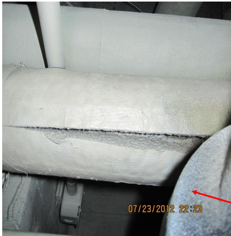
Photo 2: Asbestos-containing aircell (previously sampled) was observed in various locations throughout the building, predominately in the basement.
