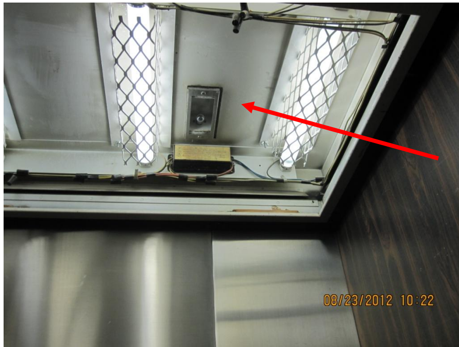
Photo 7: Suspected PCB-containing light ballast was observed in the elevator at the rear of the building. Fluorescent light ballasts associated with the T12 light fixtures in the building are suspected to contain PCBs.
