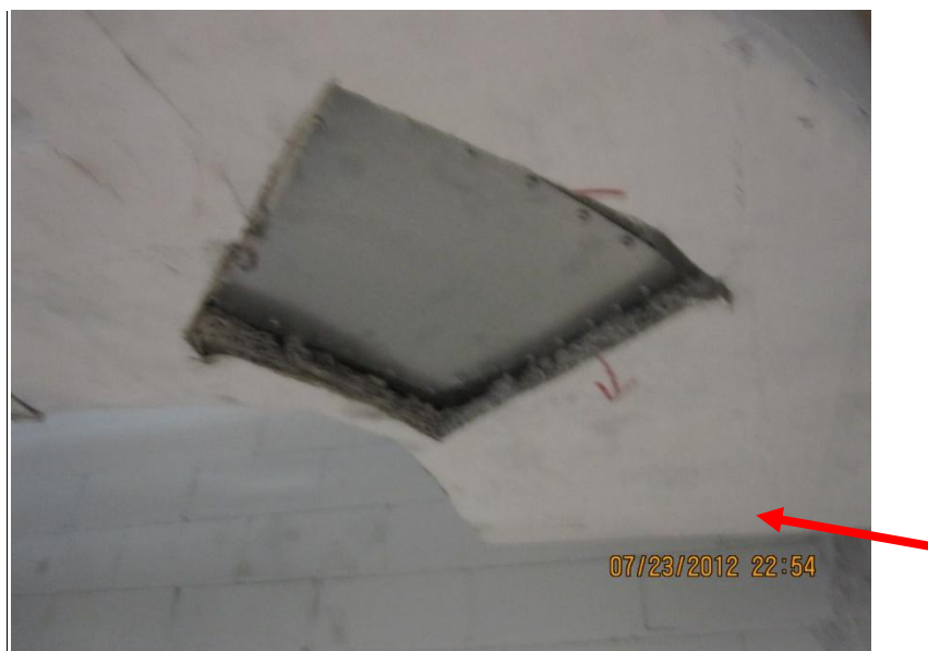
Photo 8: Aircell insulation on ductwork (previously sampled, 1998) contains regulated amounts of asbestos. This material was observed throughout the basement of the building. Small sections were observed in poor/fair condition, as seen above.
