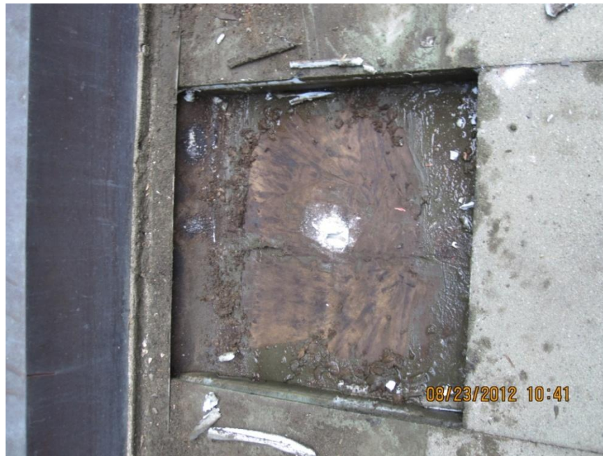
Photo 5: Roofing material, inverted roofing system (Sample 14755-65A-C and 66A-C) sampled from the sixth floor and second floor courtyard were sampled and do not contain regulated amounts of asbestos.
