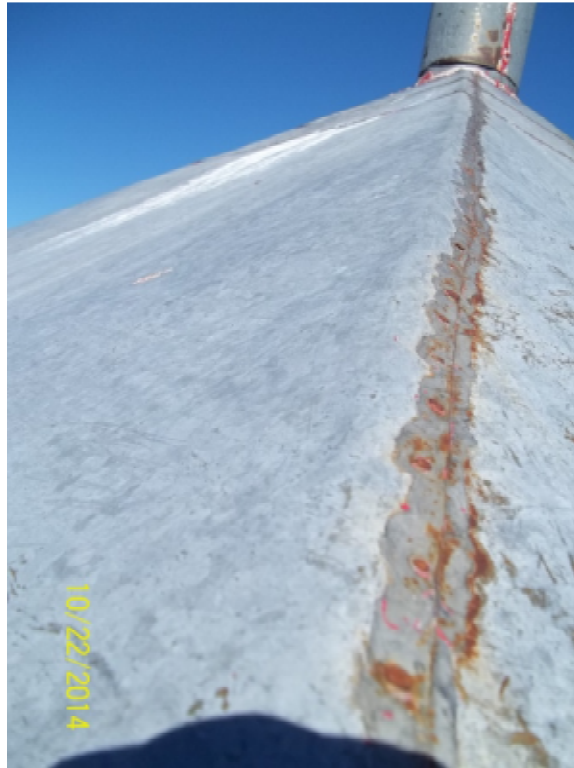
Photo 39: Sheet metal roof over the highest part of the lighthouse roof.
