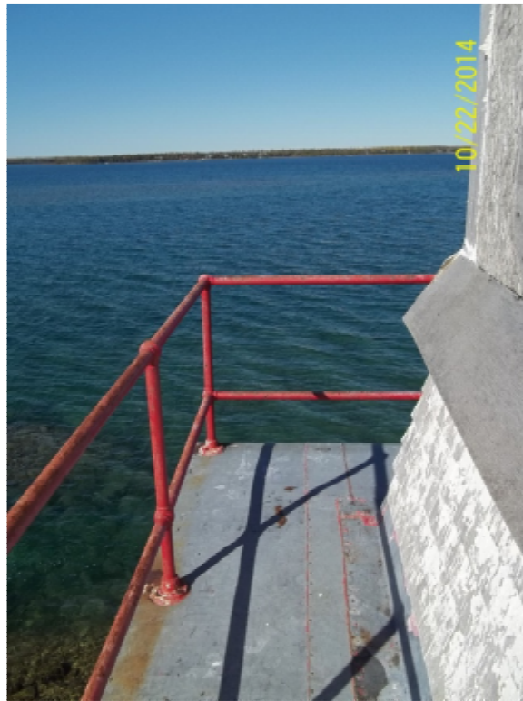
Photo 19: Walkway - view looking north.
