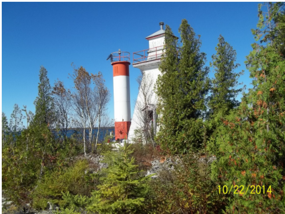
Photo 4: View looking towards the north-northwest.
