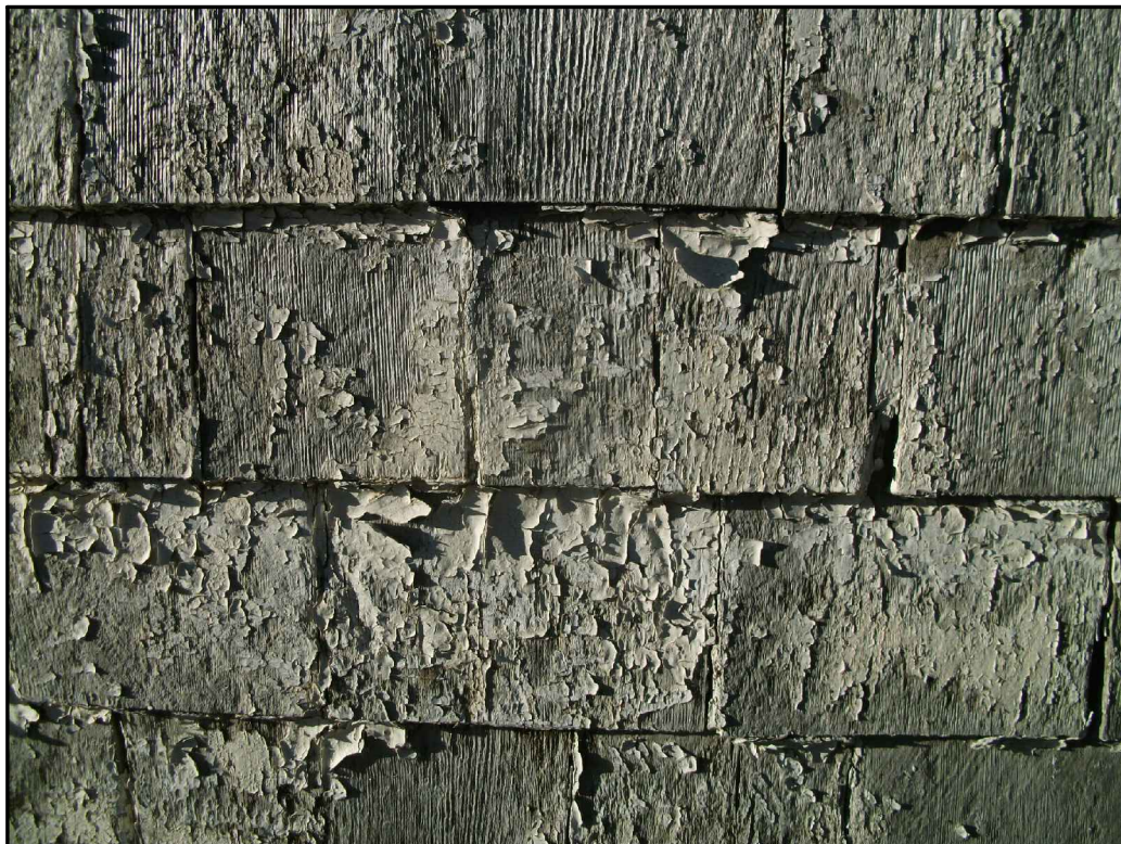
Photograph 12: White lead-based paint (poor condition) on exterior wood surface on west side of 1st floor of Old Light Tower.
