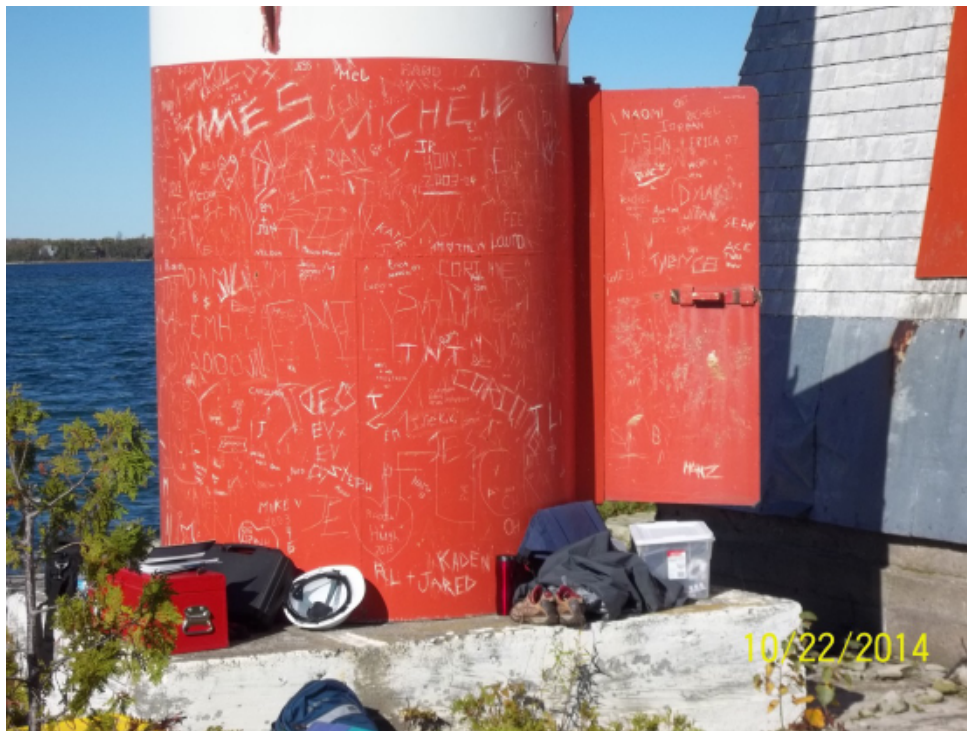
Photo 40: Base of steel tower.
