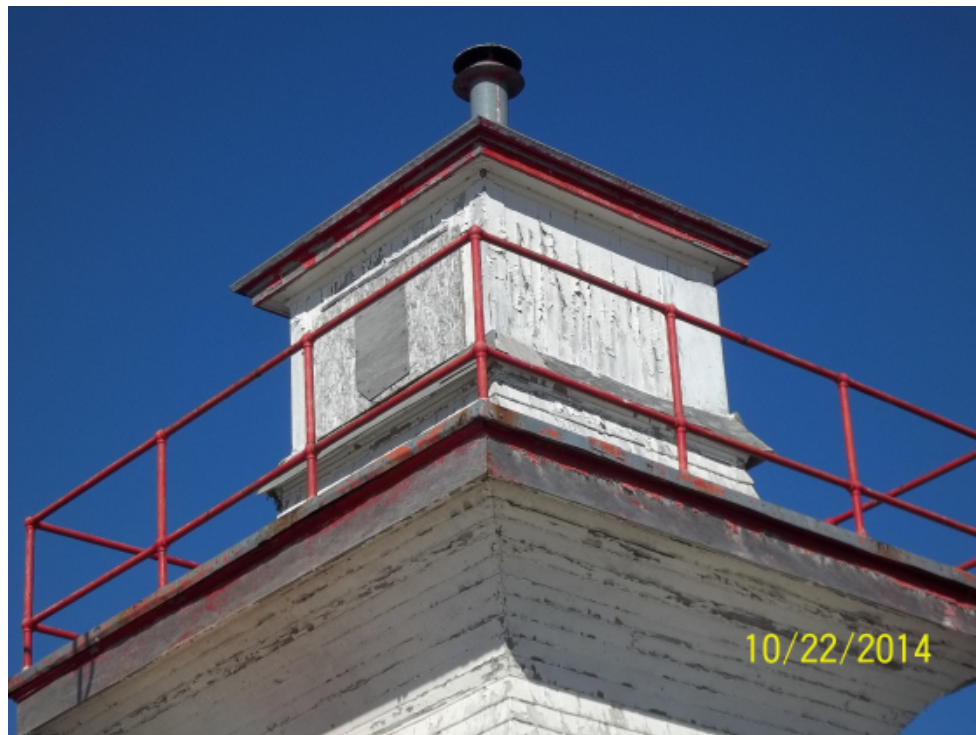
Photo 12: View from the southwest looking at the top of the lighthouse.
