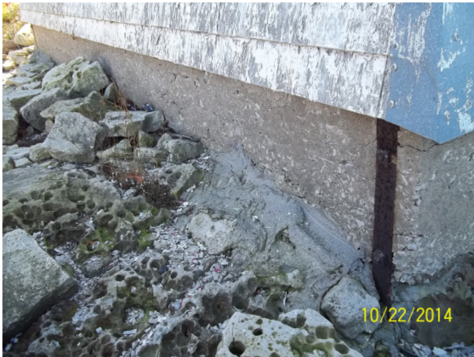
Photo 10: Steel foundation strap at northeast corner.
