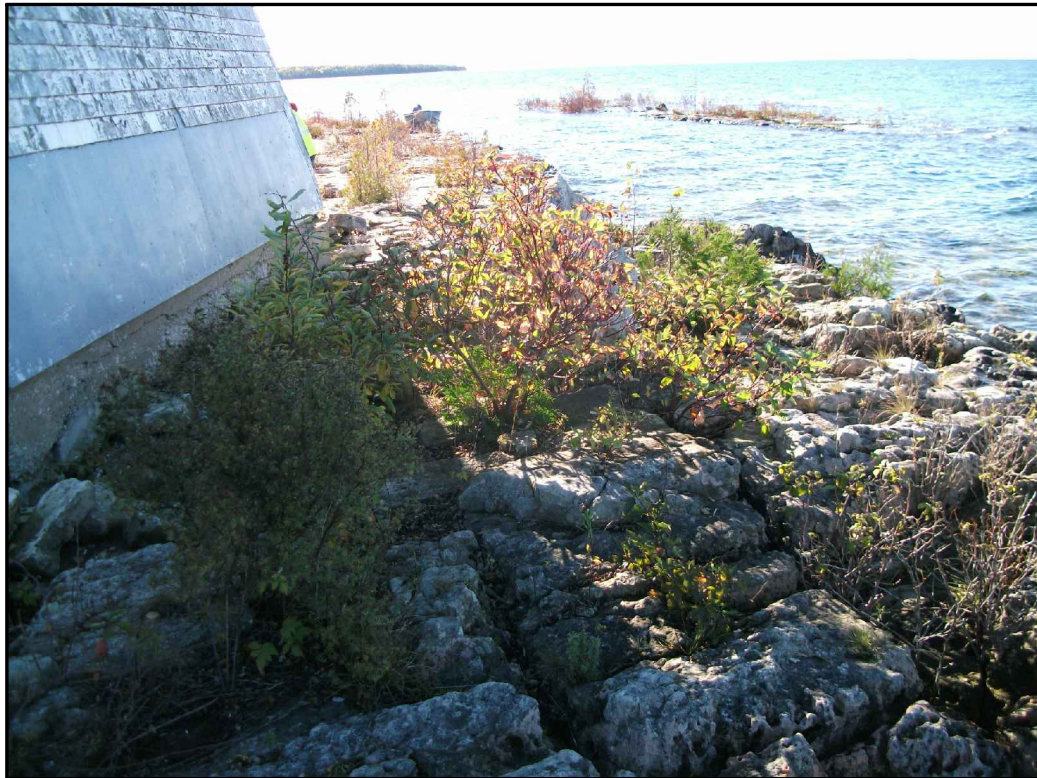
Photograph 18: Limited soil accumulation and vegetation in cracks between bedrock (looking southwest).
