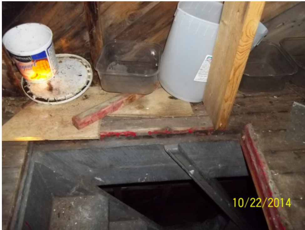
Photo 33: Hatch at upper level looking at base of south wall.
