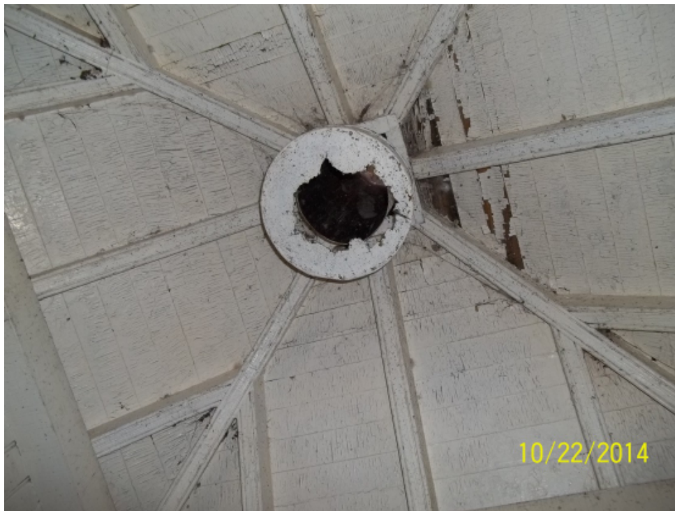
Photo 38: Interior view of the peak of the lighthouse.
