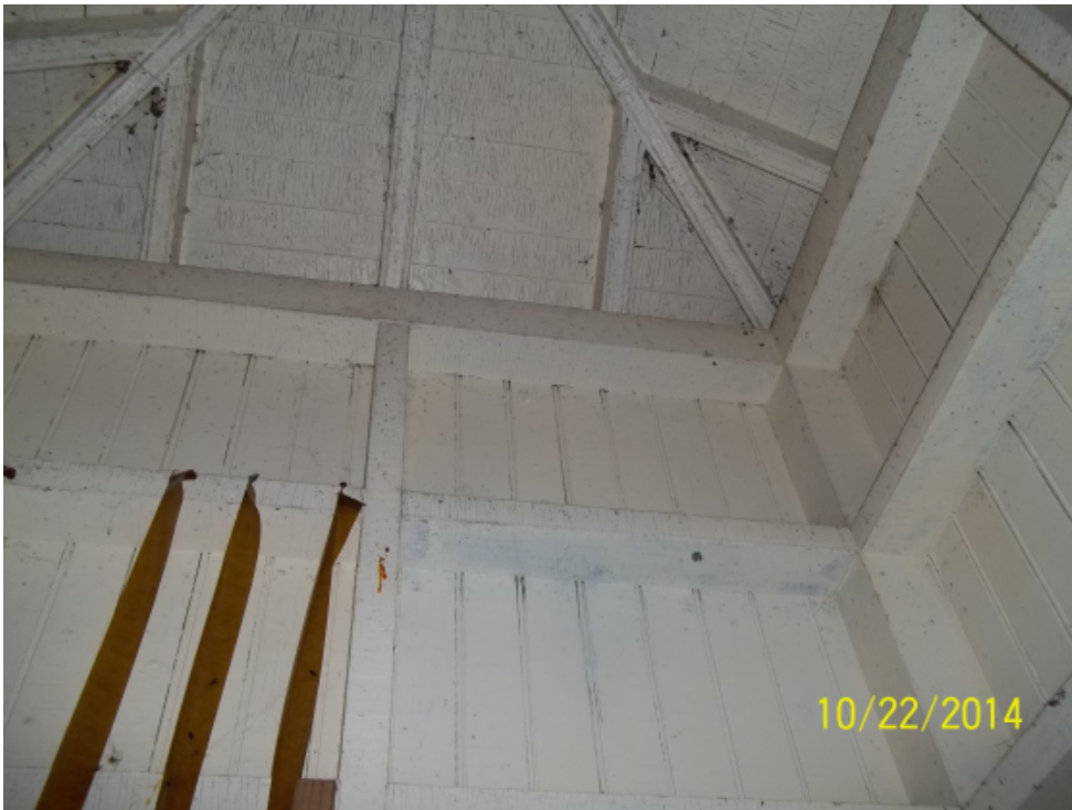
Photo 36: View looking inside at upper level of lighthouse.
