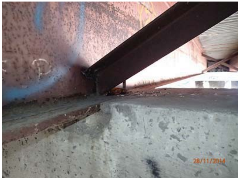
Photography 12: Some bracing "X" not welded properly
