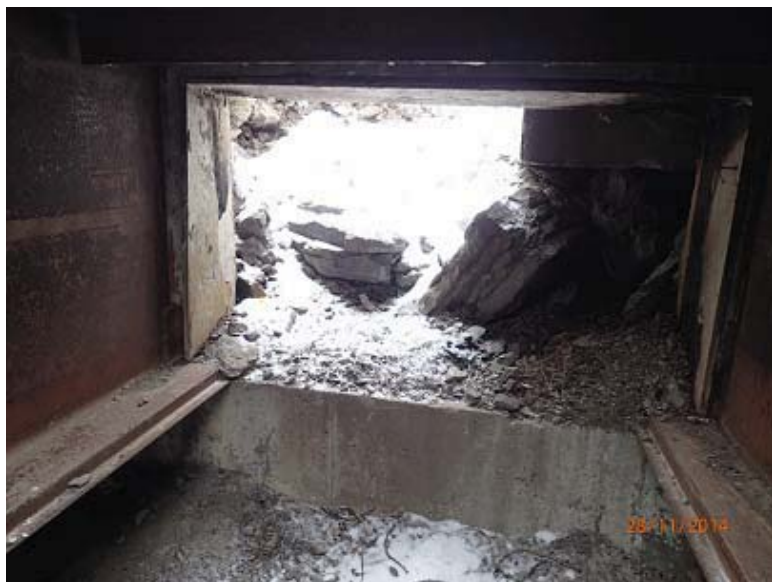
Photography 21: Concrete wall - 800mm aperture height to close
