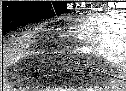
Remove waste grit from work areas as soon as possible.
