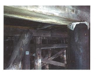
PHOTO C15-07 TIMBER PILED JETTY - TYPICAL VIEW UNDER WEST CRANE PAD
