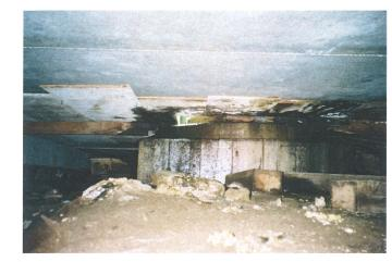
PHOTO C17-03 HIGH MAST LIGHT FOUNDATION UNDER STEEL PILED CONCRETE DECK - NOTE TIMBER FORMS LEFT IN PLACE
