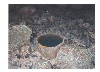
PHOTO C14-09 OPEN STEEL PIPE PILE UNDER STEEL PILED CONCRETE DECK - NOTE SAFETY RISK
