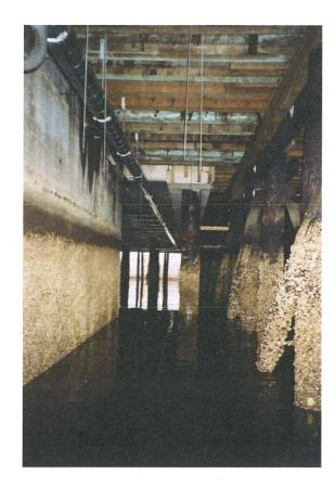
PHOTO C16-06 CONCRETE-FACED TIMBER CRIB NEXT TO TIMBER JETTY PILINGS
