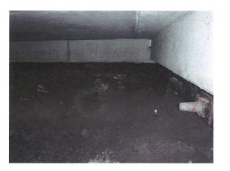
PHOTO C17-08 FORESHORE FILL MOUND UNDER STEEL PILED CONCRETE DECK - NOTE STEEL WALER AT RIGHT AND SEVERELY LIMITED HEADROOM
