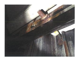
PHOTO C17-09 DETAIL VIEW OF STEEL WALER AND ANCHOR AT PAINTED SHEET PILED BULKHEAD WALL
