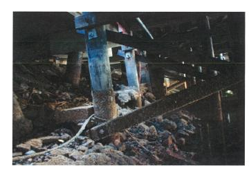
PHOTO C15-06 TIMBER PILED JETTY AT INTERFACE WITH STEEL PILED DECK- NOTE RIPRAP ON FORESHORE AND MISCELLANEOUS CONCRETE FOOTINGS
