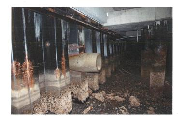
PHOTO C14-08 STORMWATER OUTFALL AT SHEET PILE BULKHEAD
