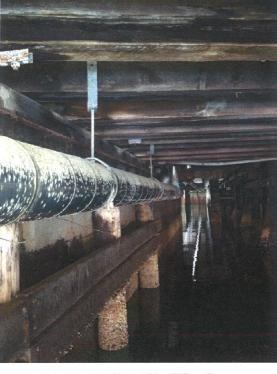
PHOTO C15-03 TIMBER PILED JETTY AT TIMBER CRIB LOOKING SOUTH - NOTE FENDERING AT FACE OF TIMBER CRIB
