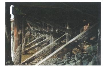
PHOTO C15-02 TIMBER PILED JETTY - TYPICAL VIEW AT EAST APPROACH JETTY LOOKING WEST
