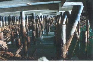
PHOTO C14-03 STEEL PILED CONCRETE DECK LOOKING EAST - NOTE BATTER PILES AND TIMBER PILE REMNANTS
