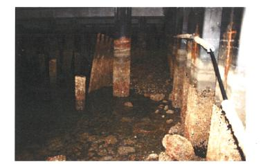
PHOTO C14-06 PAINTED SHEET PILE BULKHEAD - NOTE CATHODIC PROTECTION AND REMNANTS OF LOWER SHEET PILING (TIDE APPROX. EL+1.0M)
