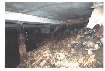
PHOTO C17-05 FORESHORE FILL MOUND UNDER STEEL PILED CRANE PAD - LOOKING NORTHWEST TOWARDS TIMBER CRIB
