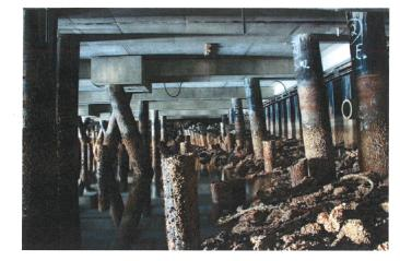
PHOTO C14-04 STEEL PILED CONCRETE DECK LOOKING WEST - NOTE CATHODIC PROTECTION CABLES AT SLAB SOFFIT
