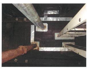
PHOTO C16-04 UNDER-PIER MECHANICAL AND ELECTRCIAL SERVICES AT TIMBER FIRE STOP WALL
