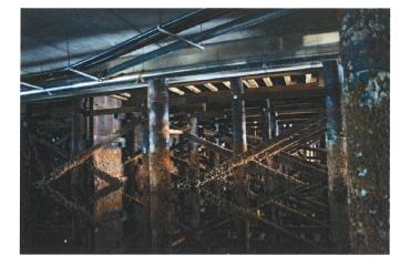
PHOTO C14-05 STEEL PILED CONCRETE DECK NEXT TO TIMBER PILED WEST JETTY - NOTE TIMBER FIRE STOP WALL AND CROSS-BRACING
