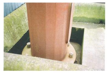
PHOTO C17-02 HIGH MAST LIGHT ABOVE STEEL PILED CONCRETE DECK - NOTE LIMITED SIZE OF DECK OPENING
