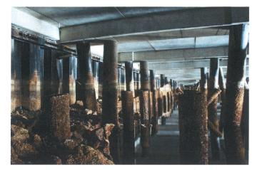
PHOTO C14-02 STEEL PILED CONCRETE DECK LOOKING EAST - NOTE TIMBER PILE REMNANTS AND LOWER SHEET PILING
