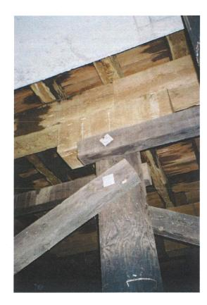
PHOTO C15-08 TIMBER INFILL DECK CONSTRUCTION - NOTE CONDITION OF TIMBER AT THIS STRUCTURE
