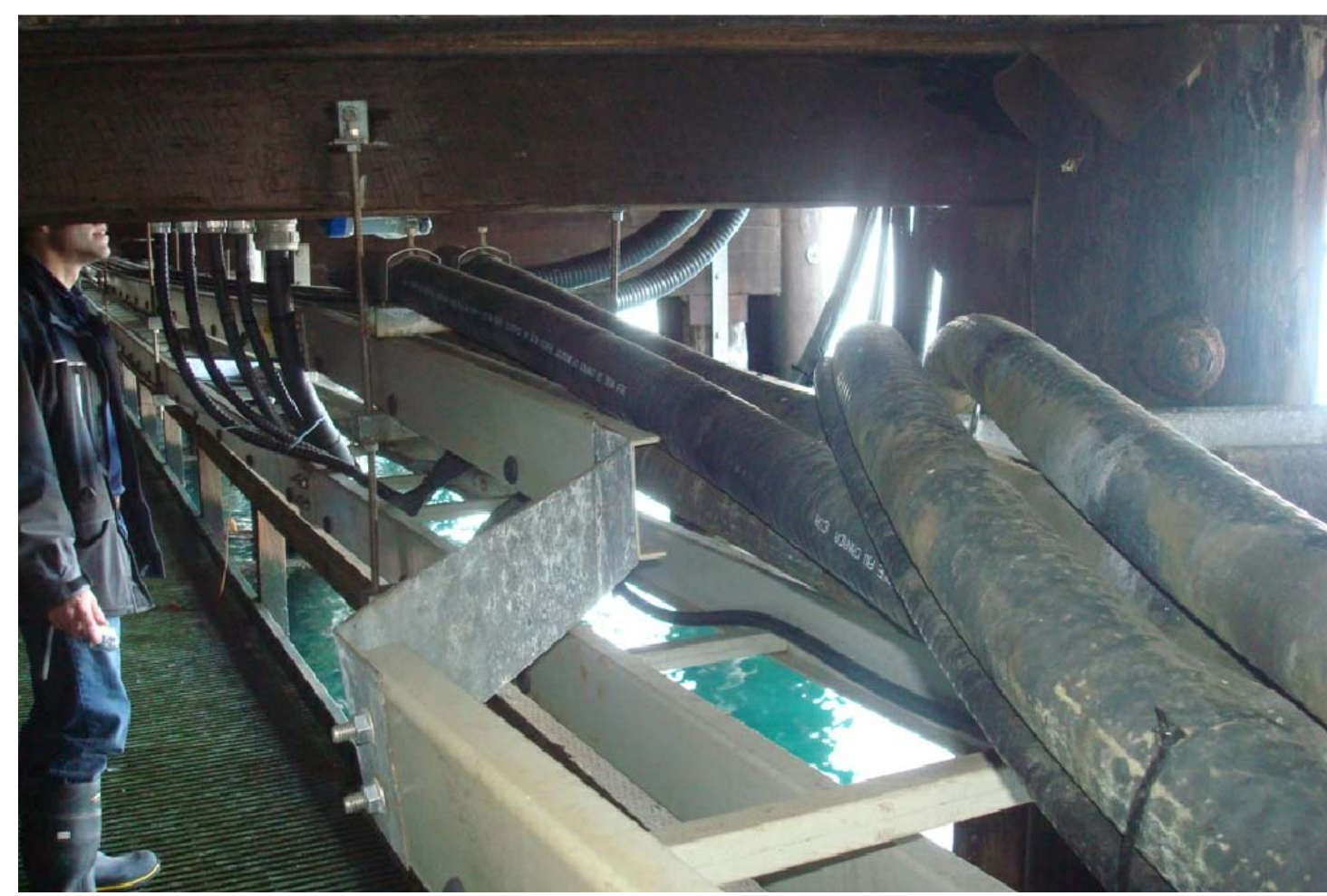
PHOTO C16-07 UNDER-PIER CATWALK AT KIOSK LOCATION - LOOKING EAST
