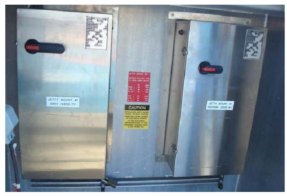
TYPICAL JETTY MOUNT KIOSK - POWER COMPARTMENT
