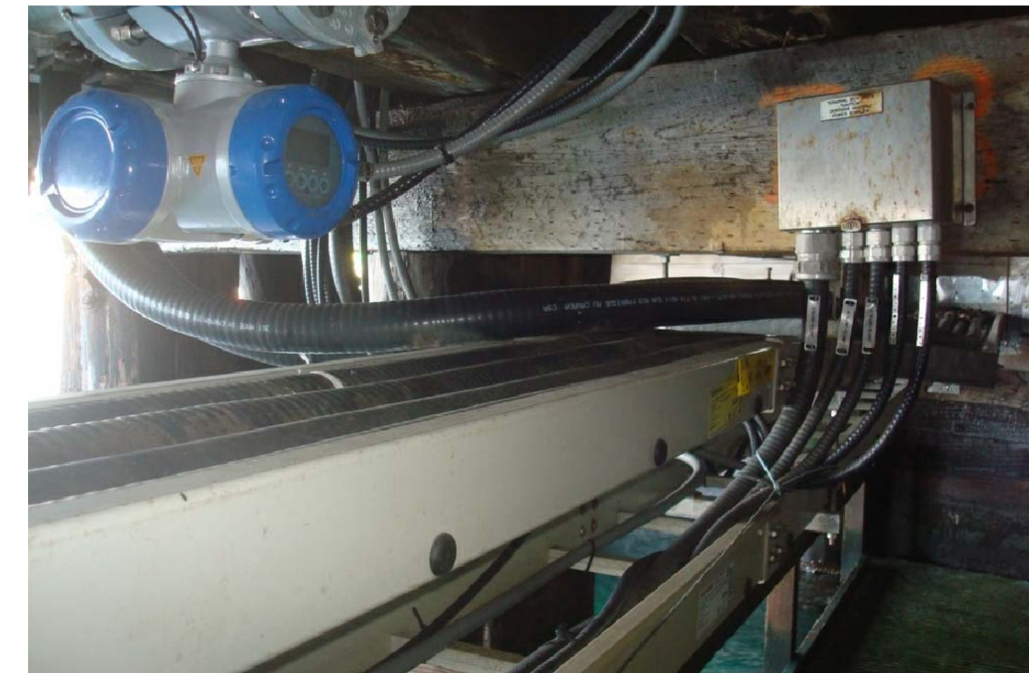
PHOTO C16-05 UNDER-PIER CATWALK AT KIOSK LOCATION - LOOKING WEST
