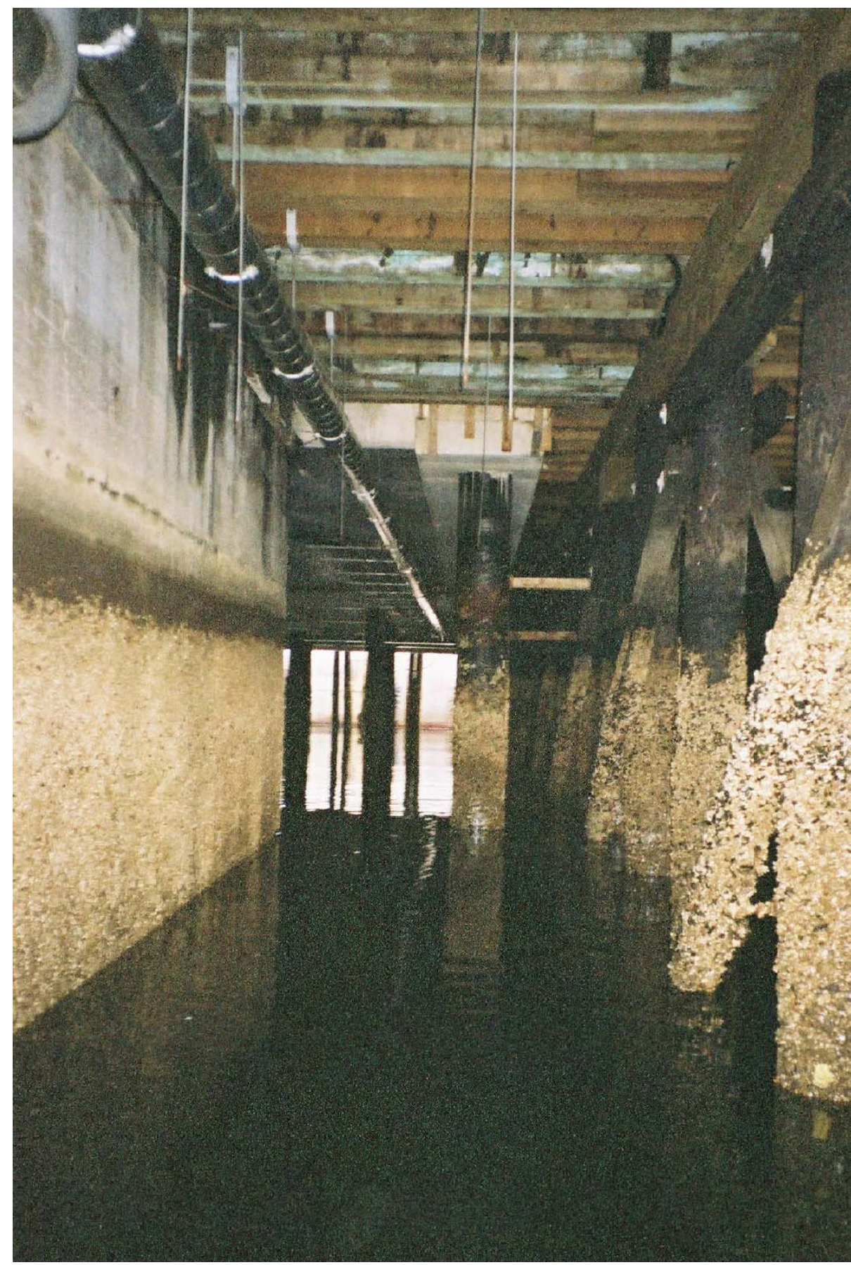
PHOTO C16-06 CONCRETE-FACED TIMBER CRIB NEXT TO TIMBER JETTY PILINGS
