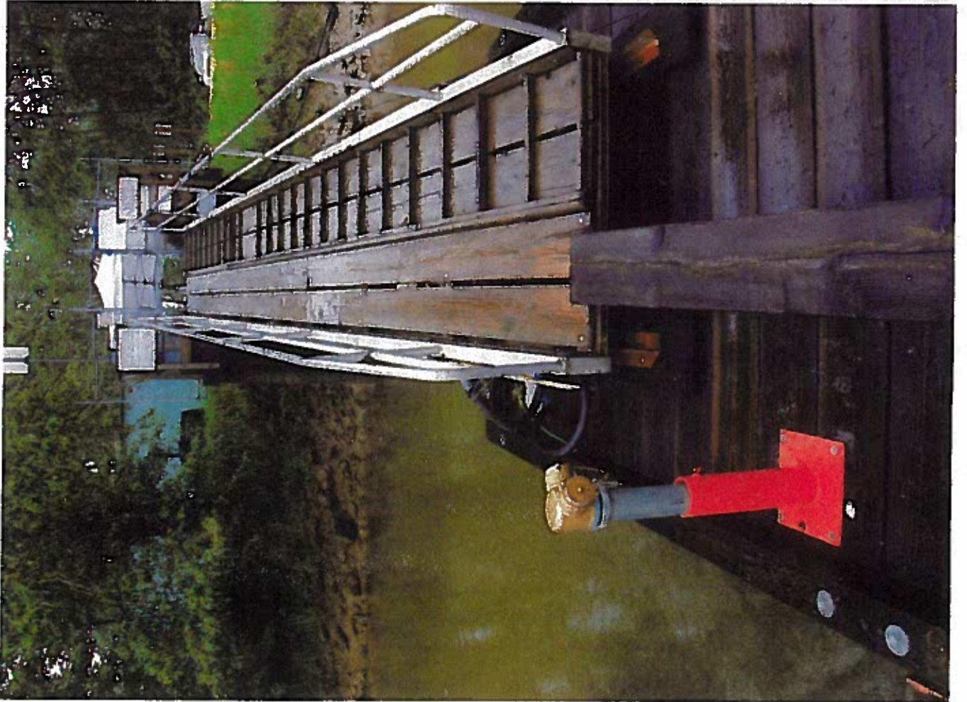
TYP STANDPIPE SUPPORTS
