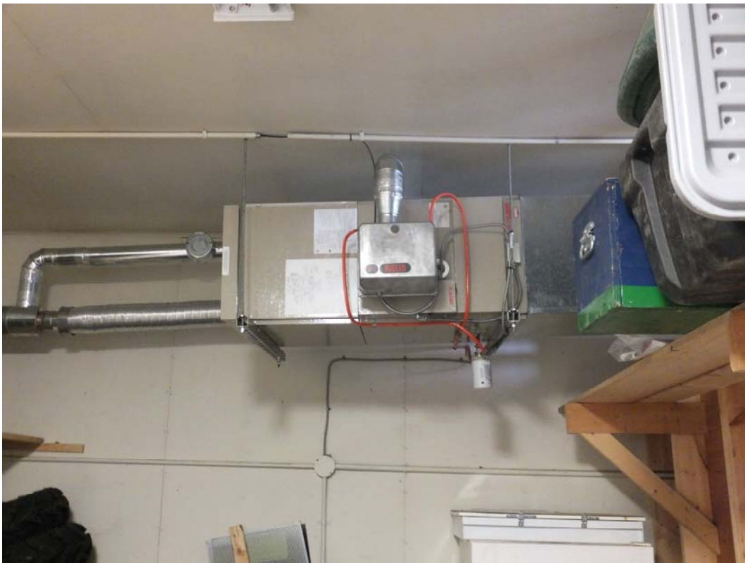
Photo 11: The oil fired ceiling mounted heater.
