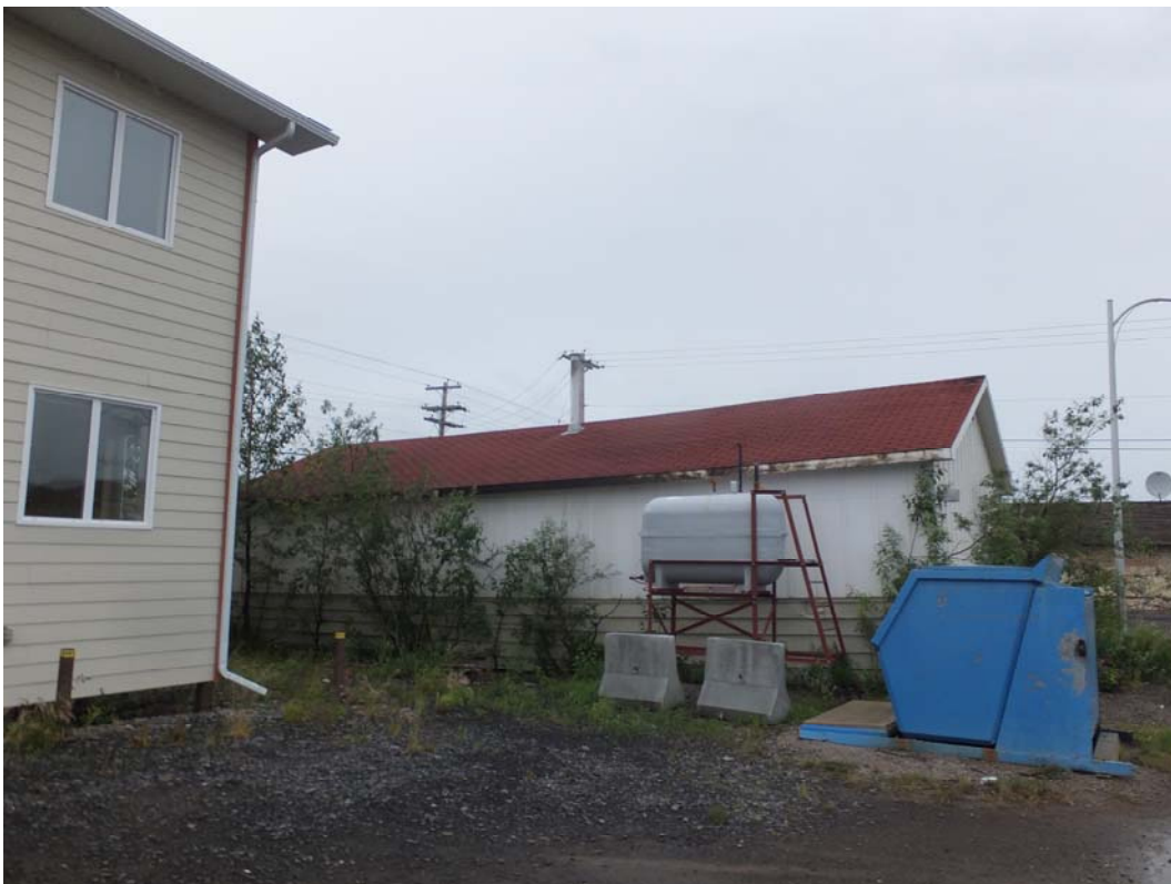
Photo 2: East side of the garage, note the above ground fuel storage tank and the chimney.
