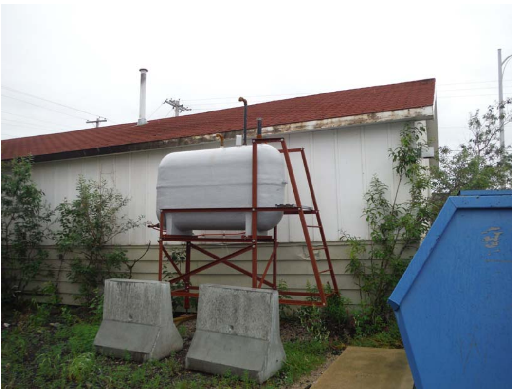
Photo 10: The above ground fuel storage tank located on the north side of the garage.
