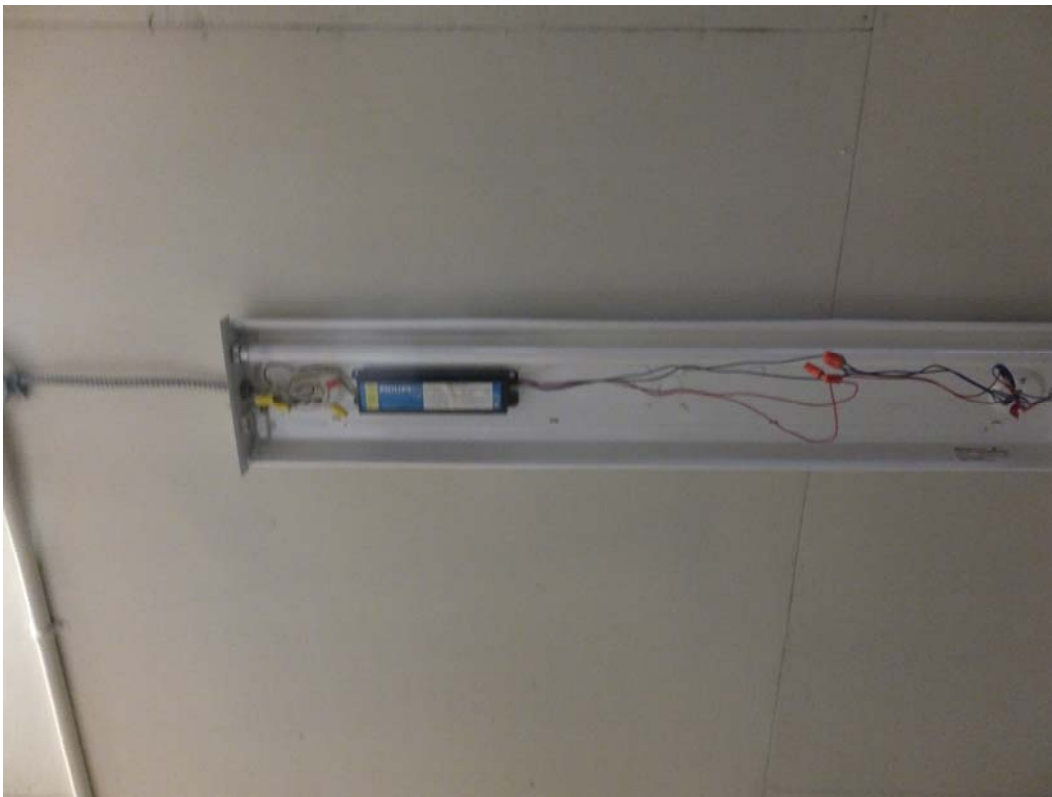
Photo 13: A typical T12 florescent light fixture, note that the ballast cover was removed prior to the inspection and that the ballast is a “NON-PCB” type.
