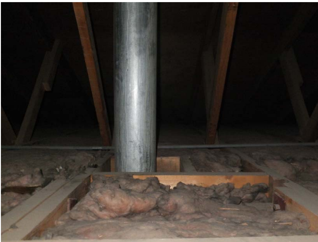
Photo 9: Attic space, looking east from access hatch. Note the wood frame construction, glass fiber batt insulation and the abandoned oil stove pipe/chimney.
