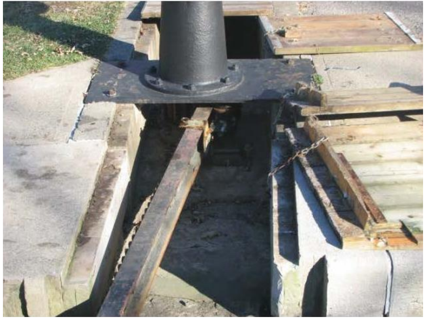
Photograph 8 - Rack and Pinion Pit (Right Bank)
