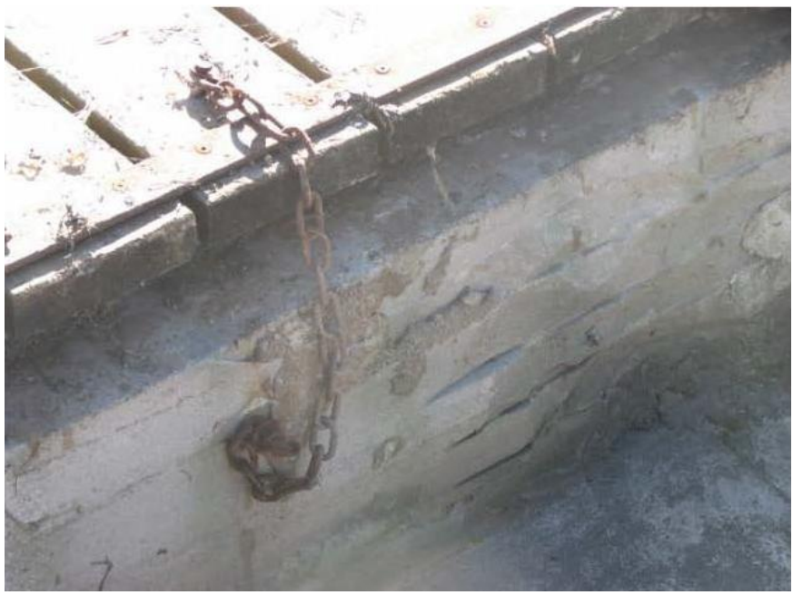
Photograph 9 - Decking Attach Chain
