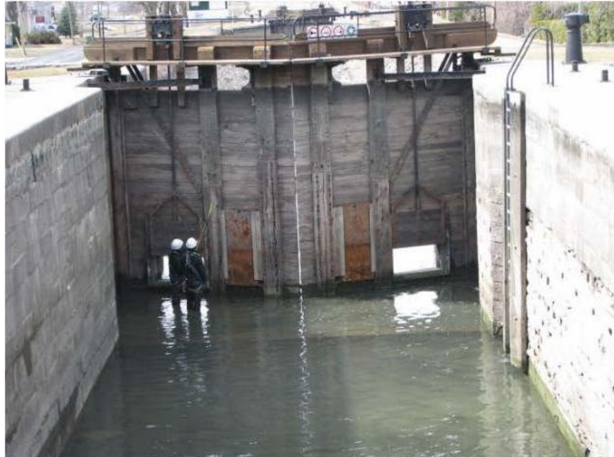
Photograph 1 - Upstream Face of the Gate
