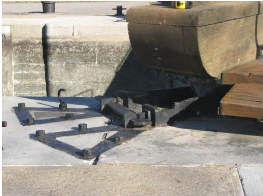
Photograph 7 - Strap Attach System (Left Bank)
