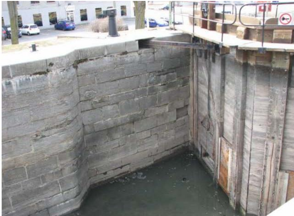
Photograph 4- Opening Mechanism - Left Gate
