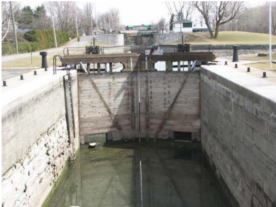
Photograph 5 - Downstream Face of the Gate
