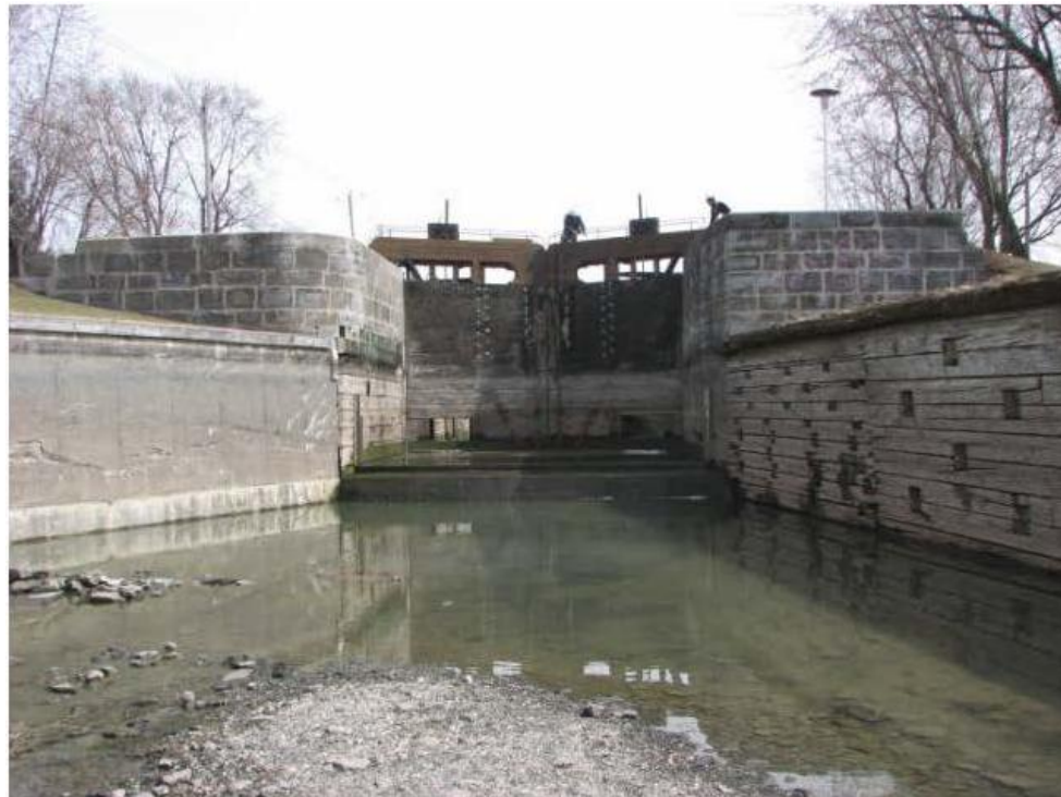
Photograph 2 - Downstream Face of the Gate
