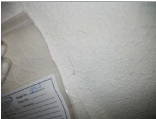
Non-asbestos texture finish on ceiling (samples 0005a-c), Main Level Living Room
