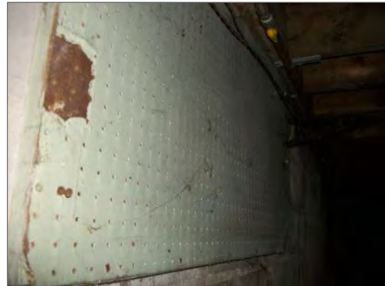
Non-asbestos wood fibre perforated board on wall, Crawlspace
