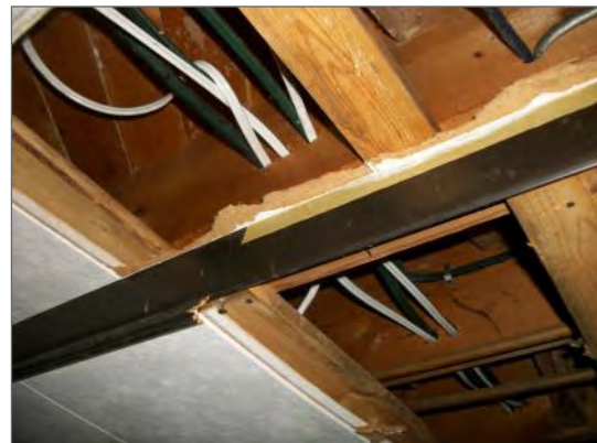
Non-asbestos 12" x 12" splined wood fibre ceiling tiles, Basement Rec Room
