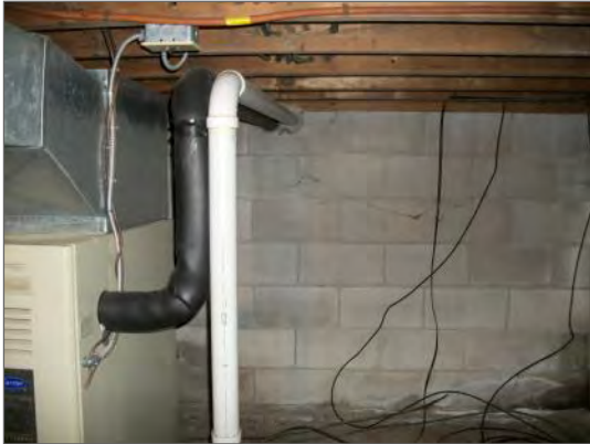
Non-asbestos Armaflex insulation on pipe serving the furnace, Crawlspace
