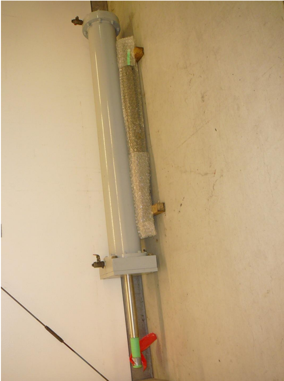
Existing Penstock Gate hydraulic cylinder with fittings shown for reference only.
