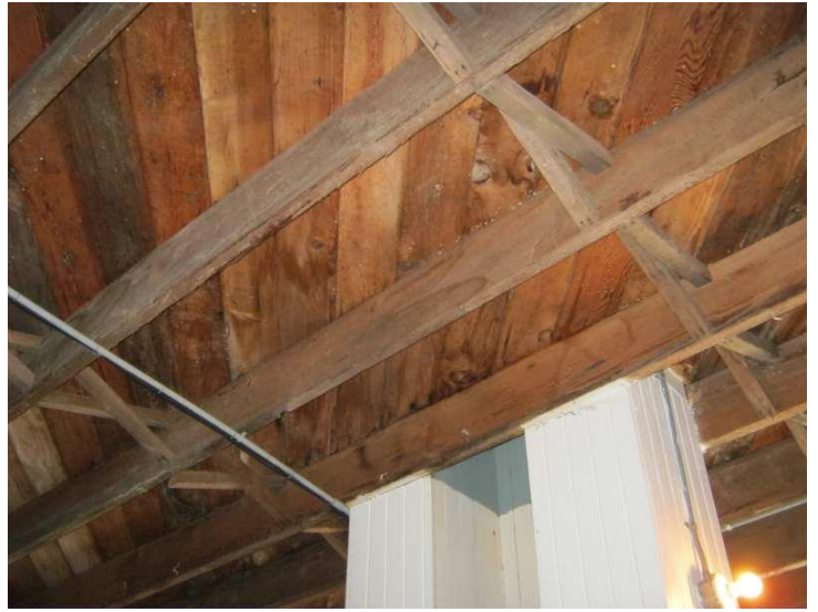
#38 - 2nd Floor Framing
