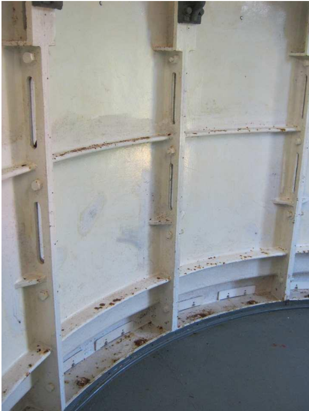
#57 - Lantern Room Interior Wall Assembly
