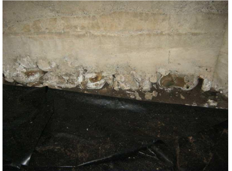
#10 - Foundation Soil Bearing Condition
