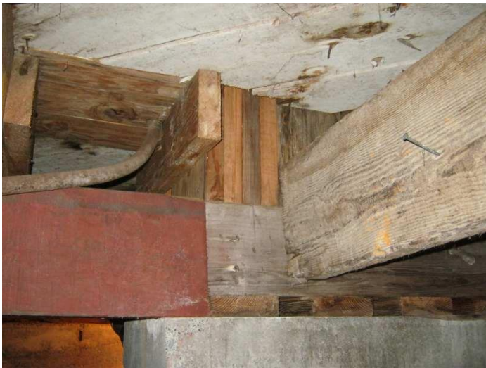
#33 - Interior Wood Column at Base Northeast - Repaired
