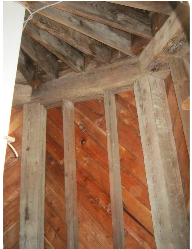
#48 - 3rd Floor Wall Framing
