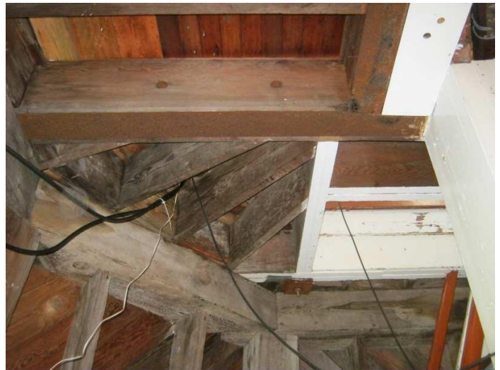
#54 - 4th Floor Framing
