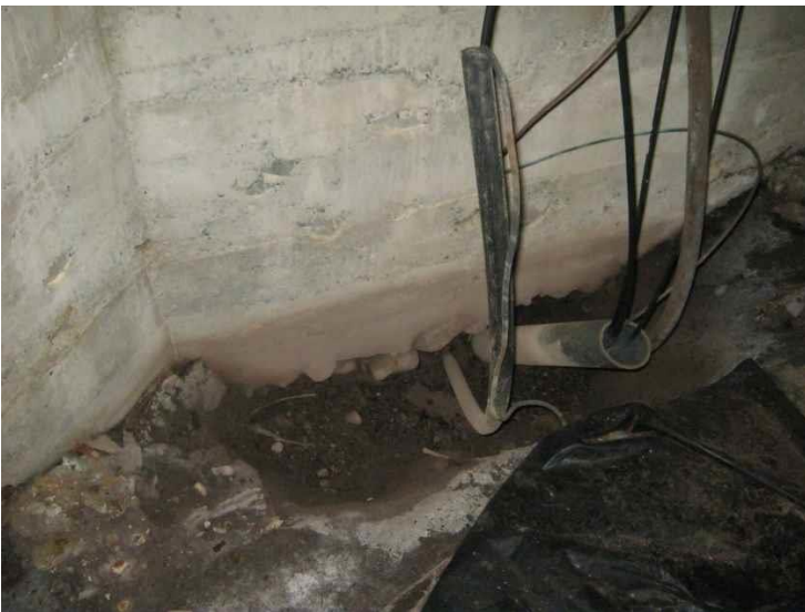
#73 - Foundation Soil Bearing Condition
