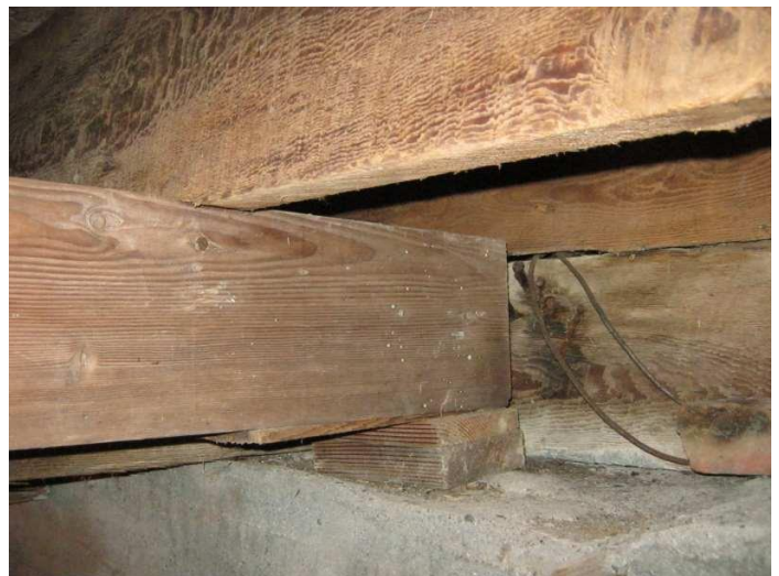
#24 - Main Floor Beam Replaced - Northwest
