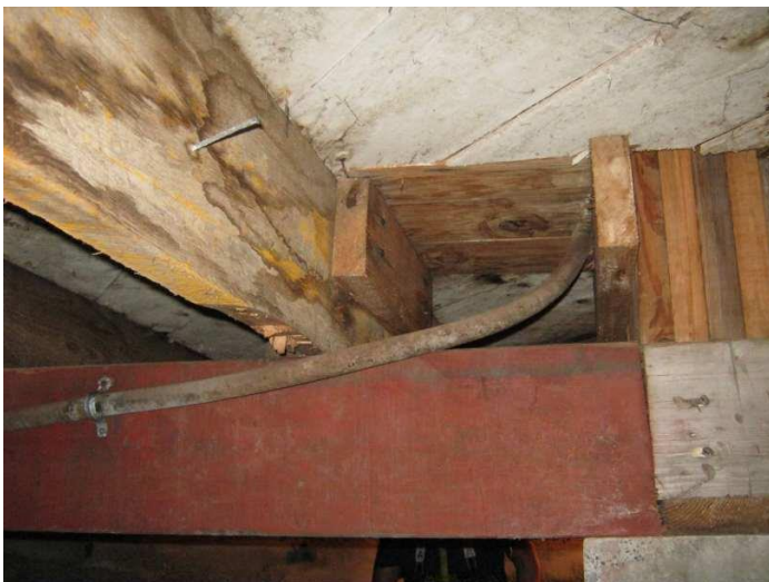
#23 - Main Floor Beam Replaced – Northeast
