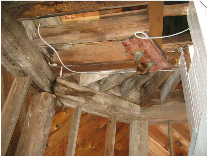
#51 - 4th Floor Framing
