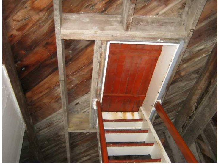
#46 - 3rd Floor Framing
