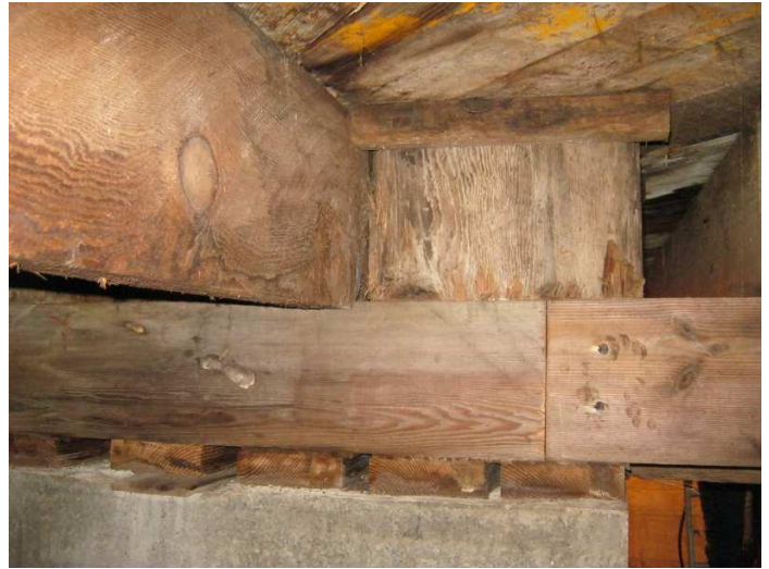
#32 - Interior Wood Column at Base Northwest - Repaired
