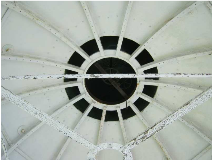
#59 - Lantern Room Roof Framing
