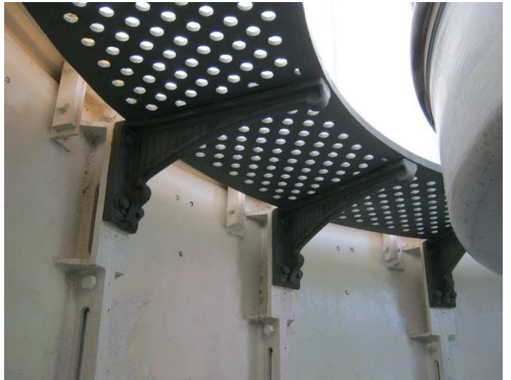
#58 - Lantern Room Interior Platform
