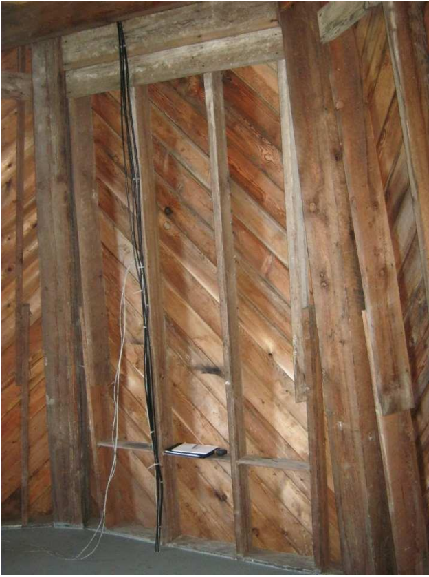
#41 - 2nd Floor Wall Framing
