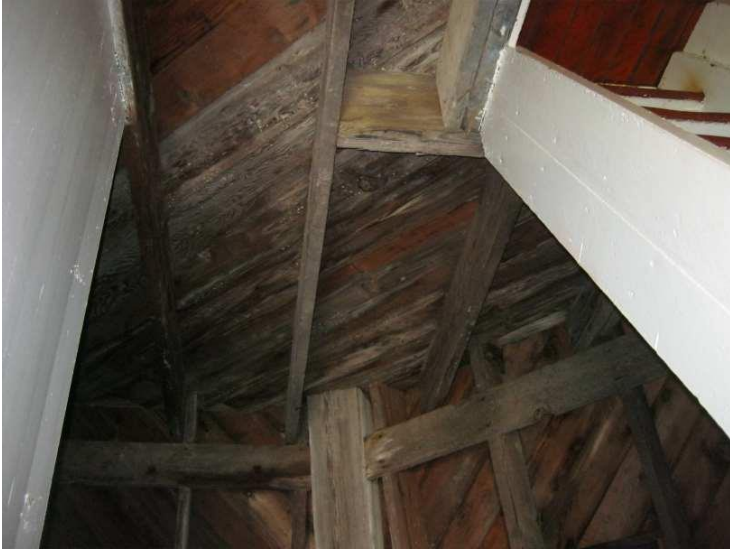
#45 - 3rd Floor Framing
