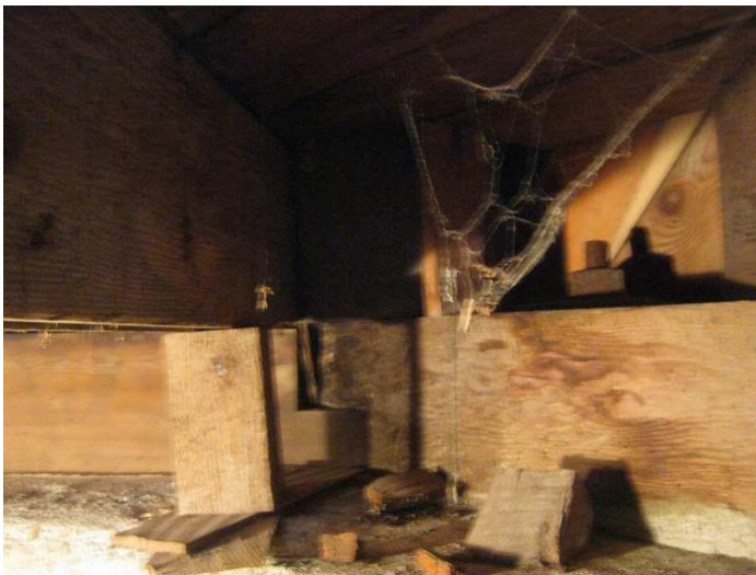
#29 - South Wall Plate Replaced - West End
