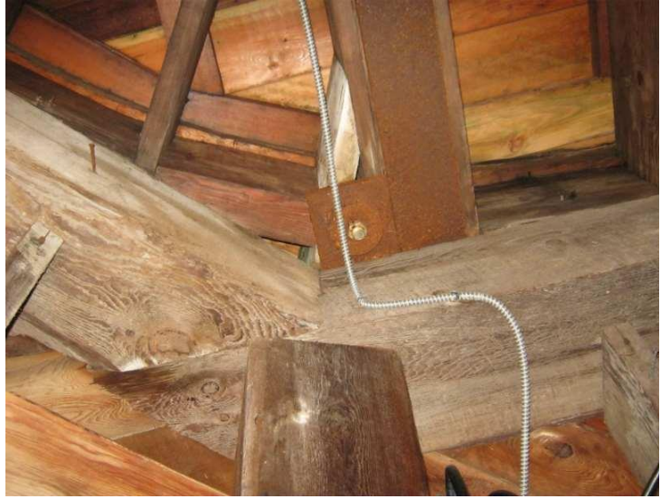
#56 - Lantern Room Anchor to 4th Floor
