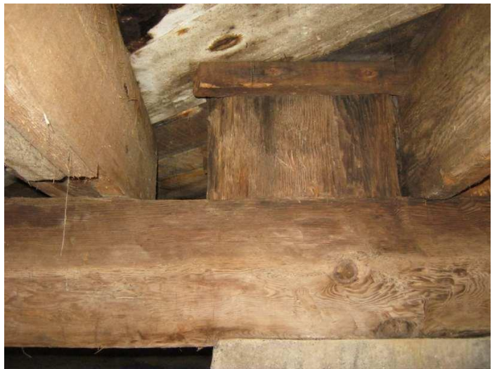
#30 - Interior Wood Column at Base Southwest - Original Construction
