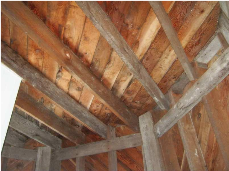
#43 - 3rd Floor Framing
