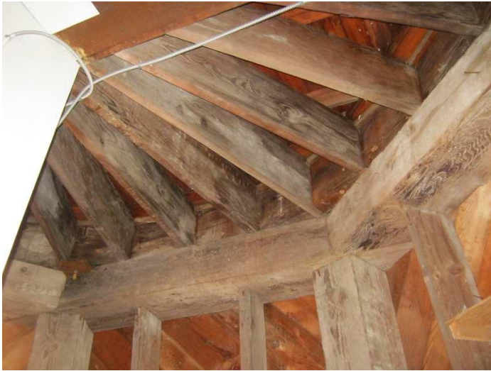
#49 - 4th Floor Framing
