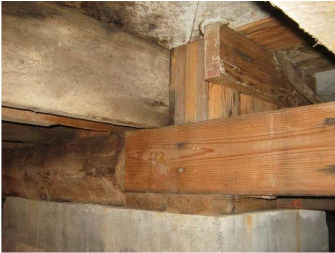
#31 - Interior Wood Column at Base Southeast - Repaired
