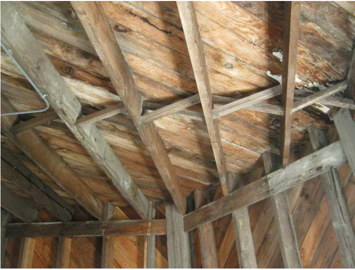
#37 - 2nd Floor Framing
