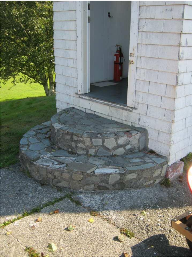
#9 - Exterior Entrance Stair
