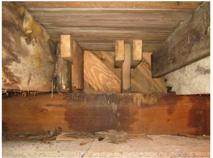
#28 - South Wall Plate Replaced - Centre
