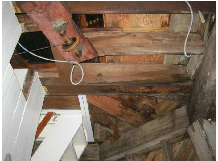
#52 - 4th Floor Framing
