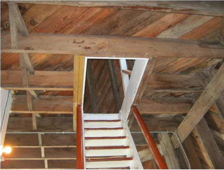
#39 - 2nd Floor Framing
