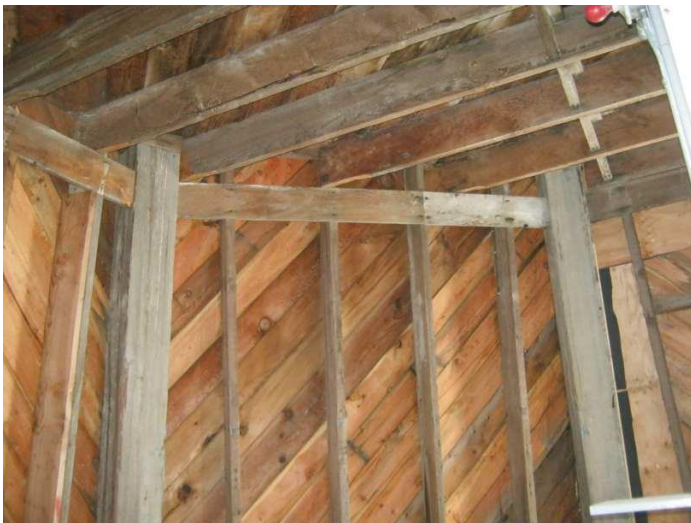
#35 - Main Floor Typical Wall Framing
