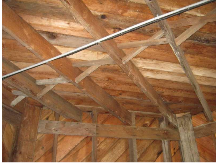
#40 - 2nd Floor Framing
