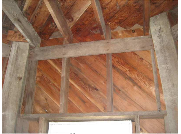
#42 - 2 nd Floor Wall Framing
