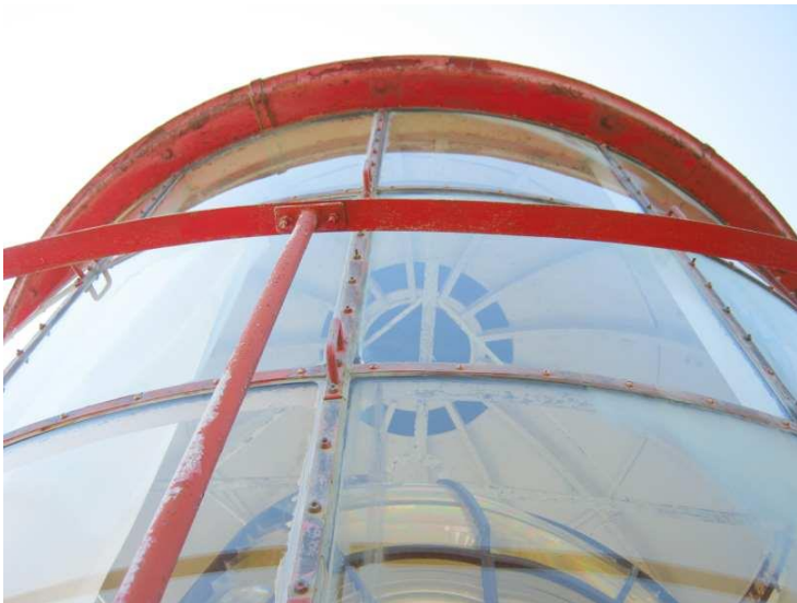
#65 - Lantern Room Window - Exterior
