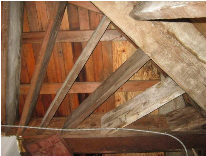
#53 - 4th Floor Framing
