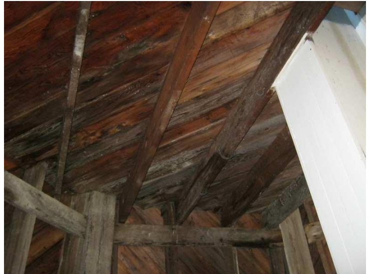
#44 - 3rd Floor Framing
