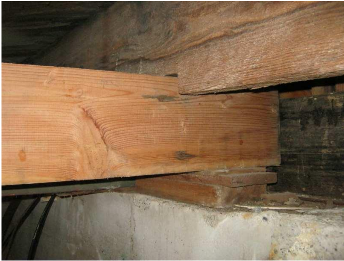
#25 - Main Floor Beam Replaced - Southeast
