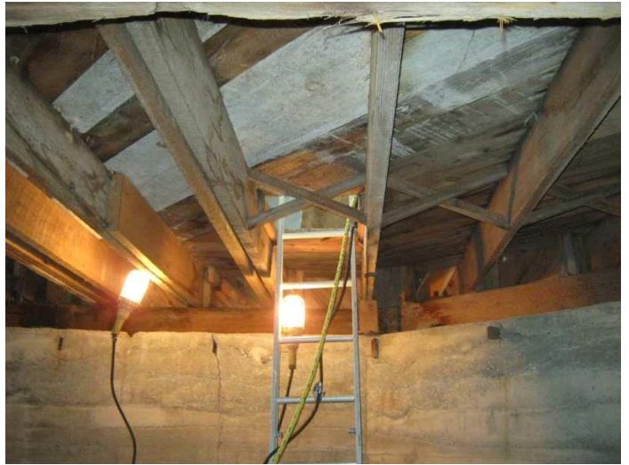
#26 - Main Floor Joist Repair - South
