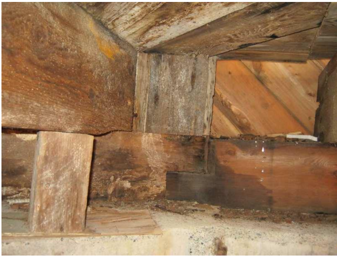
#27 - South Wall Plate Replaced - East End
