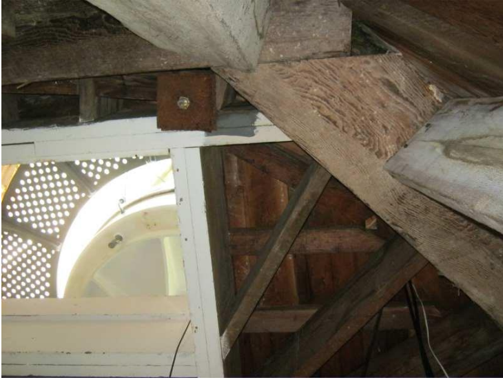
#55 - Lantern Room Anchor to 4th Floor
