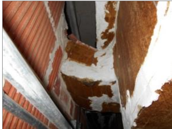
Photo 1, Asbestos containing parging cement on seams of the tar paper and fiberglass insulation on ducts throughout the main floor corridor.
