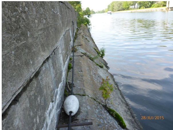
PHOTO 03 - Typical existing repairs
