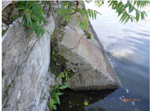
Photo 02- Typical existing repairs
