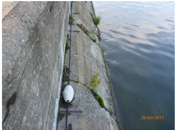
Photo 04 - Typical existing repairs
