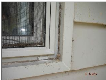
White window caulking present on exterior windows
