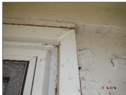
White window caulking present on exterior windows
