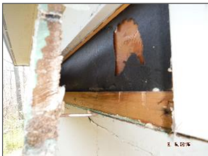
Tar paper present on the inside surfaces of building walls
