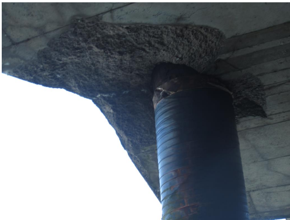
Figure 3-Large concrete spall from pile cap at BD1-I4
