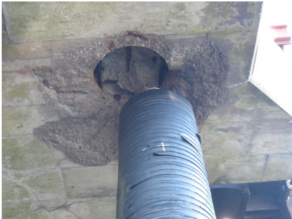
Figure 2-Pile dislodged from pile cap at BD3-K4.
