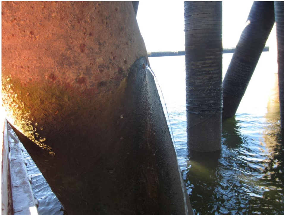
Figure 5-Hole in pile at Elev. +3.5m at pile WD1-L21.
