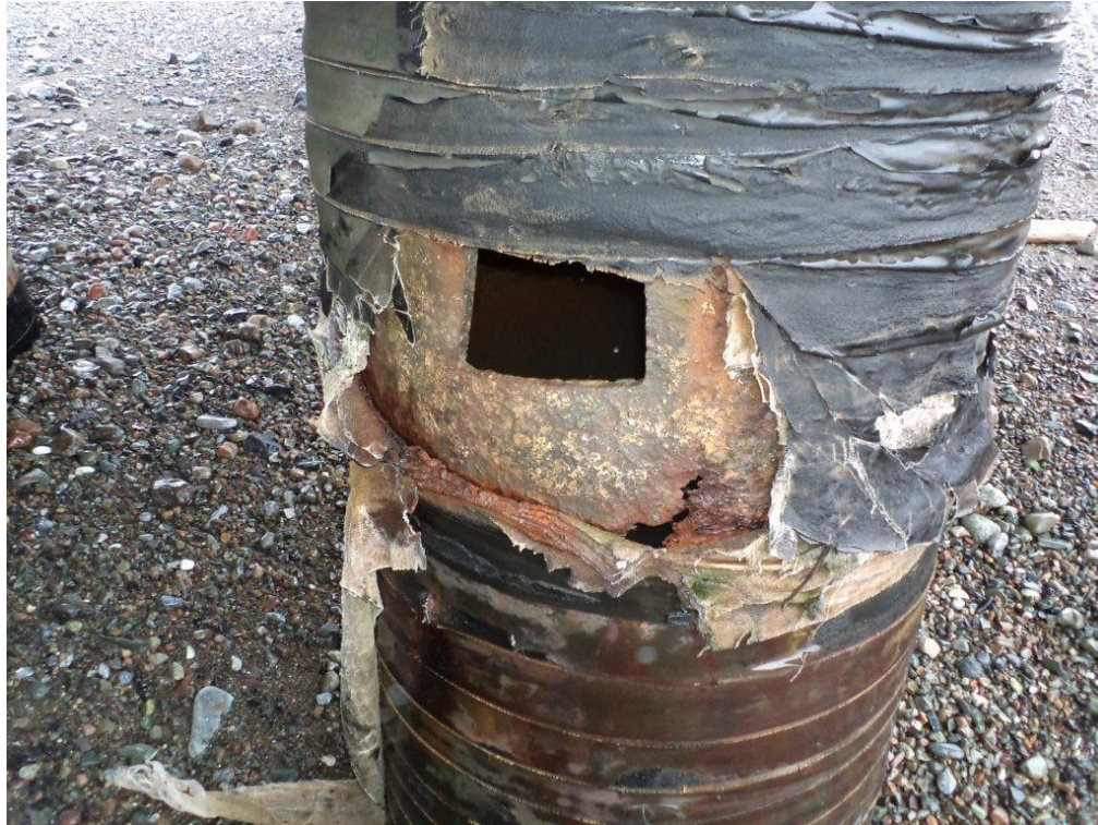
Figure 1-Coupon cut out of Pile Bent #2-Pile C10.
