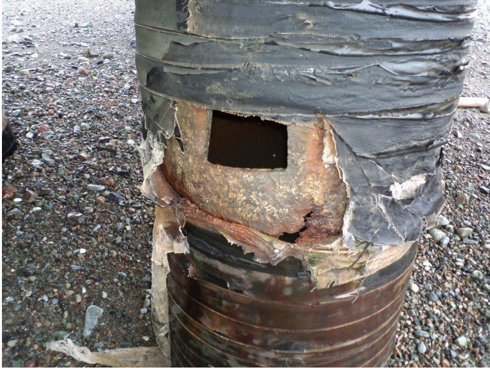
Figure 1-Coupon cut out of Pile Bent #2-Pile C10.
