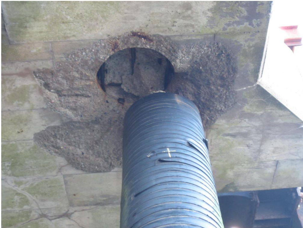
Figure 2-Pile dislodged from pile cap at BD3-K4.
