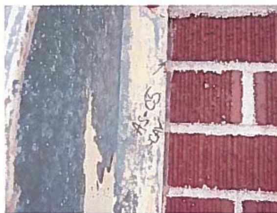
Photo 6: Photo of sample AS-05-CAV, caulking around heat shield.
