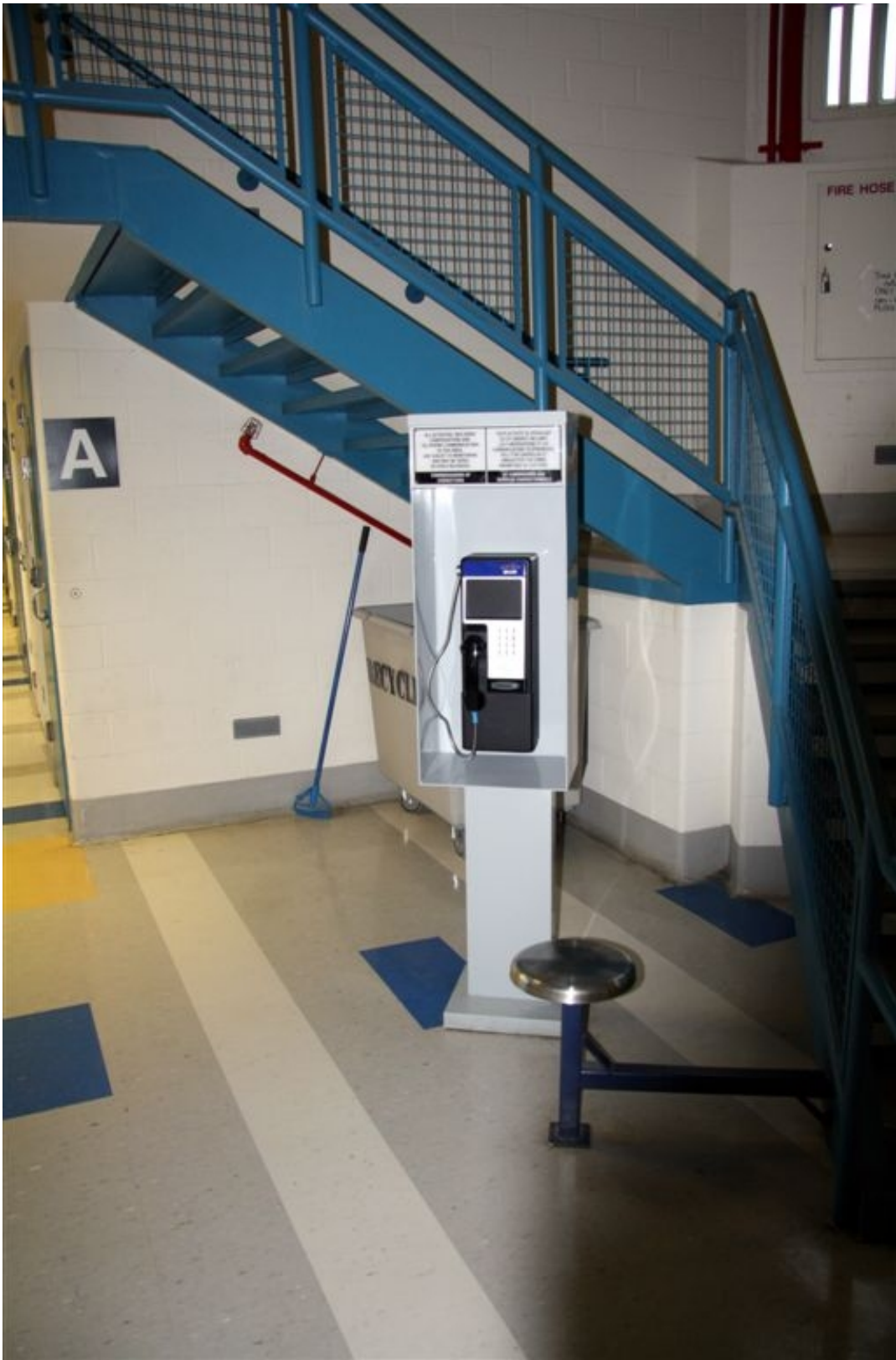
Figure 2 - Example of a Free-Standing Enclosure
