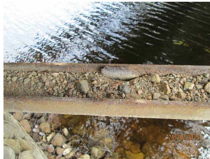
PHOTO #1 - CORRODED SWAY BRACE
