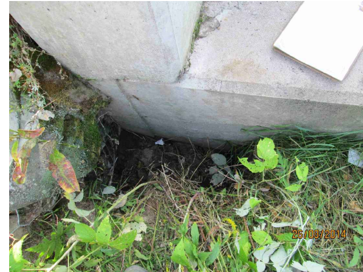
PHOTO #1 - EROSION ADJACENT TO ABUTMENT
