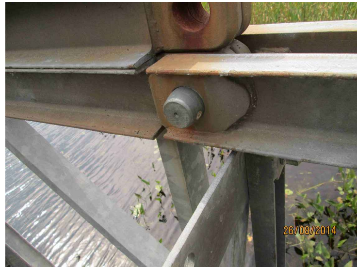
PHOTO #1 - MISSING COTTER PIN
