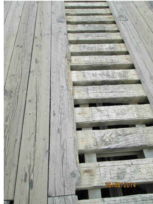
PHOTO #1 - DAMAGED RUNNING BOARDS
