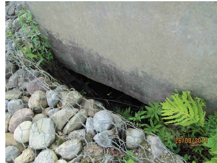
PHOTO #1 - ABUTMENT UNDERMINING
