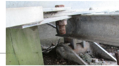
SWAY BRACE BOLTED CONNECTION
