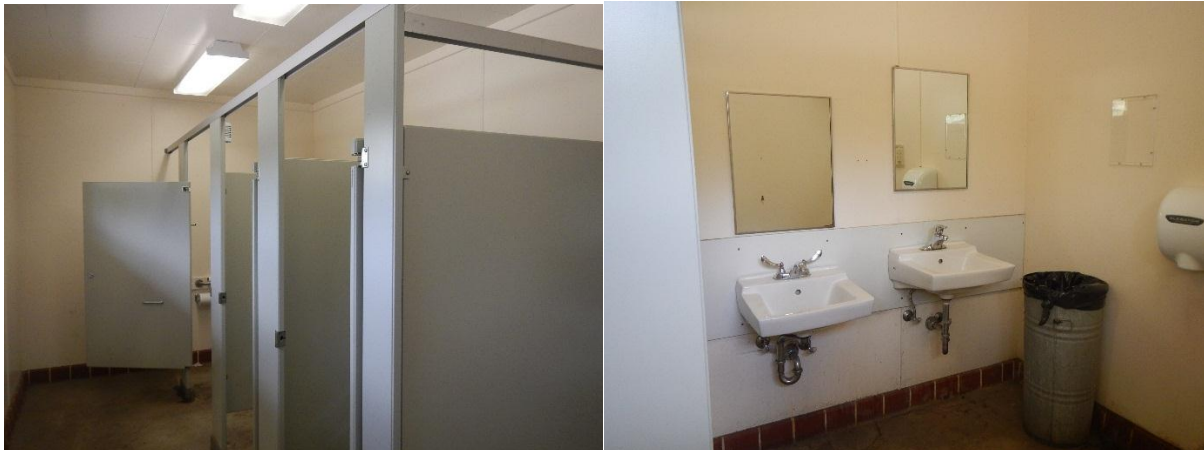
Existing washroom interior – Minnewanka DUA
