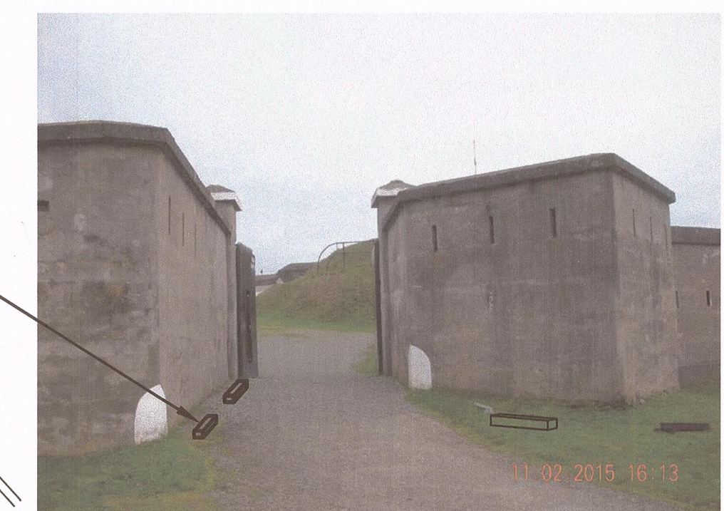
PHOTO #4 - GUARD HOUSE ENTRANCE
