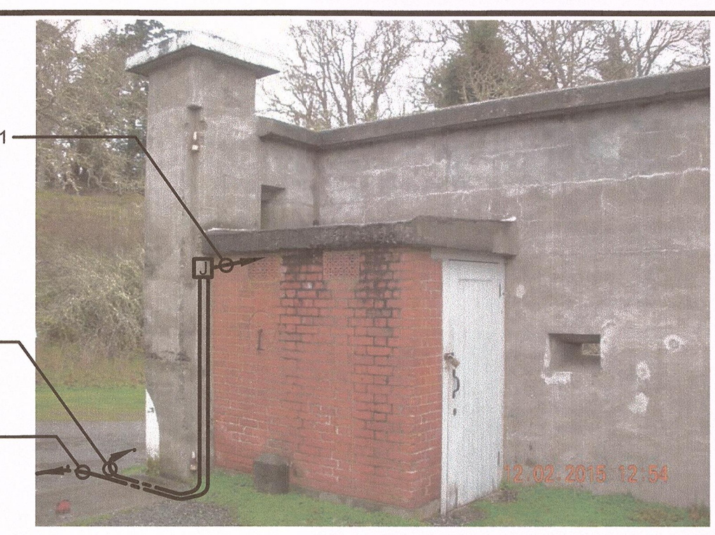
PHOTO #1 CASEMENT BARRACKS ELECT. RM.
