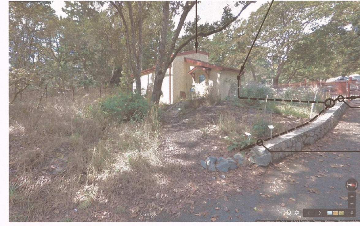
PHOTO #4 - ENTRY KIOSK BUILDING
