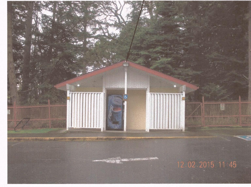
PHOTO #2 - WASHROOM BUILDING
