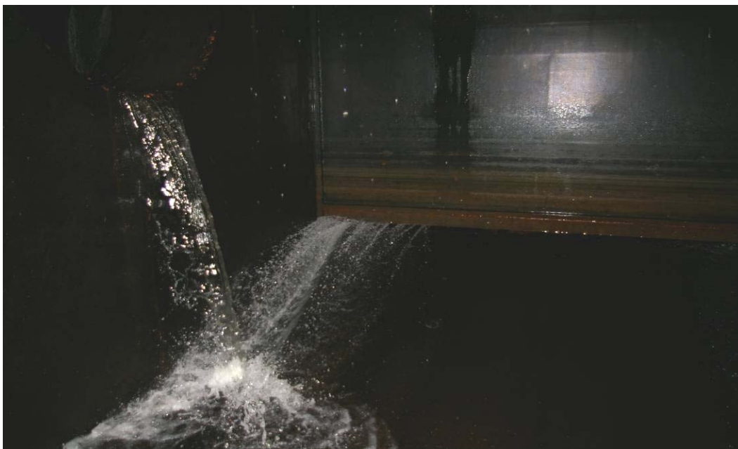
Photo 3 (August 15, 2007) Regulating Tunnel – Leakage beneath right side of Main Service Gate. Flow on left side of photo is leakage past the 1500 mm diameter Low Level Intake Gate.
