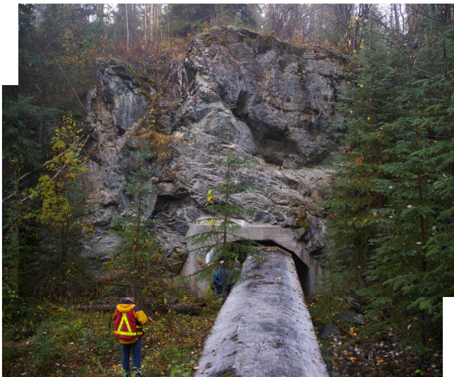
Photo 12 (October 10, 2007) West Supply Tunnel portal at Beaver Creek – No change noted since previous inspection; slope should be checked scaled.
