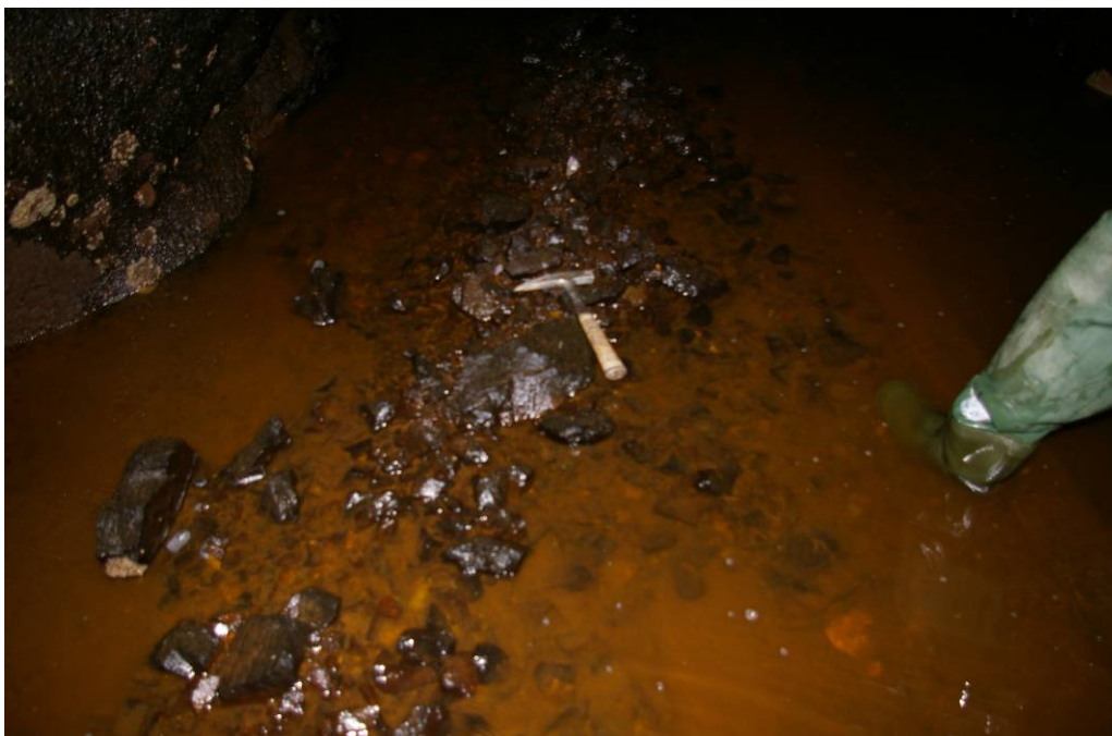
Photo 7 (August 15, 2007) West Supply Tunnel – Localized “wind-row” of rocks just downstream of small refuge bay on left side of tunnel (compare with Photo 2 of EBA December, 2002 report - no change noted in 2007).
