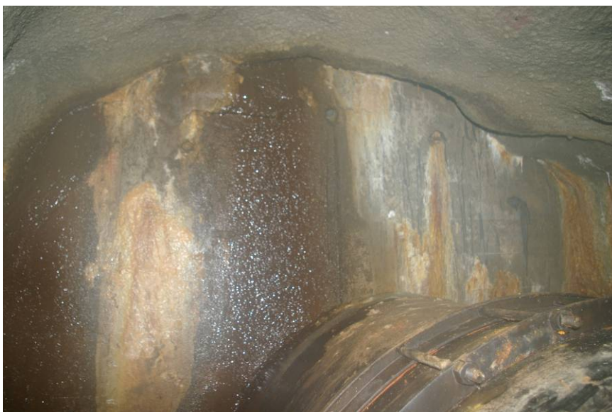
Photo 13 (October 9, 2007) East Supply Tunnel, Beaver Creek Bulkhead (Looking downstream) - The seepage rate (approximately 0.35 l/min by visual estimate) from crown of bulkhead on left side with tunnel “watered-up” should be monitored regularly for evidence of deterioration.
