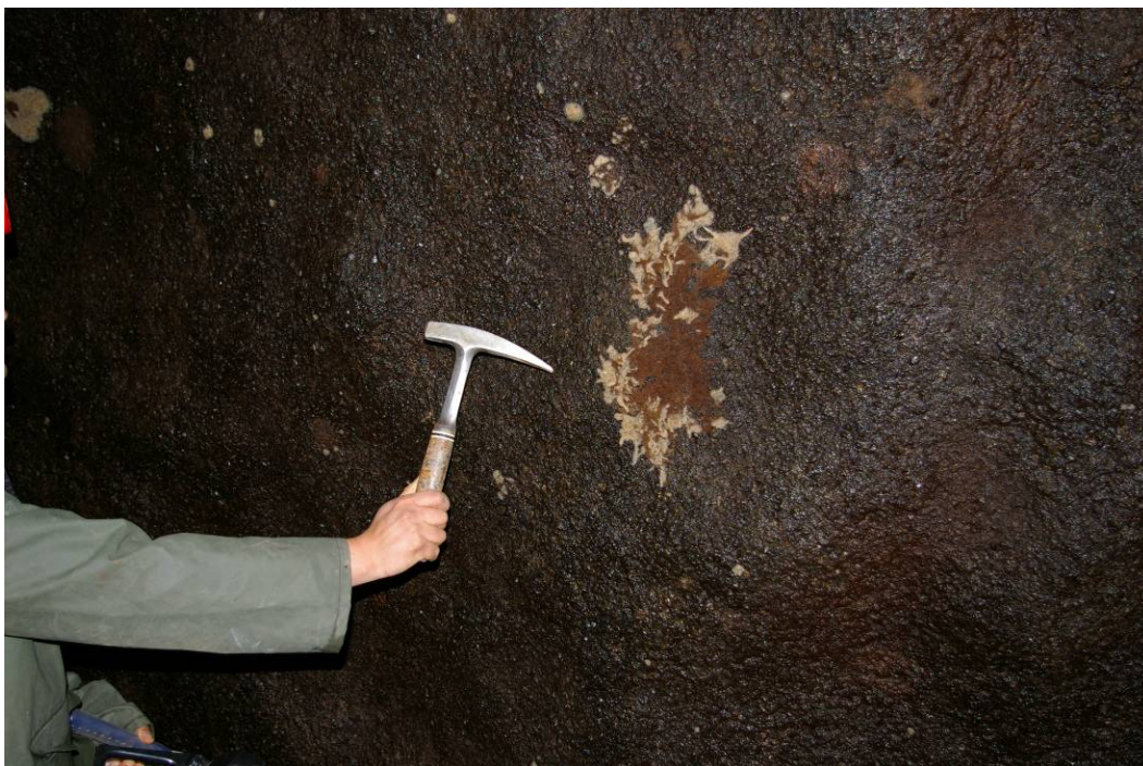
Photo 8 (August 15, 2007) West Supply Tunnel – Typical biological growth (possibly freshwater sponge) on shotcreted tunnel wall.
