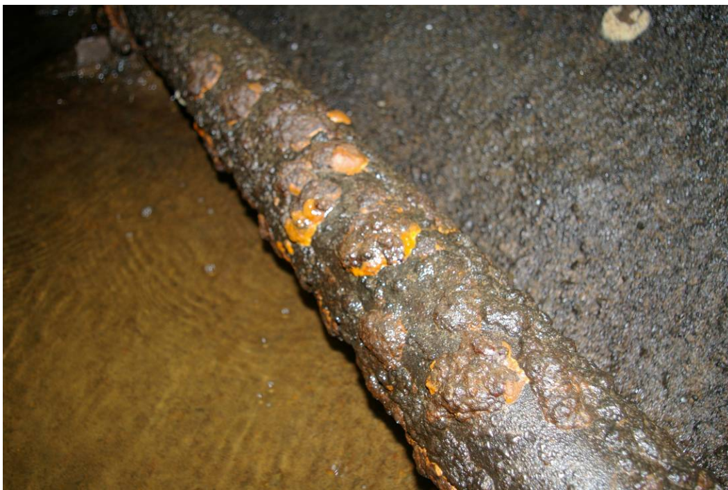
Photo 20 (August 15, 2007) East Supply Tunnel – Typical corrosion blisters on drain pipe.
