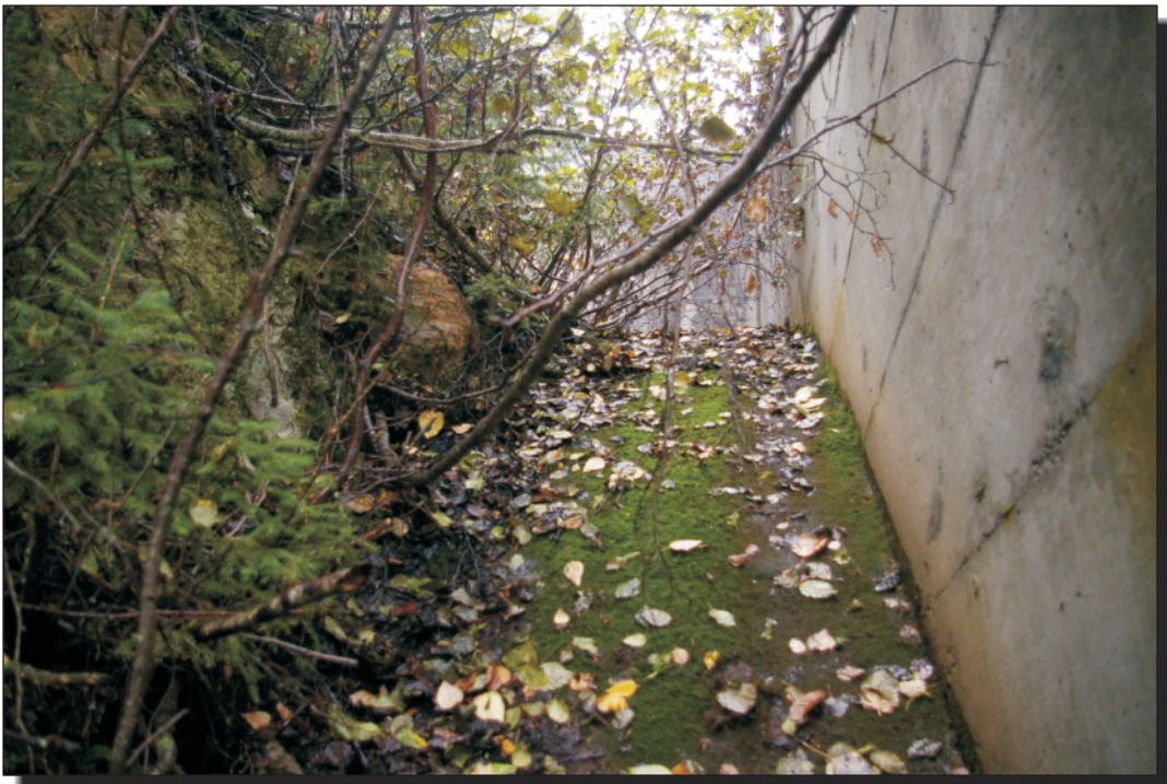
Photo 19 Right abutment between spillway wingwall and rock abutment.
