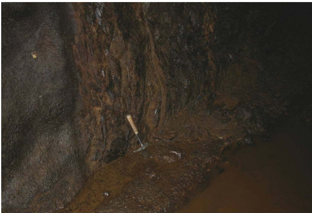
Photo 6 (August 15, 2007) West Supply Tunnel – Minor ( \leq 150 mm) rockfall on tunnel invert below unlined tunnel section (shotcrete visible on left).
