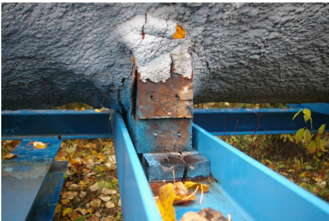
Photo 23 (October 9, 2007) Pipeline Trestle – Typical wood wedges used to support the supply pipeline on trestle show only relatively minor decay.
