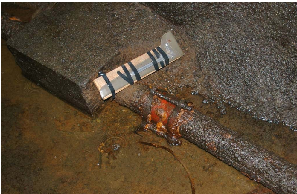
Photo 19 (August 15, 2007) East Supply Tunnel – Pipe clamp at drain pipe measurement Location #2.
