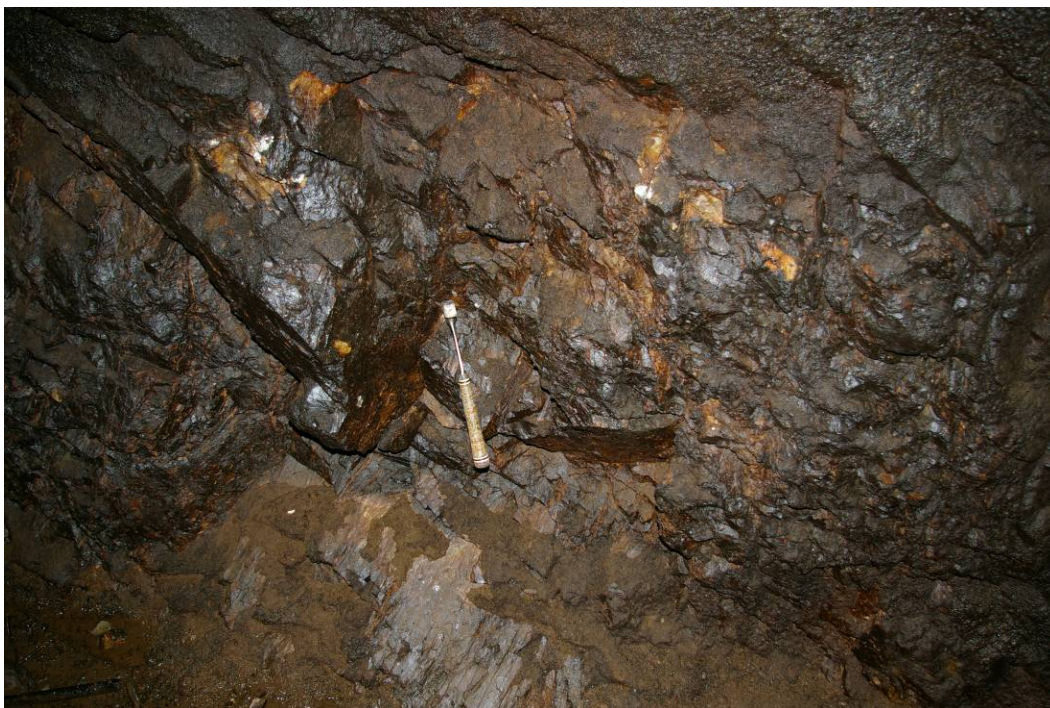
Photo 4 (August 15, 2007) West Supply Tunnel – Typical areas of loosened “drummy” rock on lower wall of tunnel (below shotcrete lining).
