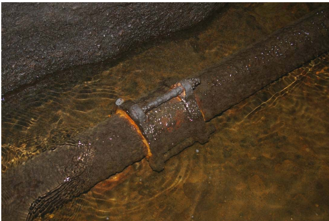
Photo 16 (August 15, 2007) East Supply Tunnel – Typical condition of clamp connections on drain pipe.
