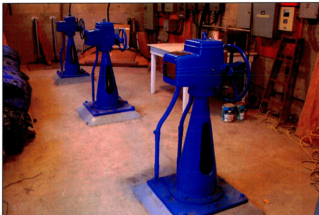
Figure 2: Regulating works hollow-cone valve actuators.
