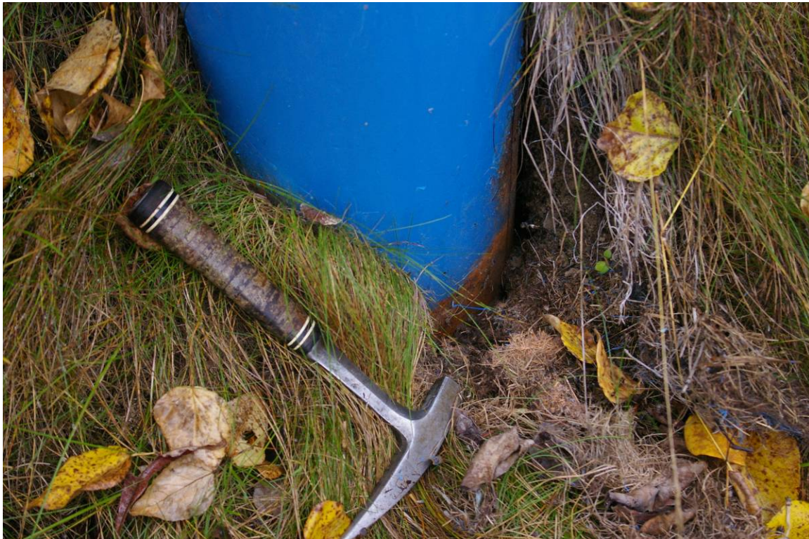
Photo 24 (October 9, 2007) Pipeline Trestle – Minor separation of soil noted adjacent to two piles does not appear to be recent.
