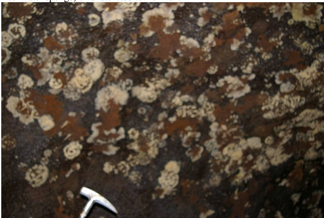
Photo 8 (August 15, 2007) West Supply Tunnel – Typical biological growth (possibly freshwater sponge) on shotcreted tunnel wall.
