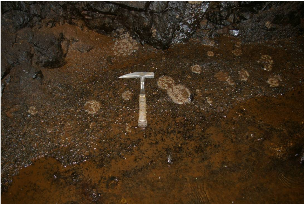
Photo 10 (August 15, 2007) West Supply Tunnel – Localized areas of biological growth (possibly freshwater sponge) on tunnel invert that were not noted during previous inspections.
