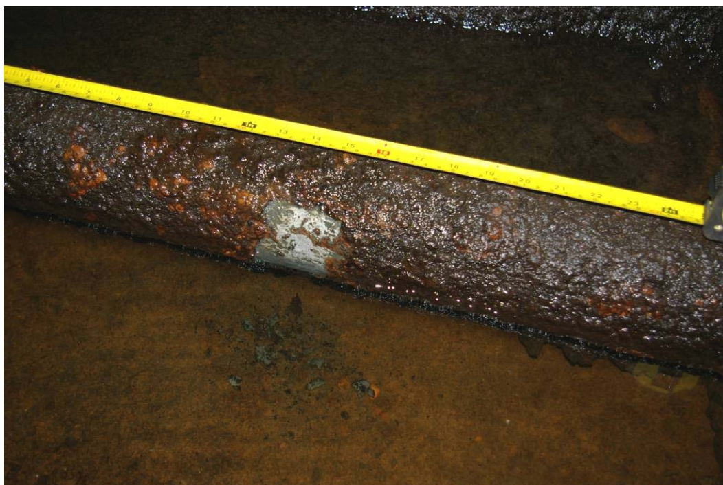
Photo 15 (August 15, 2007) East Supply Tunnel – Drain pipe measurement Location #1 – close up view. Pitting of pipe appears relatively shallow.
