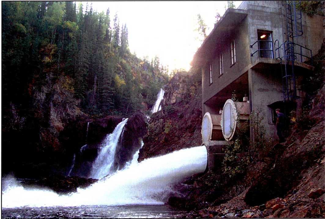
Figure 4: 36 in Hollow cone valve in operation.
