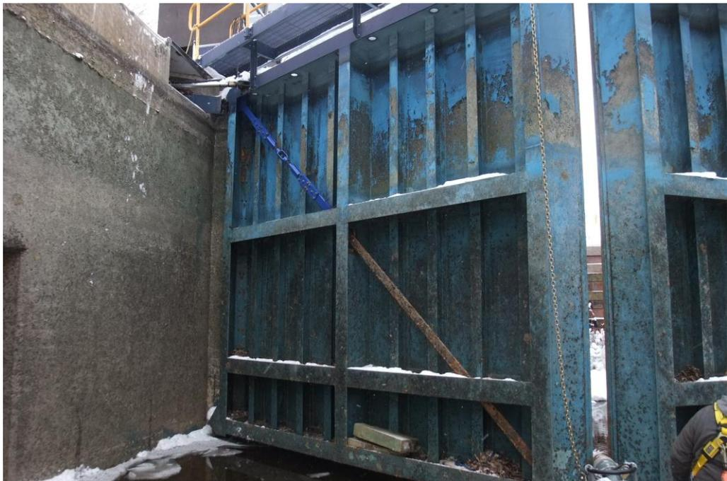
**Picture 4:** Picture showing downstream side of lower gates and railings. Railing and deck will be removed. Gate will be removed from lock chamber and set in laydown area on timbers.
