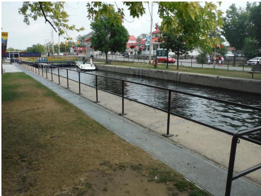
**Picture 12:** Picture of typical trench cover plates to be galvanized. Embedded steel to be painted with System 2. Railings to be replaced.
