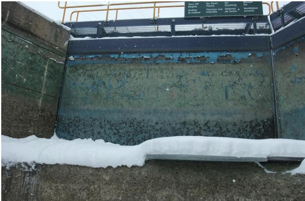
**Picture 4:** Picture showing downstream side of upper gates railings and deck. Railing and deck will be removed by Parks Canada. Gate will be removed from lock chamber by Parks Canada and set in laydown area on timbers.
