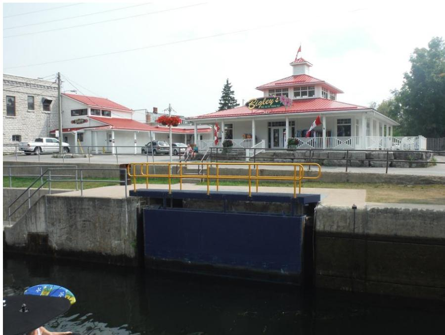
**Picture 10:** Picture of typical gate deck and railing. Decks and mounting brackets to be painted, railings to be replaced.
