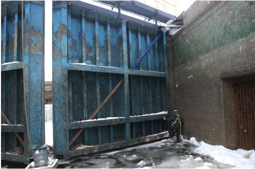
**Picture 3:** Picture of upstream side of lower gates. Note: Gates will be removed from lock chamber.
