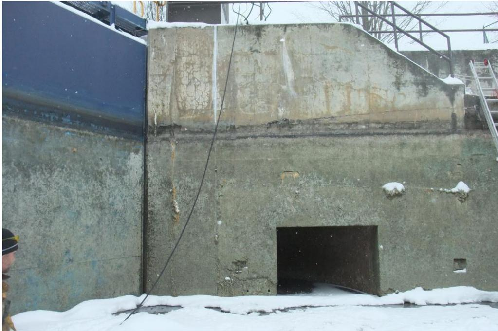
**Picture 7:** Picture of downstream side of lower gates showing water demarcation line. All non-submerged portions of gate to receive urethane finish.
