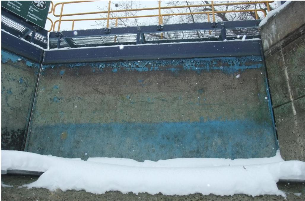
**Picture 5:** Picture of downstream side of upper gates. Note: gates will be removed from lock chamber by Parks Canada. Railings and deck will be removed from gate by Parks Canada.
