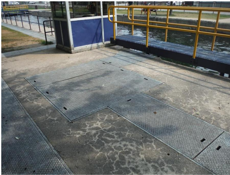
**Picture 11:** Picture of typical trench cover plates to be galvanized. Embedded steel to be painted with System 2.
