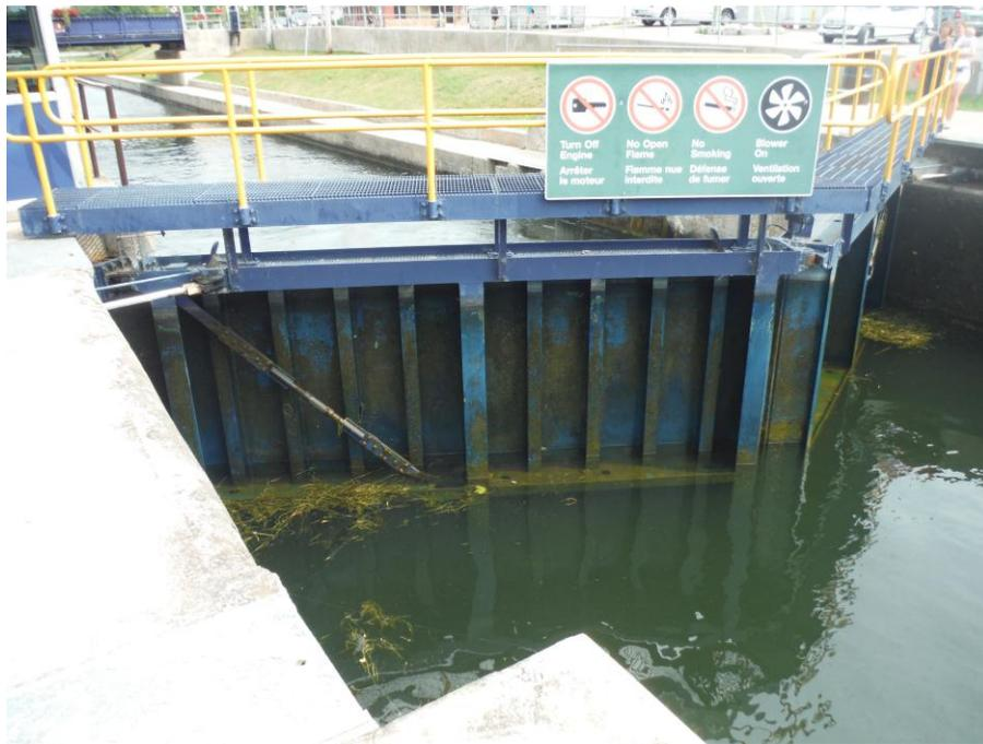
**Picture 9:** Picture of typical gate deck and railing. Decks and mounting brackets to be painted, railings to be replaced.
