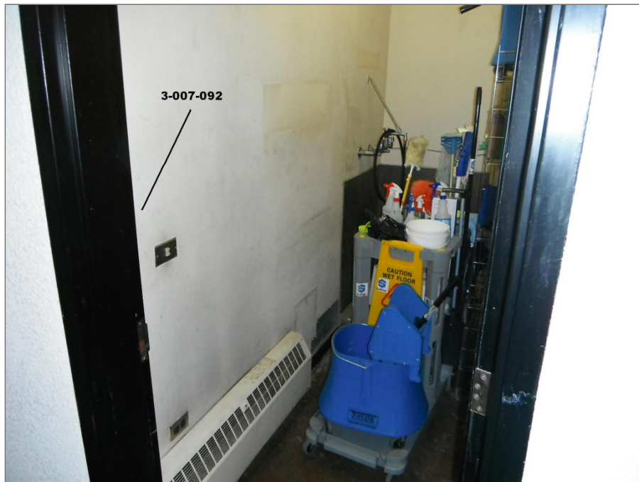
Photo 47: Asbestos-containing drywall joint compound applied to the interior wall of the janitorial room on the third floor. Tetra Tech sample 3-007-092.
