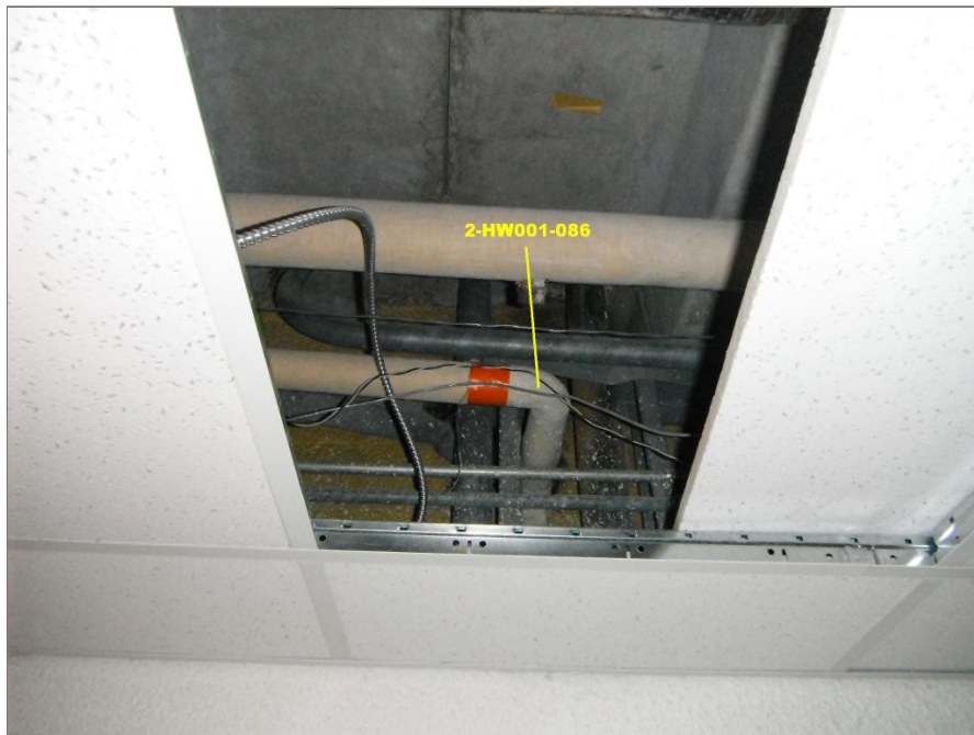
Photo 43: Asbestos-containing mudded insulation applied to the 2" diameter pipe elbow within the northeastern hallway of the second floor. Tetra Tech sample 2-HW001-086.
