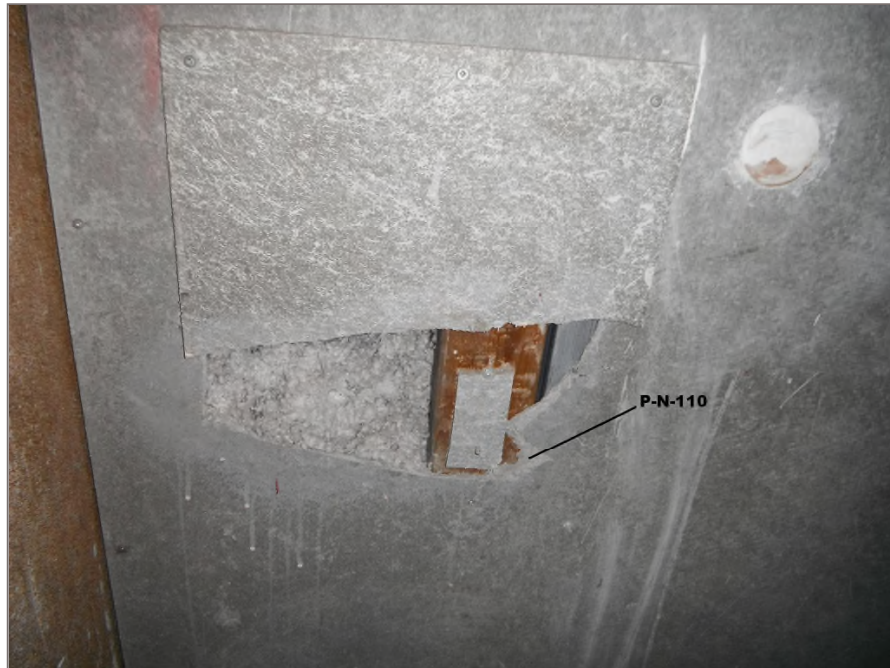
Photo 55: Asbestos-containing transite cement board applied to the perimeter walls of the penthouse. Tetra Tech sample P-N-110.
