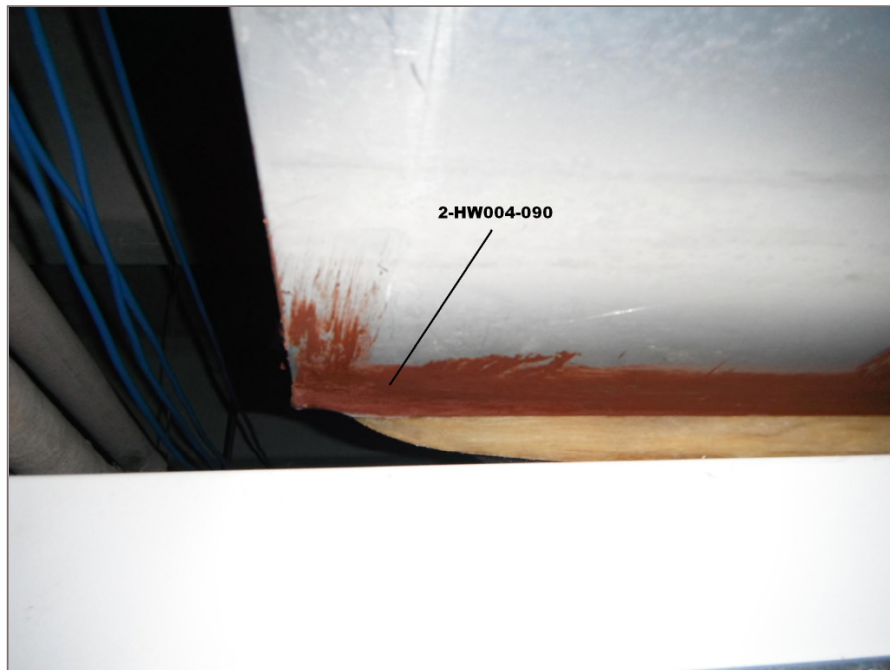
Photo 45: Asbestos-containing red mastic applied to the square HVAC ducting within the southwestern hallway of the second floor. Tetra Tech sample 2-HW004-090.
