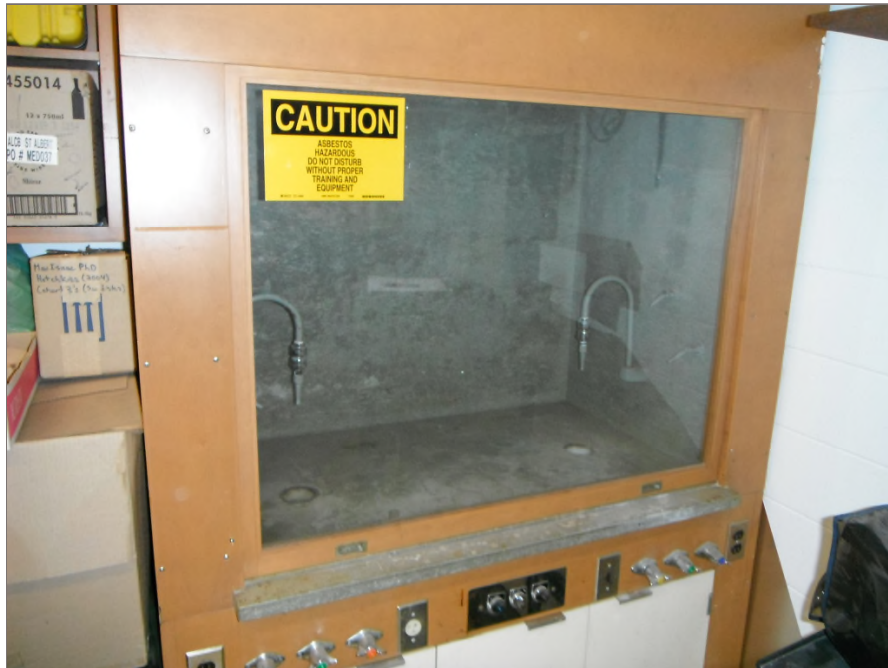
Photo 63: Asbestos-containing transite cement wall board present within a fume hood.
