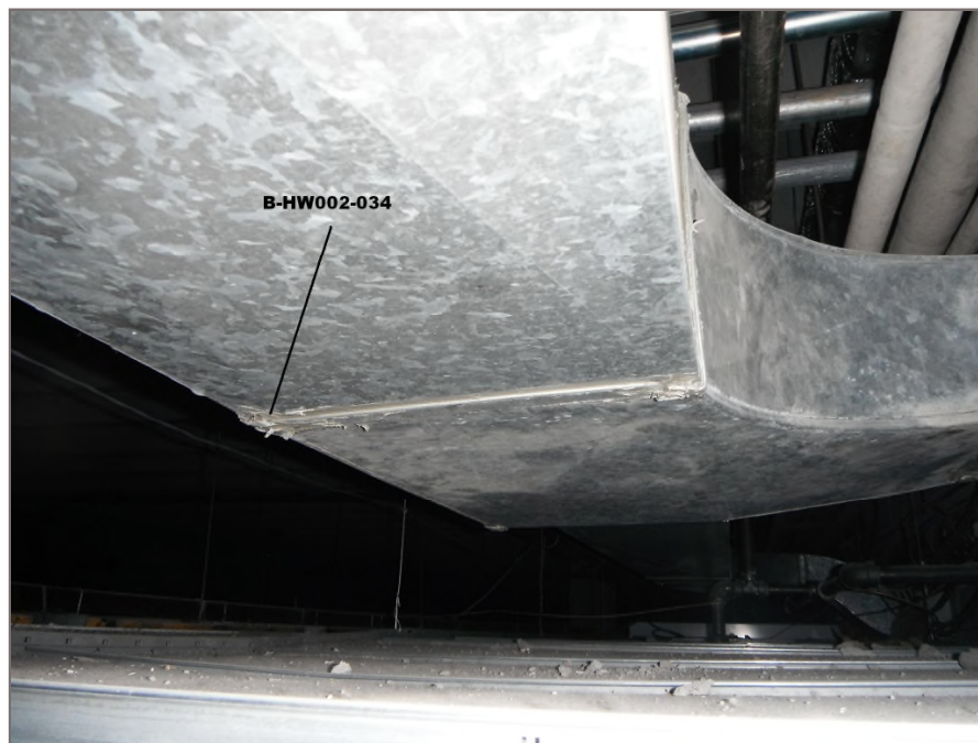
Photo 19: Asbestos-containing grey mastic applied to the HVAC ducting within the basement hallway ceiling space. Tetra Tech sample B-HW002-034.
