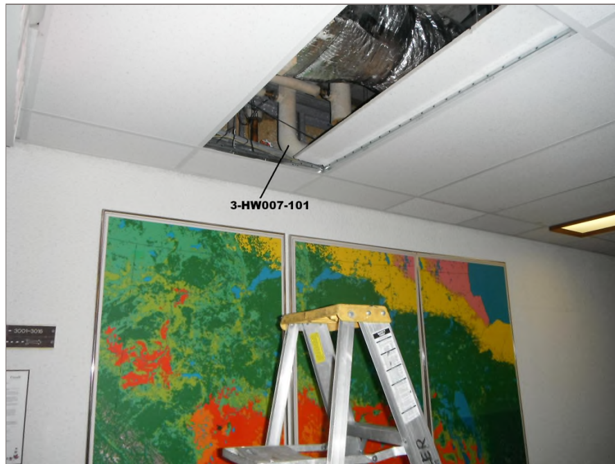
Photo 53: Asbestos-containing mudded insulation applied to the 2" diameter pipe elbow within the third floor central hallway ceiling space. Tetra Tech sample 3-HW007-101.
