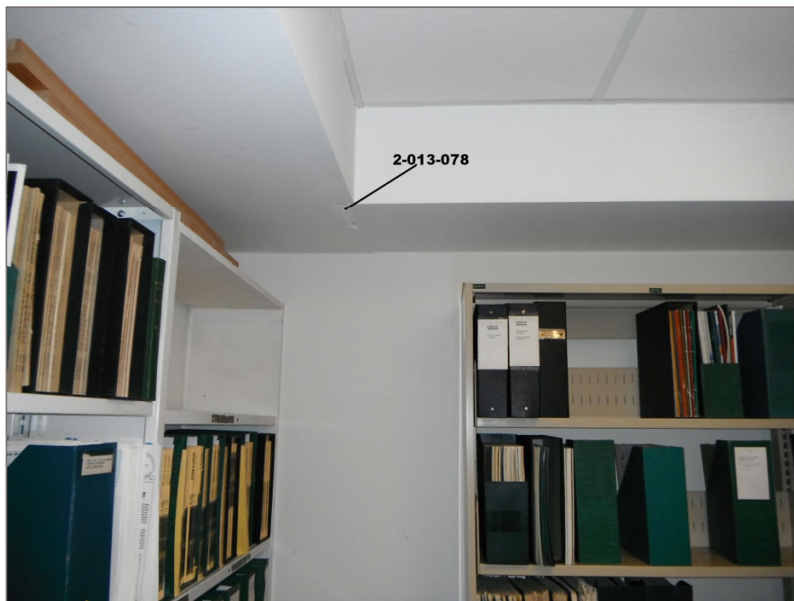
Photo 38: Asbestos-containing drywall joint compound applied to the bulkhead of the second floor library. Tetra Tech sample 2-013-078.
