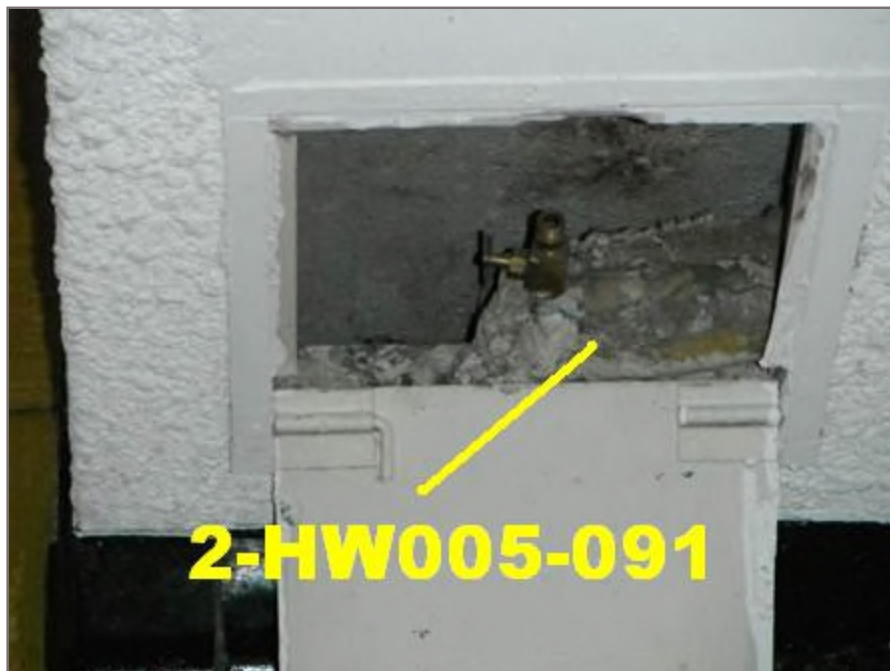
Photo 46: Asbestos-containing mudded insulation applied to the 2" diameter pipe elbow within the south hallway perimeter wall. Tetra Tech sample 2-HW005-091.
