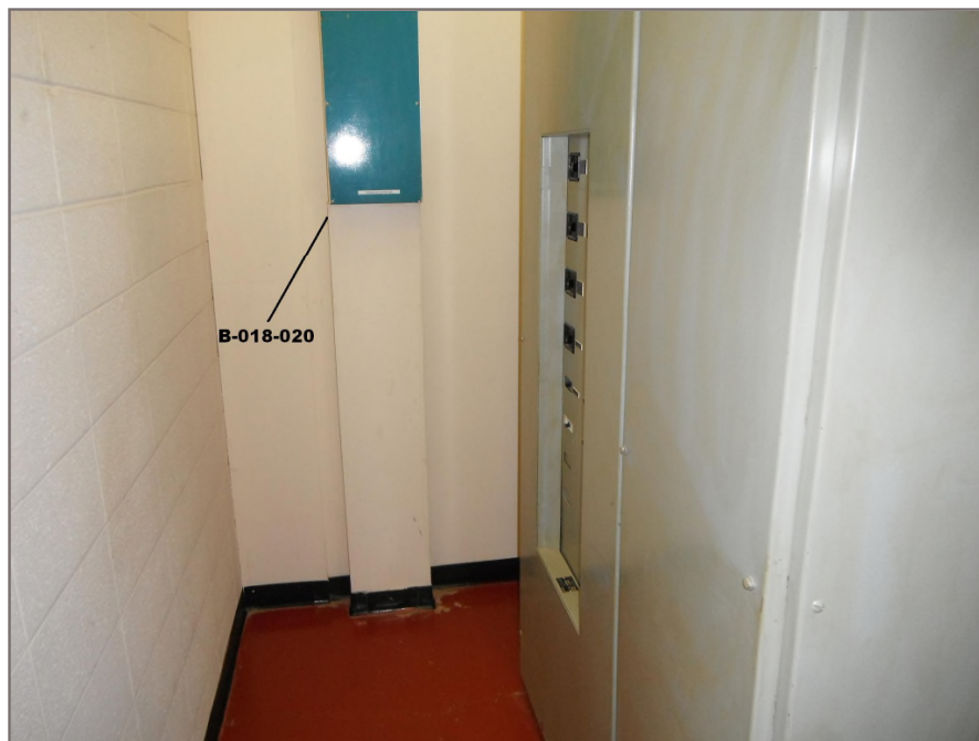
Photo 12: Asbestos-containing drywall joint compound associated with the column in the basement electrical room. Tetra Tech sample B-018-020.
