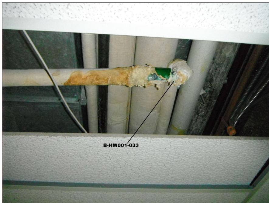
Photo 18: Asbestos-containing mudded pipe insulation applied to the elbow of a 2" diameter pipe within the basement hallway. Tetra Tech sample B-HW001-033.
