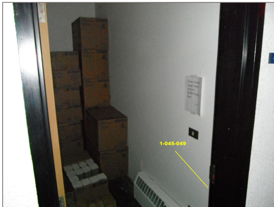
Photo 24: Asbestos-containing drywall joint compound applied to the wall of the first floor janitorial room. Tetra Tech sample 1-045-049.
