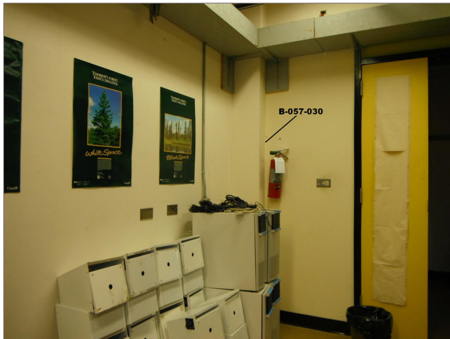
Photo 17: Asbestos-containing drywall joint compound applied to the column of the telephone room within the basement. Tetra Tech sample B-057-030.
