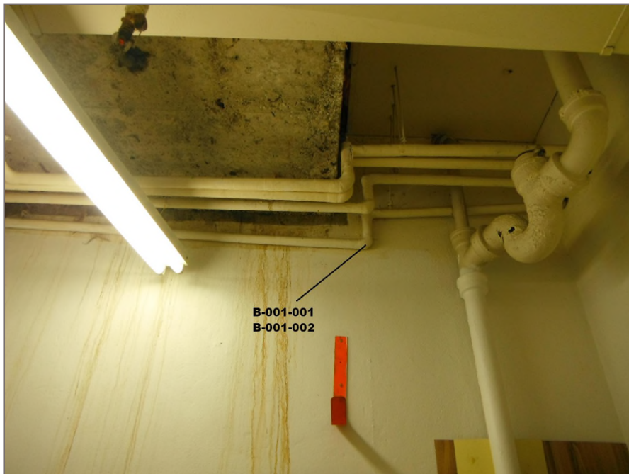
Photo 6: Asbestos-containing mudded pipe insulation applied to the 2" diameter pipe elbow in the basement storage room. Tetra Tech sample B-001-001.
