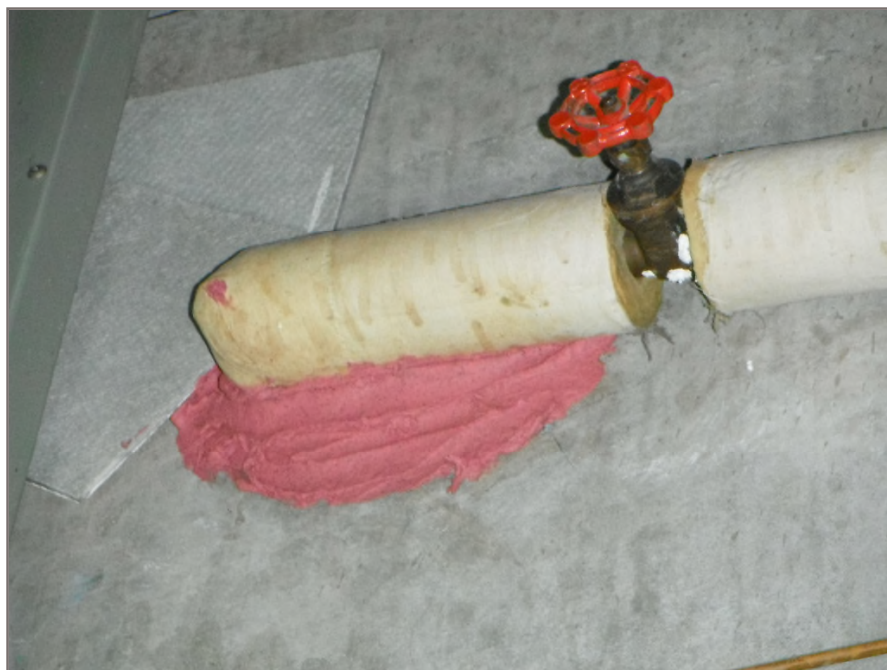
Photo 61: Asbestos-containing mudded mechanical insulation applied to exhaust fan #49 within the south end of the penthouse adjacent to the exit door. Tetra Tech sample P-S-130.
