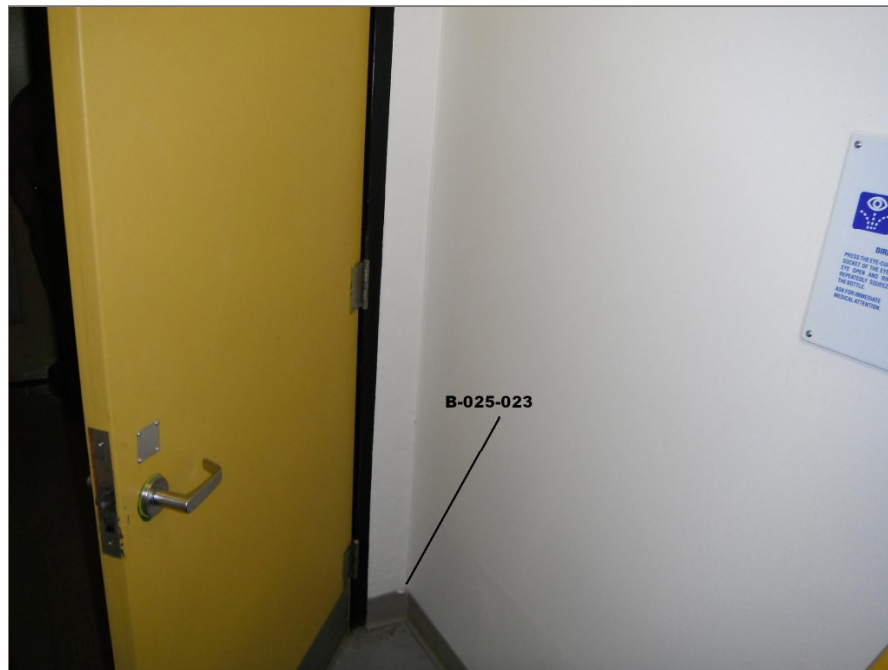
Photo 13: Asbestos-containing drywall joint compound applied to the interior wall of the basement janitor room. Tetra Tech sample B-025-023.
