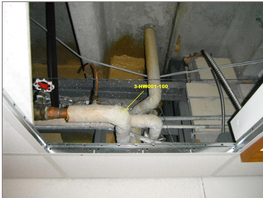
Photo 52: Asbestos-containing mudded insulation applied to the 2" diameter pipe elbow within the third floor northeastern hallway ceiling space. Tetra Tech sample 3-HW001-100.
