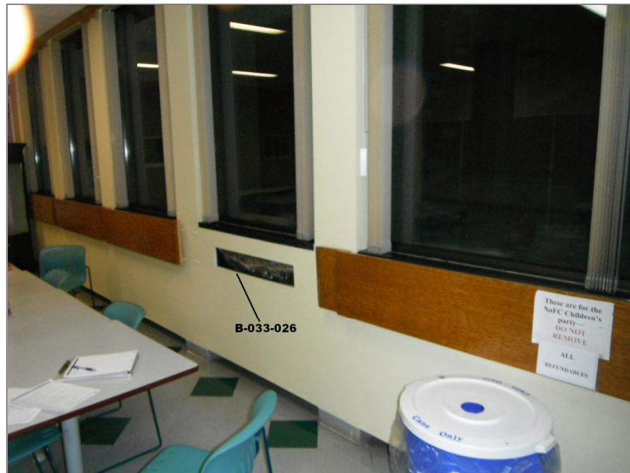
Photo 15: Asbestos-containing drywall joint compound applied to the perimeter wall of the lunch room within the basement. Tetra Tech sample B-033-026.
