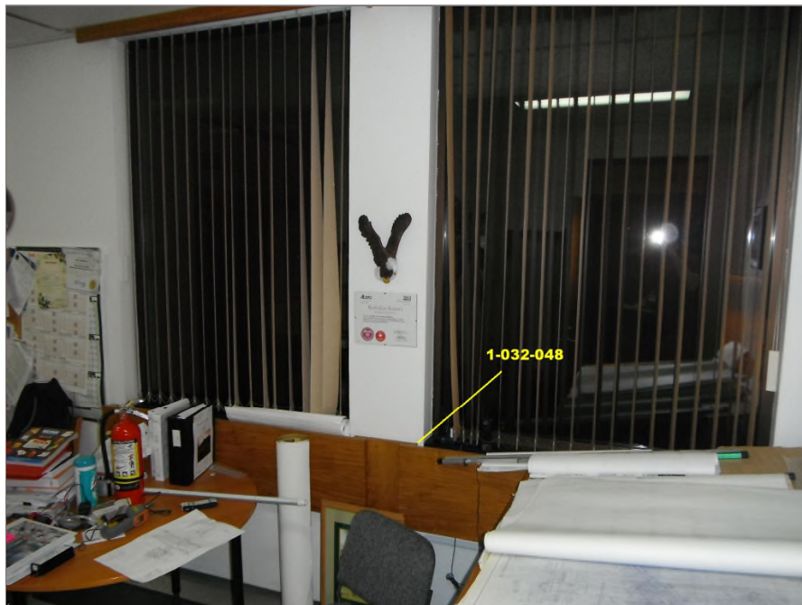
Photo 23: Asbestos-containing drywall joint compound associated with the perimeter wall of a first floor office. Tetra Tech sample 1-032-048.
