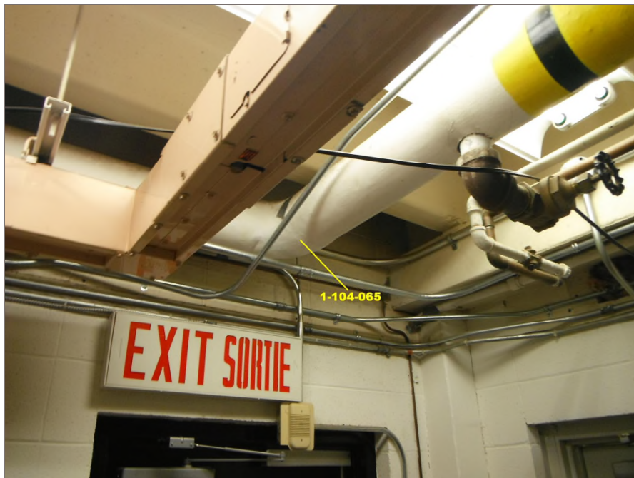
Photo 33: Asbestos-containing mudded insulation applied to the 6" diameter pipe elbow within the laboratory. Tetra Tech sample 1-104-065.
