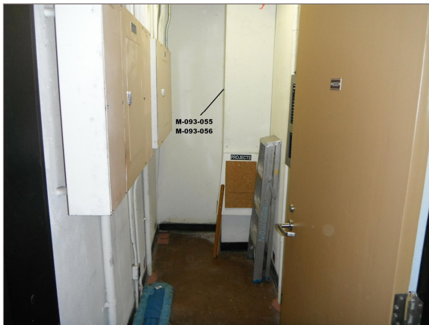
Photo 28: Asbestos-containing drywall joint compound associated with the walls of a janitorial room on the first floor. Tetra Tech sample 1-093-055.
