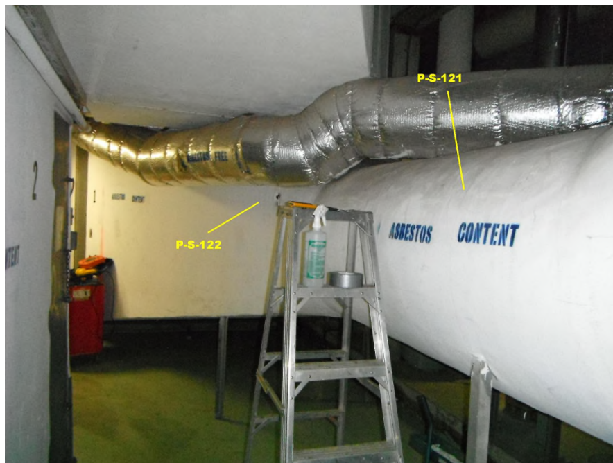
Photo 66: Asbestos-containing mudded mechanical insulation applied to the AHU #1 cold deck within the penthouse. Tetra Tech sample P-S-122.
