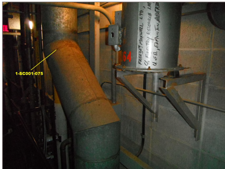
Photo 36: Asbestos-containing silver mastic applied to the 16" diameter pipe within the south service corridor of the first floor. Tetra Tech sample 1-SC001-075.
