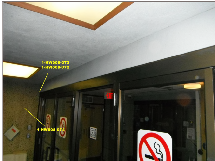
Photo 35: Asbestos-containing brown mastic applied to the door frame of the northwest entrance. Tetra Tech sample 1-HW008-072.
