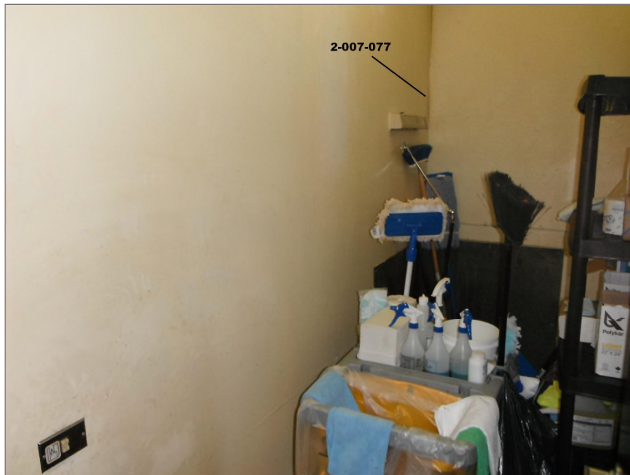
Photo 37: Asbestos-containing drywall joint compound applied to the interior wall of the second floor janitorial room. Tetra Tech sample 2-007-077.
