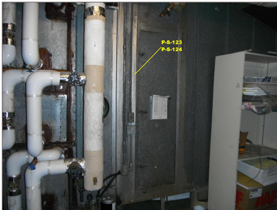
Photo 59: Asbestos-containing grey mastic applied to the metal ducting around the door of the AHU #2 cold deck within the penthouse. Tetra Tech sample P-S-123.
