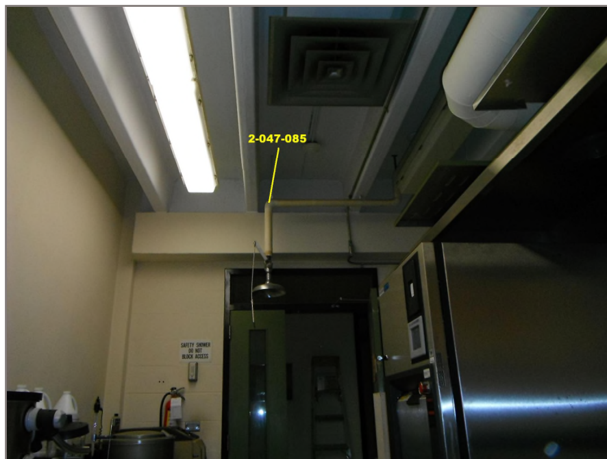
Photo 42: Asbestos-containing mudded insulation applied to the 2" diameter pipe elbow within the second floor laboratory. Tetra Tech sample 2-047-085.
