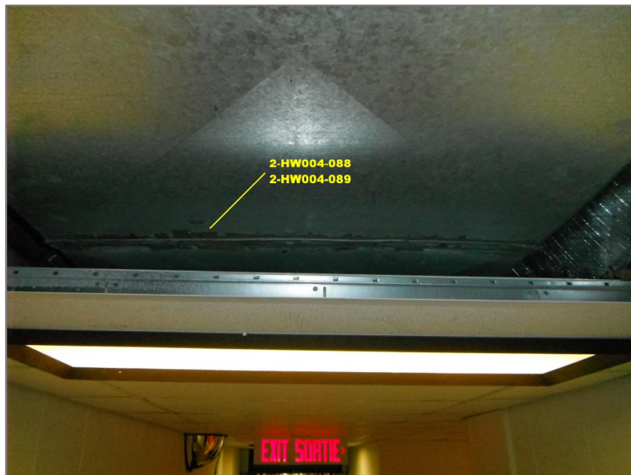
Photo 44: Asbestos-containing grey mastic applied to the square HVAC ducting within the southwestern hallway of the second floor. Tetra Tech sample 2-HW004-088.
