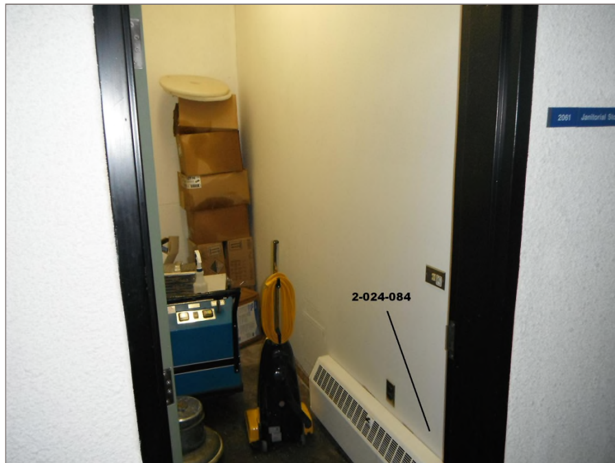
Photo 41: Asbestos-containing drywall joint compound applied to the interior wall of the second floor janitorial room. Tetra Tech sample 2-024-084.
