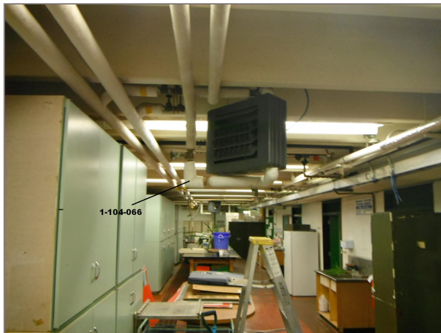
Photo 34: Asbestos-containing mudded insulation applied to the 2" diameter pipe elbow within the laboratory. Tetra Tech sample 1-104-066.
