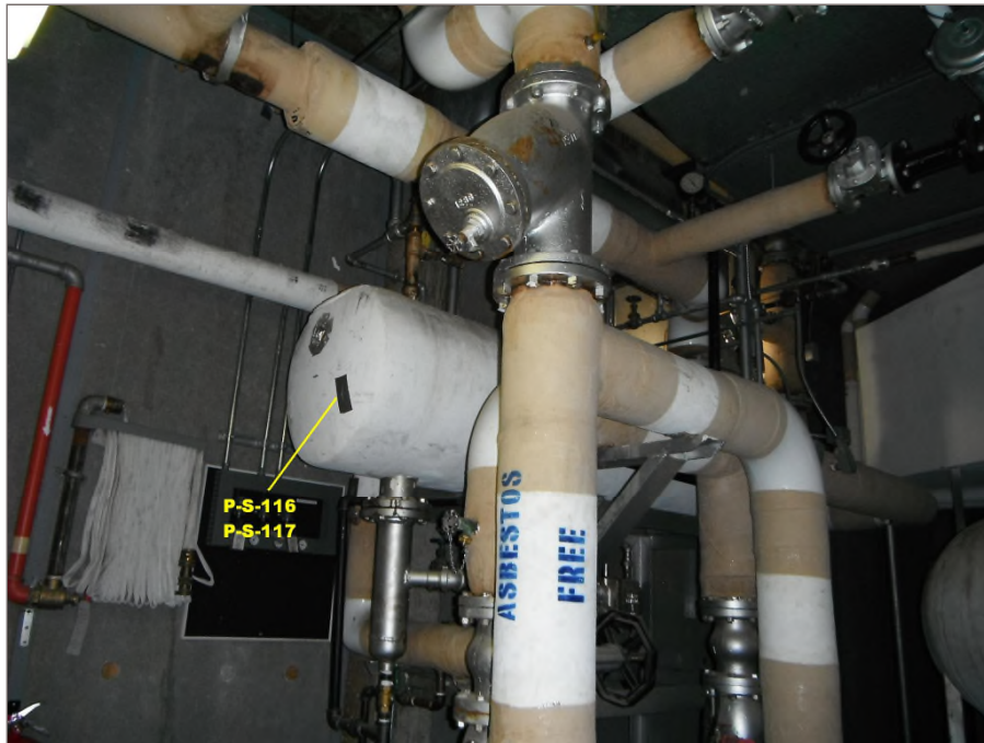
Photo 57: Asbestos-containing mudded mechanical insulation applied to the glycol heat exchanger within the penthouse. Tetra Tech sample P-S-116.
