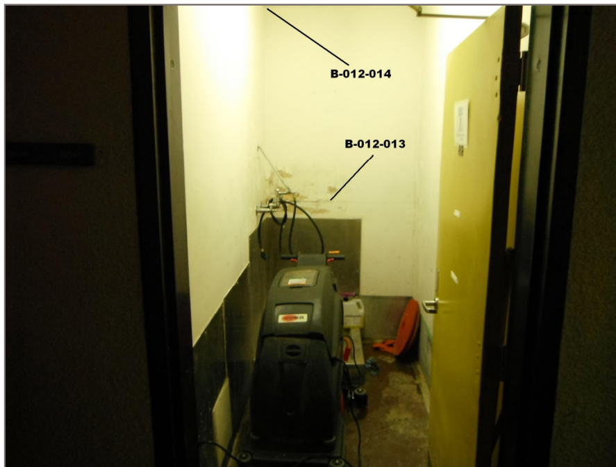
Photo 9: Asbestos-containing drywall joint compound applied to the walls and ceiling of the janitorial room within the basement. Tetra Tech sample B-012-013/014.
