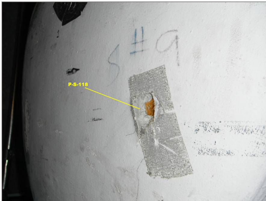
Photo 58: Asbestos-containing mudded mechanical insulation applied to the AHU #2 cold and hot decks within the penthouse. Tetra Tech sample P-S-118.
