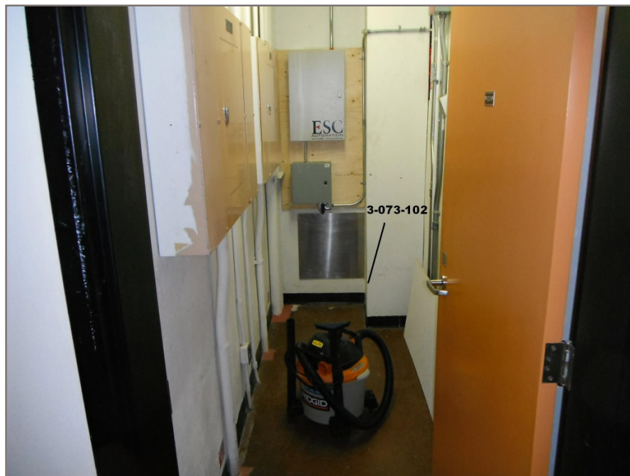
Photo 54: Asbestos-containing drywall joint compound applied to the interior column of the third floor janitorial room. Tetra Tech sample 3-073-102.
