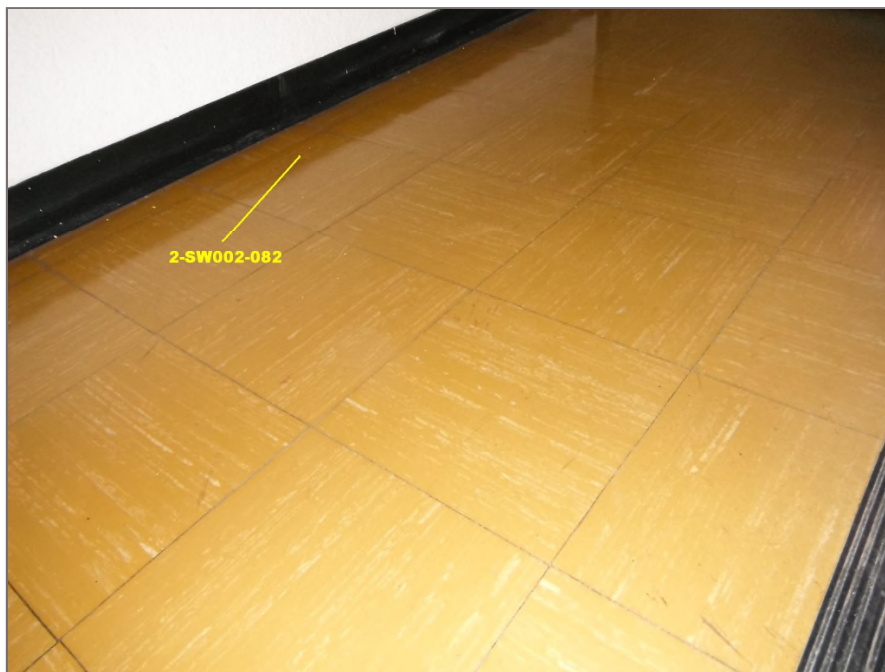
Photo 40: Asbestos-containing 12"x12" olive vinyl floor tiles within the southwestern stairwell. Tetra Tech sample 2-SW002-082.
