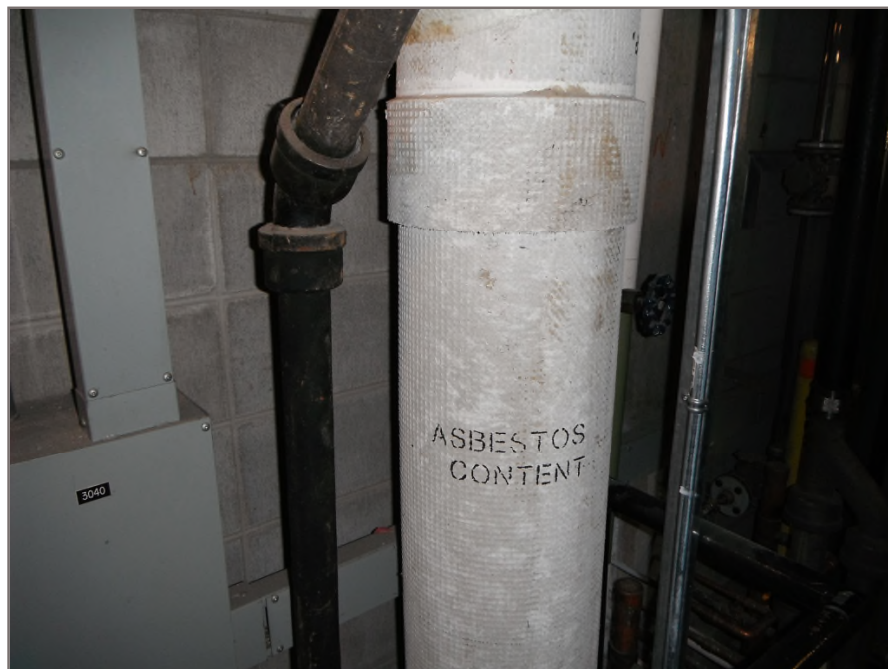
Photo 64: Asbestos-containing transite cement pipe present within the Penthouse.
