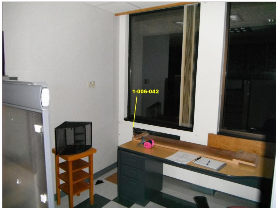
Photo 21: Asbestos-containing drywall joint compound applied to the perimeter wall of a cubicle space in the east wing. Tetra Tech sample 1-006-042.
