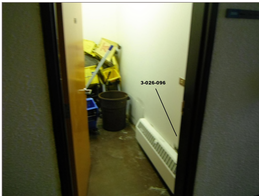
Photo 50: Asbestos-containing drywall joint compound applied to the interior wall of the janitorial room on the third floor. Tetra Tech sample 3-026-096.
