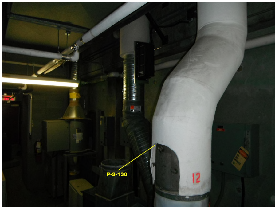
Photo 61: Asbestos-containing mudded mechanical insulation applied to exhaust fan #49 within the south end of the penthouse adjacent to the exit door. Tetra Tech sample P-S-130.
