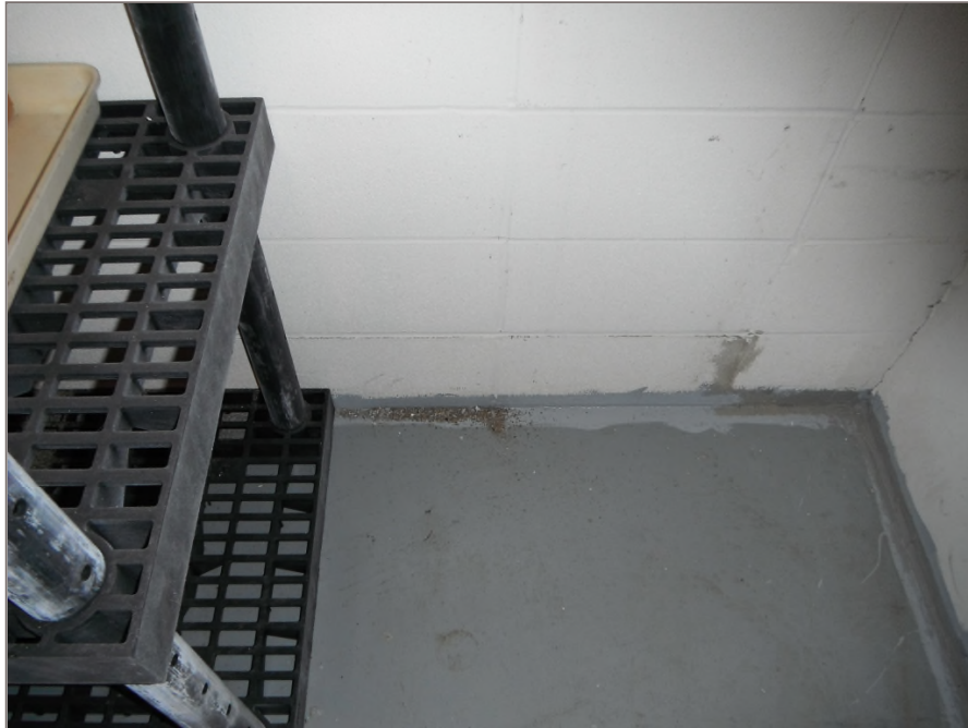
Photo 65: Vermiculite insulation present on the floor of the HAZMAT shed storage room.
