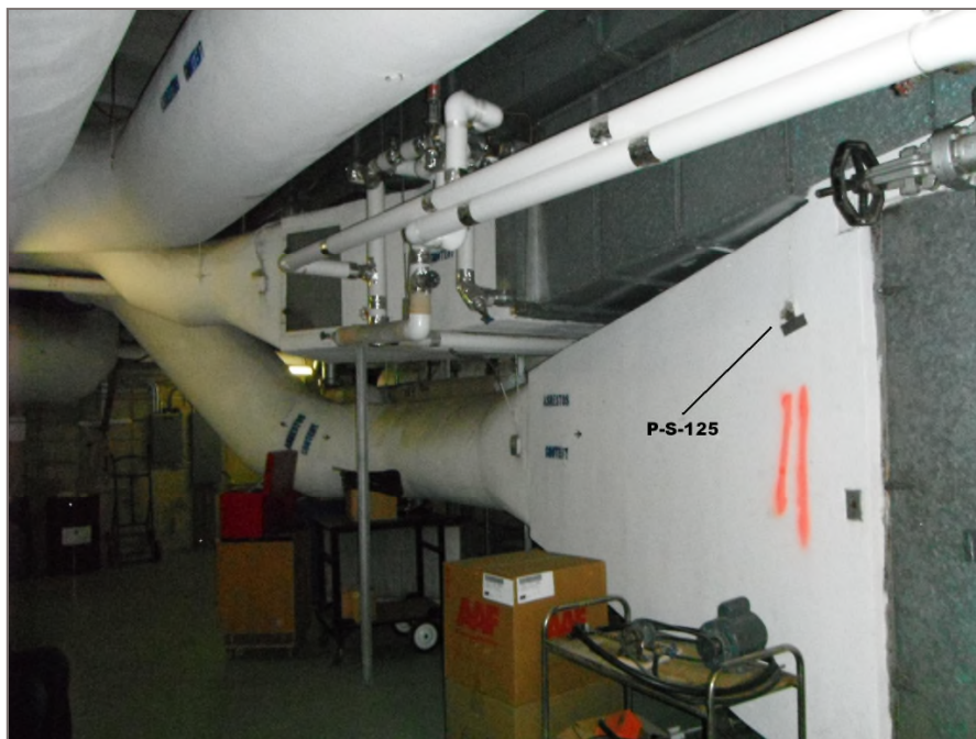
Photo 60: Asbestos-containing mudded mechanical insulation applied to the AHU #2 cold deck within the penthouse. Tetra Tech sample P-S-125.
