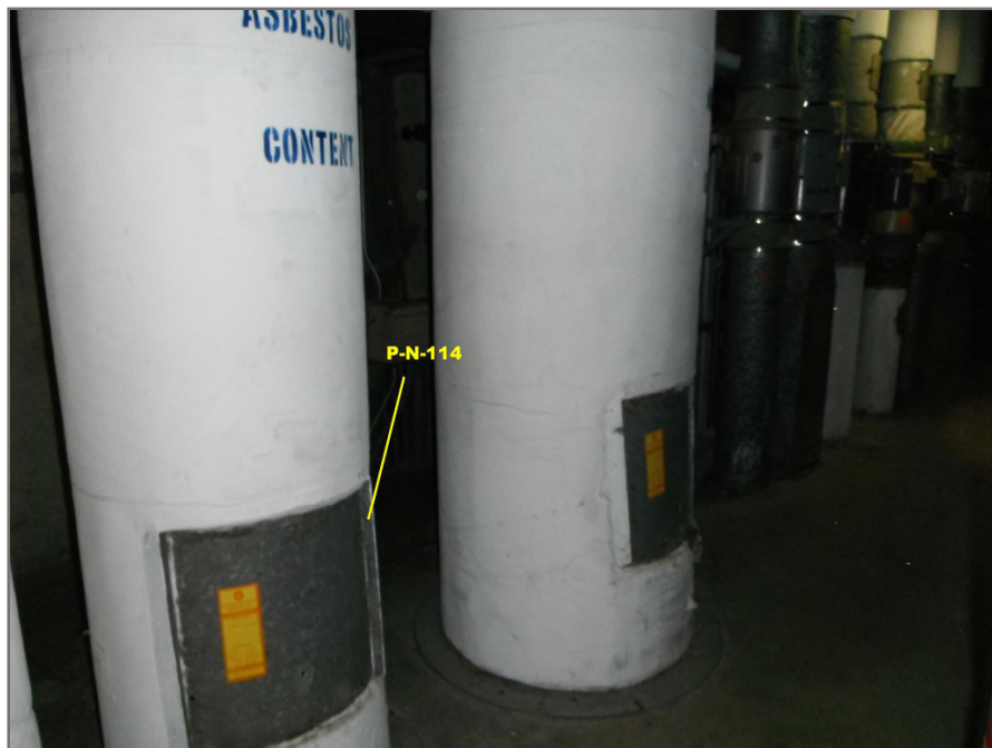
Photo 56: Asbestos-containing mudded mechanical insulation applied to the 24" diameter pipe within the penthouse. Tetra Tech sample P-N-114.
