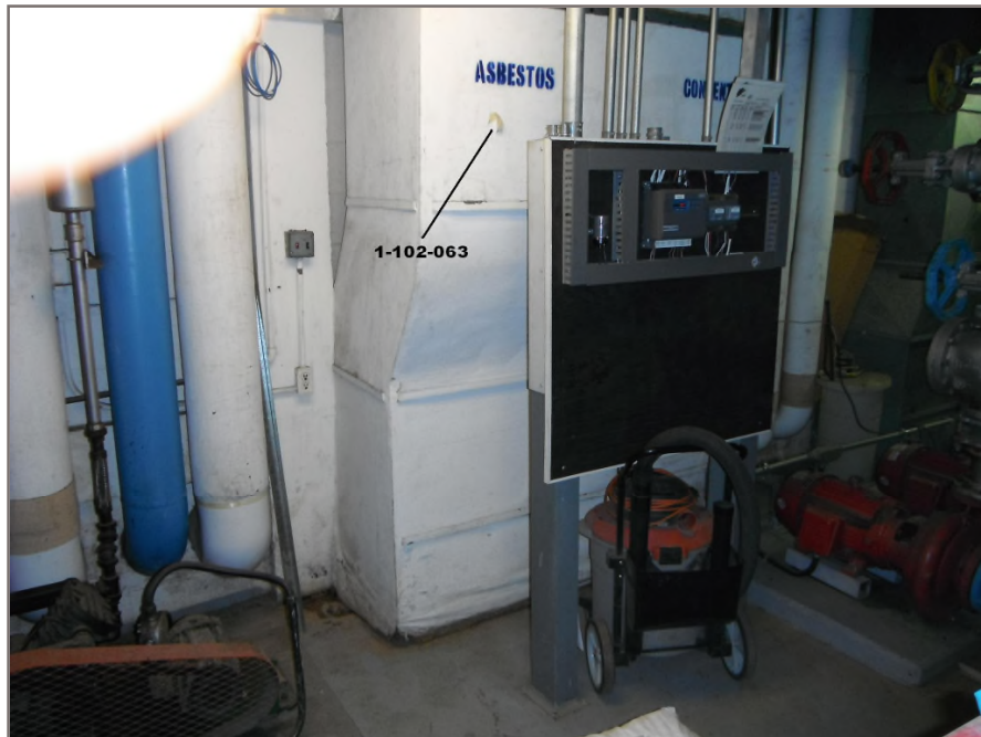
Photo 32: Asbestos-containing mudded insulation applied to the air handling unit located at the north end of the boiler room. Tetra Tech sample 1-102-063.
