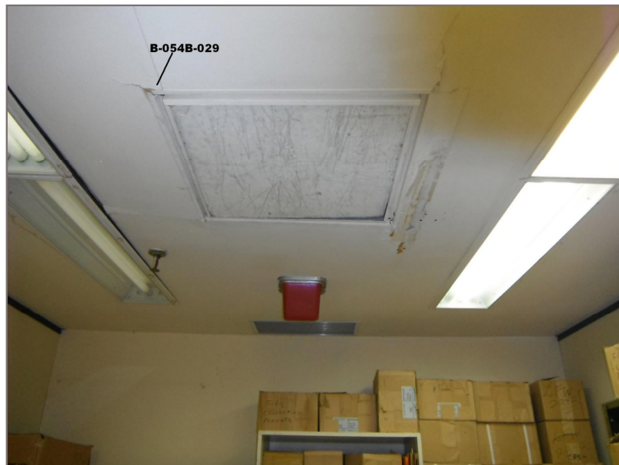
Photo 16: Asbestos-containing drywall joint compound applied to the ceiling of the office space within the basement. Tetra Tech sample B-054B-029.
