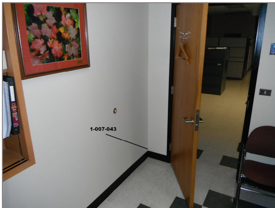
Photo 22: Asbestos-containing drywall joint compound associated with the interior wall of an office space in the east wing. Tetra Tech sample 1-007-043.
