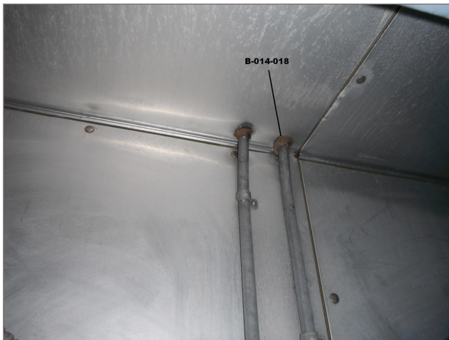
Photo 10: Asbestos-containing tan putty applied to the pipe penetration of the walk-in cooler within the basement. Tetra Tech sample B-014-018.
