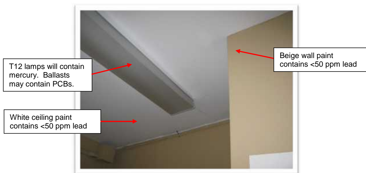
Photo 6: Typical fluorescent light fixture. The T12 lamps will contain liquid mercury which vapourizes when the lamp is energized. The fixture may contain a PCB ballast. White ceiling paint and beige wall paint have both been tested and confirmed to contain <50 ppm lead.
