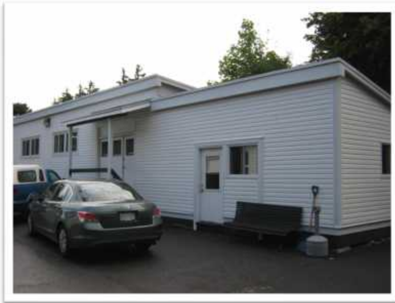
Photo 1: Exterior view of the Shop. Asphaltic roofing materials and window caulking are both non-friable suspected ACMs.
