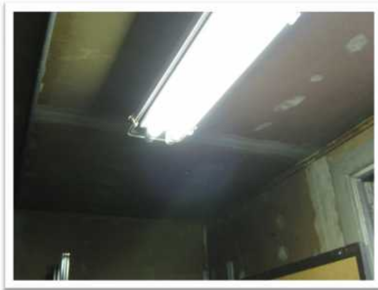
Photo 5: Typical fluorescent light fixture. Each light tube will contain a single droplet of mercury. The ballasts are also suspected to contain PCBs.
