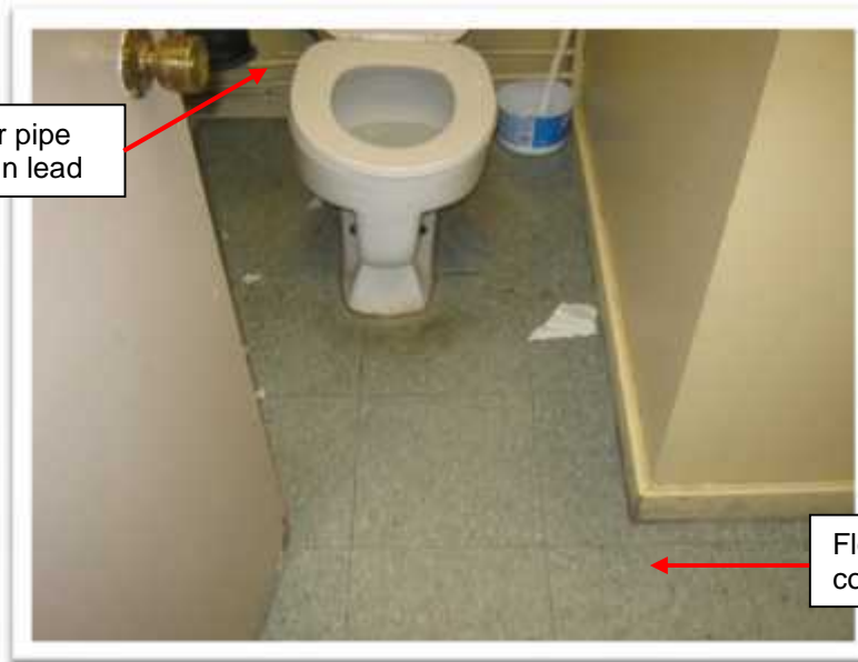
Photo 3: Vinyl floor tiles in Survey Location #5 (Bathroom) have been tested (Samples 94189-03A-C) and confirmed to contain no asbestos.
