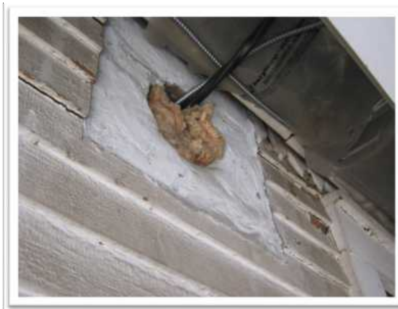
Photo 2: Parging cement over redundant opening in the west wall. Laboratory analysis has confirmed that the material (Sample 335846-01) does not contain asbestos.
