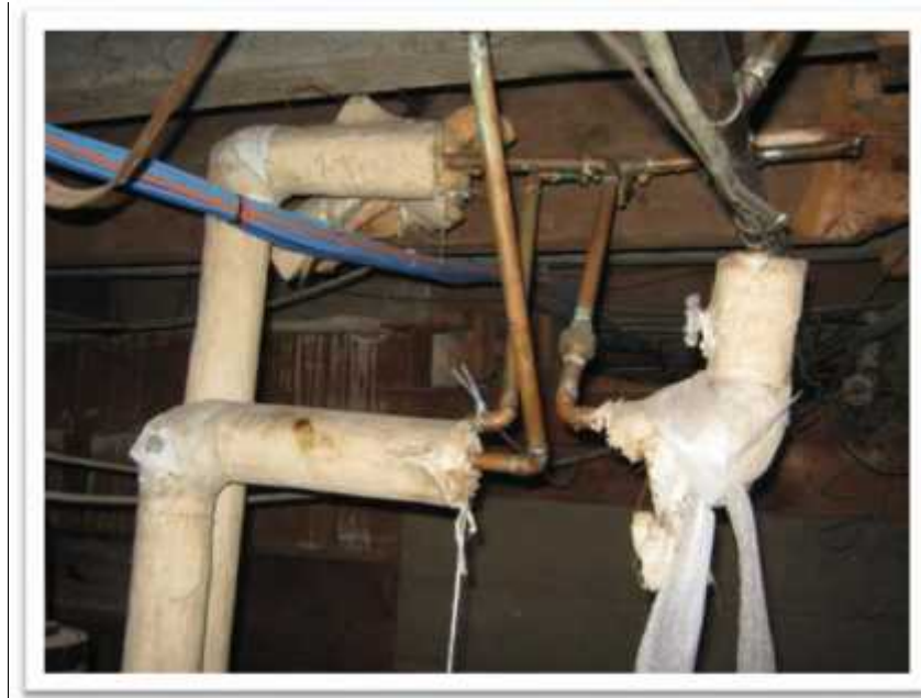
Photo 7: Grey cement compound on pipe fittings in the basement mechanical/storage room contains 90% chrysotile asbestos (Sample 243867-04-A). There are 4 fittings exposed and in POOR condition.
