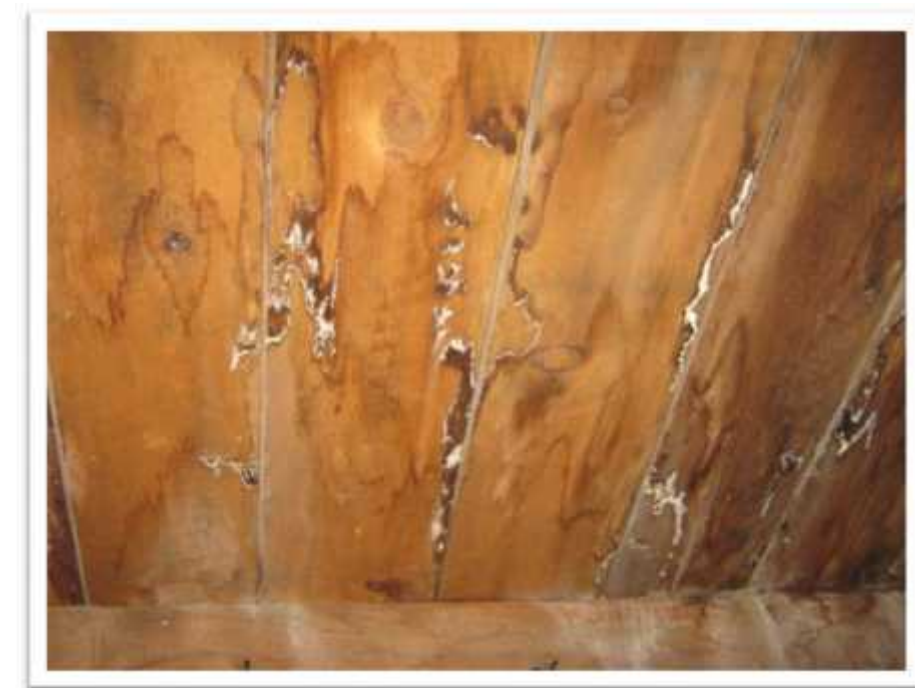
Photo 6: Mould impacted underside of wooden floorboards (Sample 243867-TL-01) was observed in the basement storage room. Affected area is approximately 10 square metres total.
