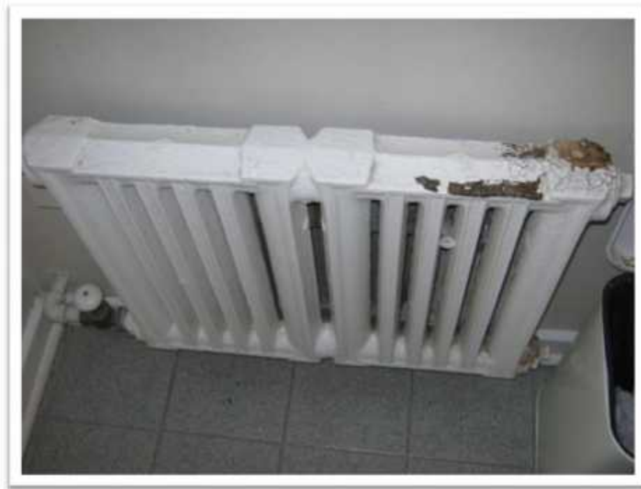
Photo 13: White radiator paint (Sample 243867-LP-01) contains 19,800 ppm lead.
