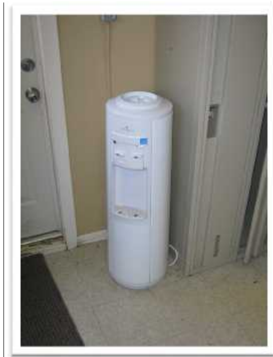
Photo 7: Typical water cooler will contain an ODS-suspect refrigerant. Refrigerators and window mounted air conditioners will also contain ODS-suspect refrigerants. None of this equipment is an integral part of the building structure or its finishes.
