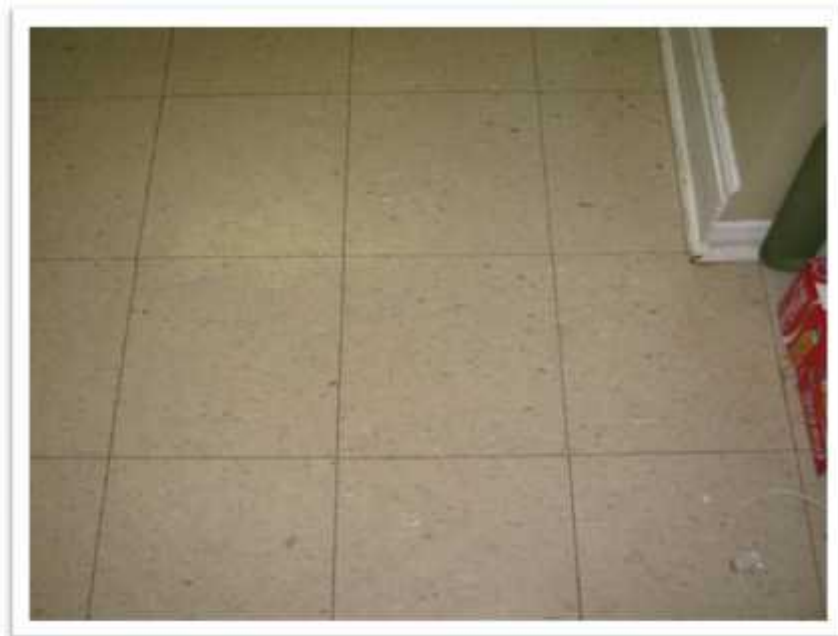
Photo 12: Brown 12" x 12" vinyl tile flooring sampled in the ground floor rear common area does not contain asbestos (Samples 243867-09A-C).
