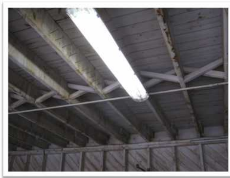
Photo 7: Typical fluorescent light fixture with T8 tubes is not expected to contain a PCB ballast. Each tube will, however, contain a droplet of mercury which vapourizes when the tube is energized.
