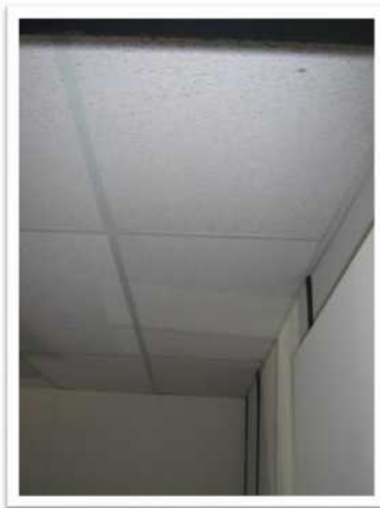
Photo 14: 2' x 4' lay-in ceiling tile sampled in the ground floor front offices does not contain asbestos (Samples 243867-10A-C).
