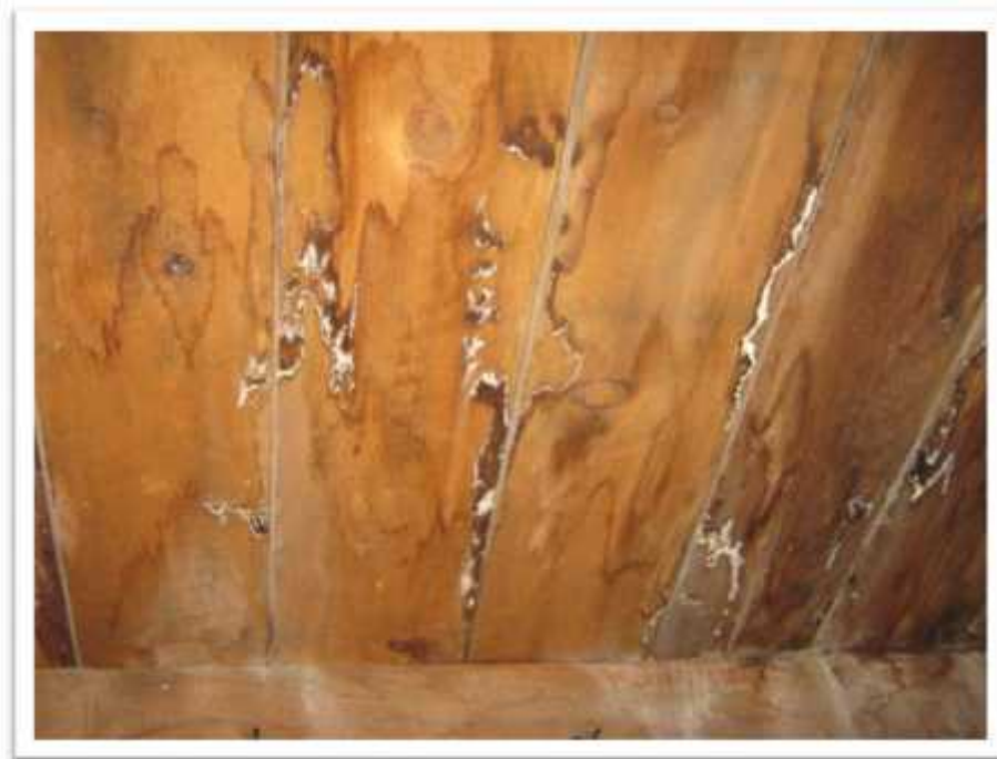
Photo 6: Mould impacted underside of wooden floorboards (Sample 243867-TL-01) was observed in the basement storage room. Affected area is approximately 10 square metres total.
