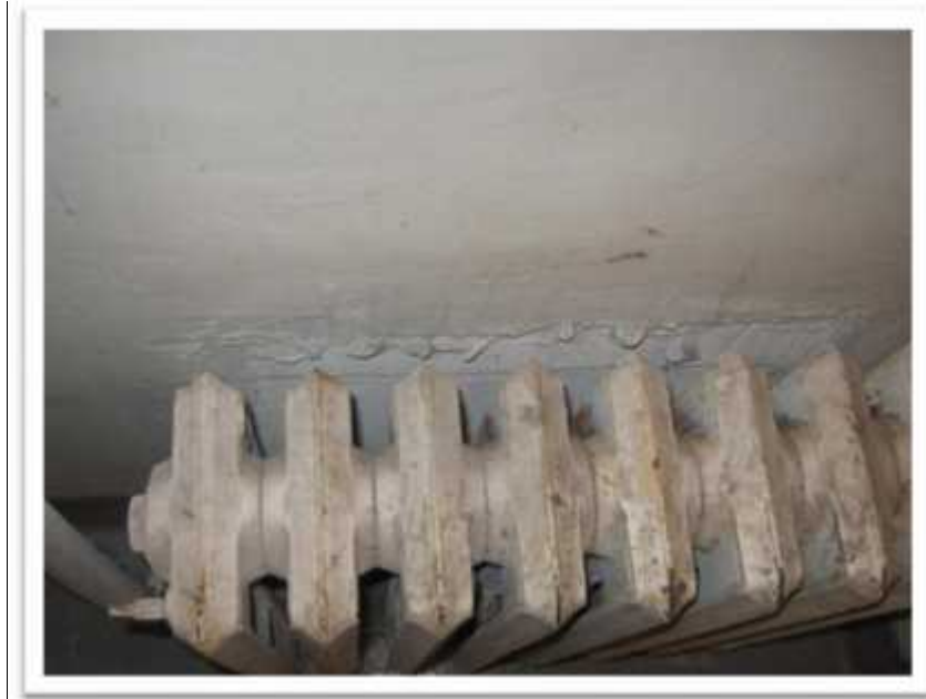
Photo 3: Wall surfacing material (Samples 243867-01A-E) sampled in the Garage washroom does not contain asbestos.
