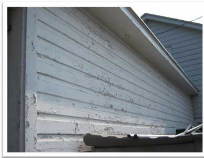
Photo 5: Exterior white paint (Sample 335846-LP-01) contains 13,700 ppm lead. This paint is delaminating from its wood substrate and is in POOR condition. Remedial action is required.
