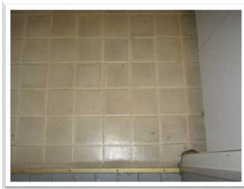
Photo 9: Light brown coloured vinyl sheet flooring (Samples 243867 06A-C) sampled does not contain asbestos (ground floor shower room pictured here).
