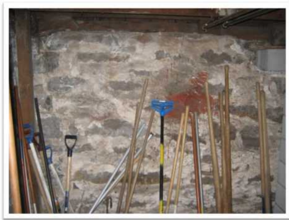
Photo 5: Stonework surface parging material (Samples 243867-03A-E) sampled does not contain asbestos.
