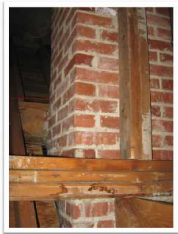
Photo 19: Chimney brick mortar sampled does not contain asbestos (Samples 243867-14A-C).
