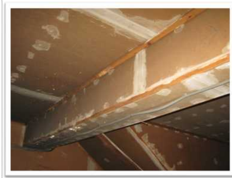
Photo 3: Drywall joint compound has been tested and does not contain regulated concentrations of asbestos.
