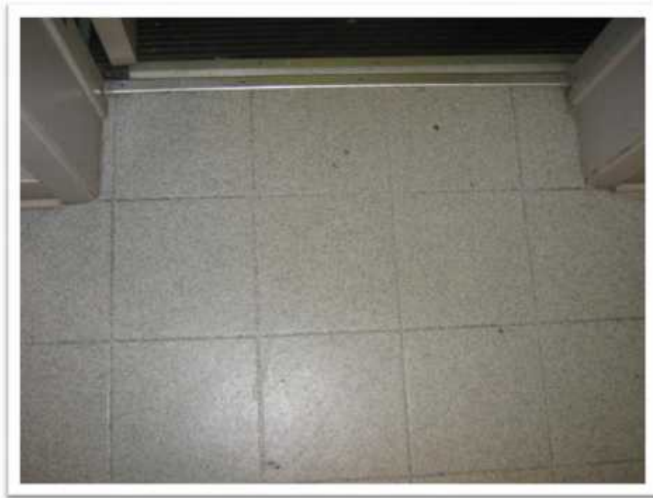
Photo 15: Grey/blue vinyl sheet flooring sampled throughout the ground floor does not contain asbestos (Samples 243867-11A-C).
