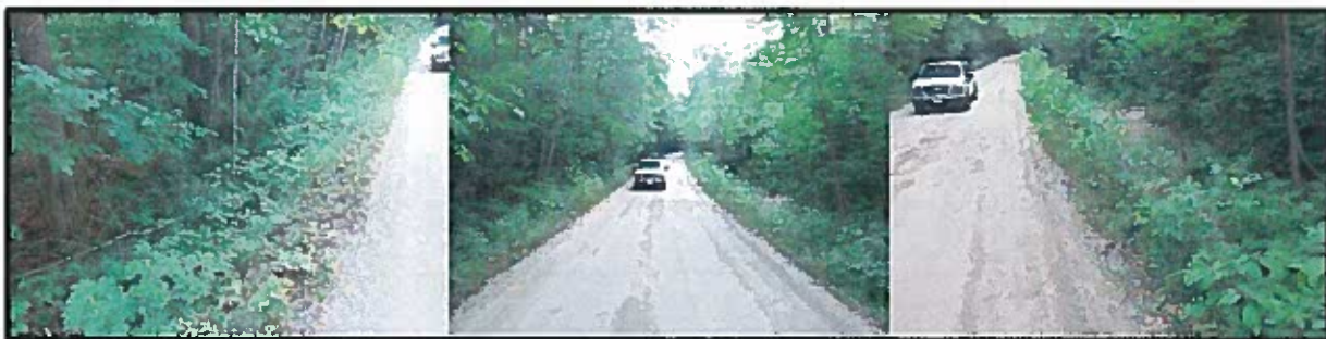
Photo 9- Photos for point 16 showing the steep drop offs on both sides of the road. Road widen will be limited to maintain shoulder stability and caution signage installed. Photos taken heading away from highway.
