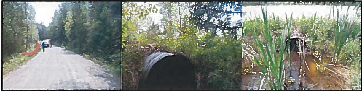
Photo 6 - Photo of location 9 to 11. First photo taken heading toward Highway 6, second photo is of culvert on northwest side of road and the third is of the culvert on the southeast side. The culvert exit/entrance on the northwest side has a deep plunge pool that fish are enable to pass at lower water levels, therefore, a fish ladder should be installed in enable passage.
