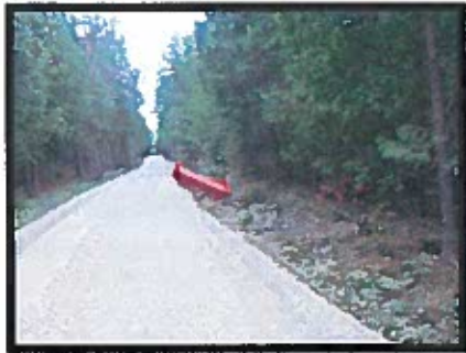
Photo1- Photo of rock outcrop at point 1. Shot taken facing southwest (i.e., traveling towards the highway). Red arrow showing rocks that will need to be moved further into forest edge.
