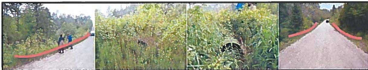
Photo 5- Photo series for points 6 and 7 showing the present culvert and approximate location for eco-fencing. An ecopassage will be installed near the location of the culvert. Red lines indicate a rough path for the fencing to follow. First photo is taken heading towards highway 6, the last one is taken heading away.
