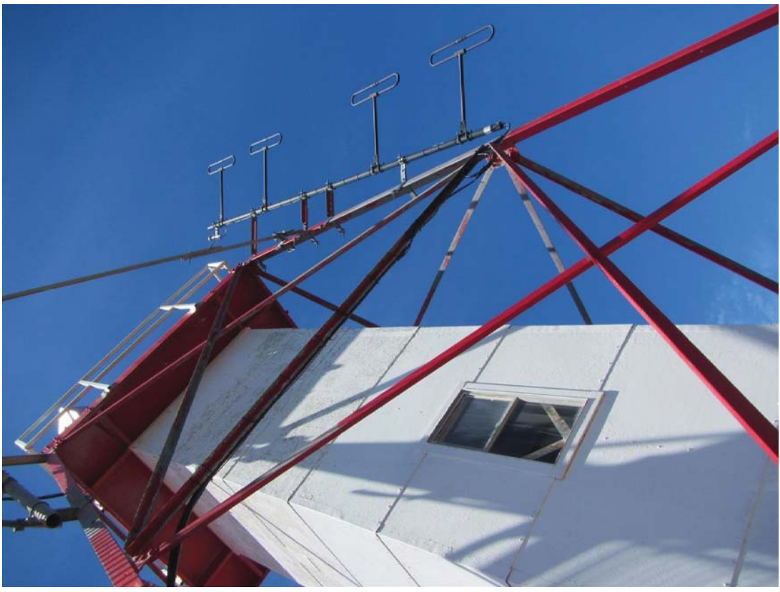
Two antennas attached to tower, do not work affront.
