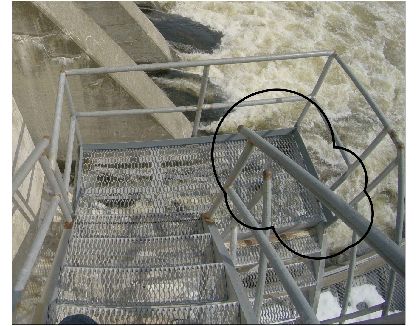
NOTE 8: TYP. CUT OUT AND REPLACE 1.3m 50mm GALVANIZED STEEL PIPE FOR RAILING WHERE CRACKED/SPLIT.
