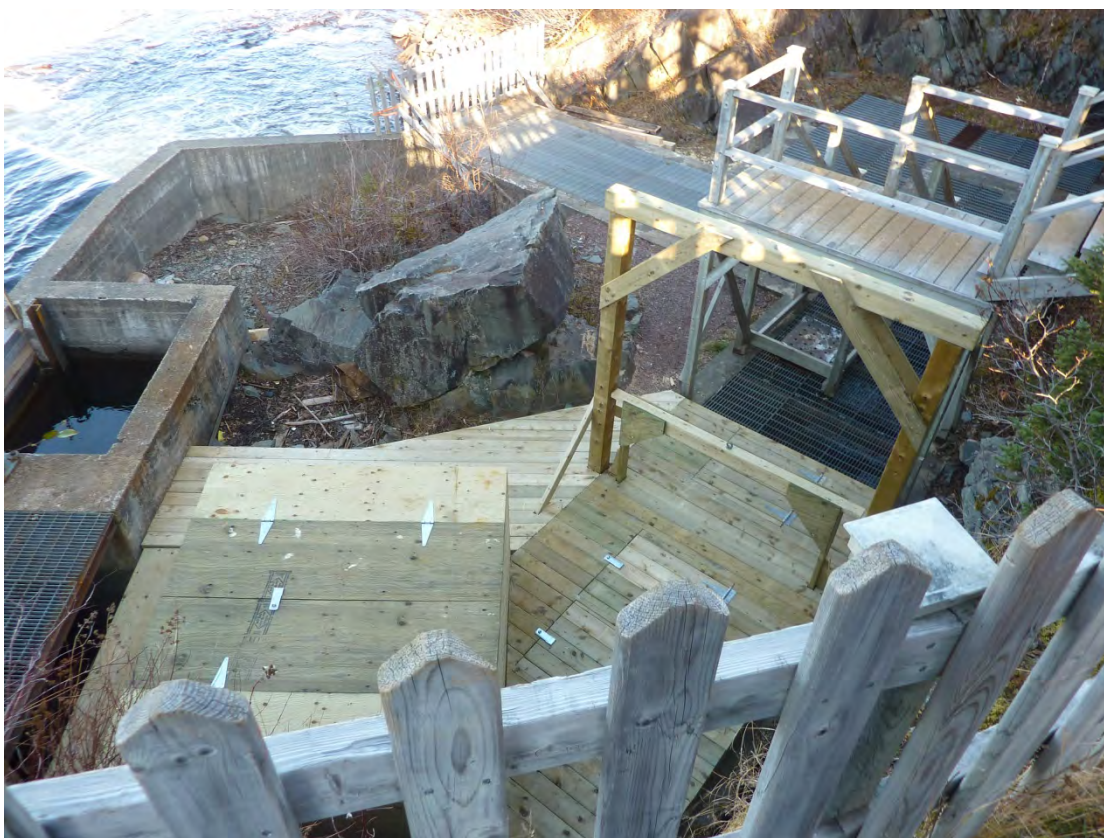
2009 – Overall fishway with timber enclosure over fish trap area
