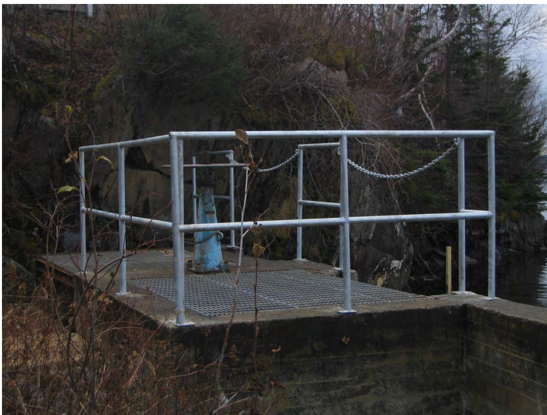
2009 – Steel pipe railing around Pool No. 5 & 6
