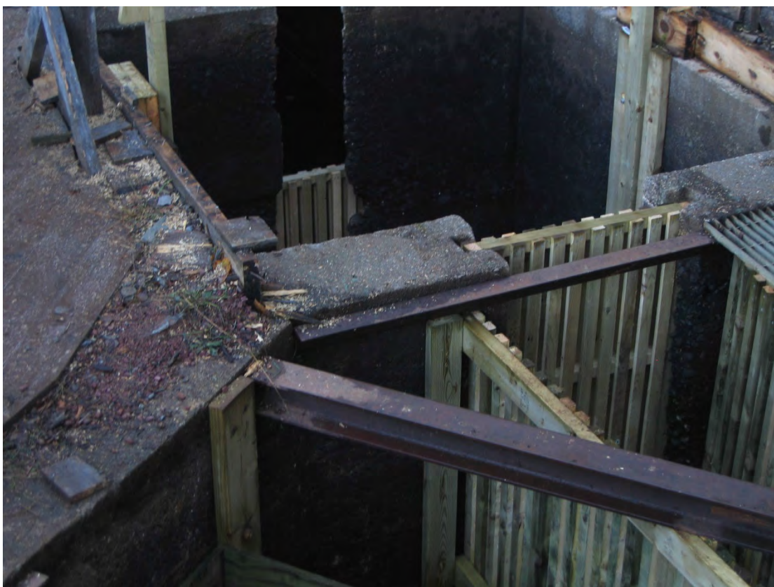
2009 – Wooden fish counting trap without above enclosure (Pools No. 4 & 5)
