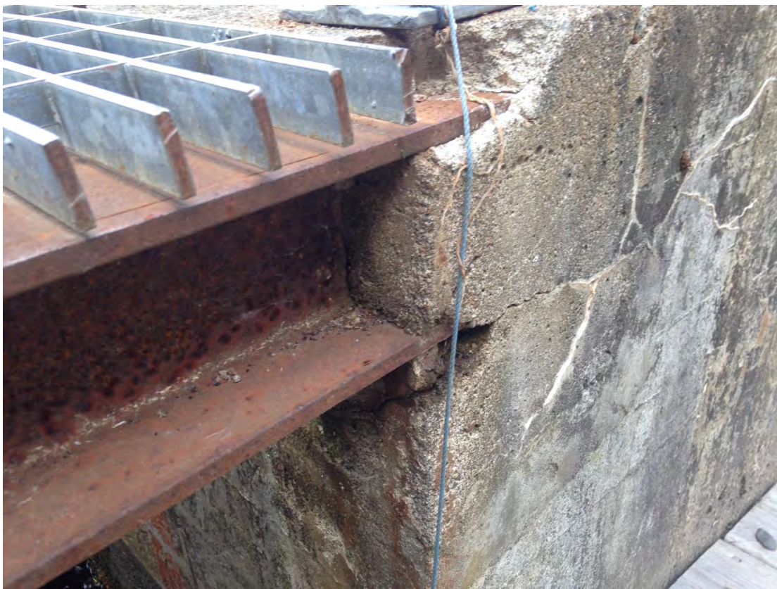
2015 – Embedded steel grating support with concrete damage
