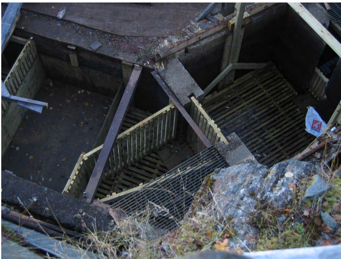
2009 – Wooden fish counting trap without above enclosure (Pools No. 4 and 5)
