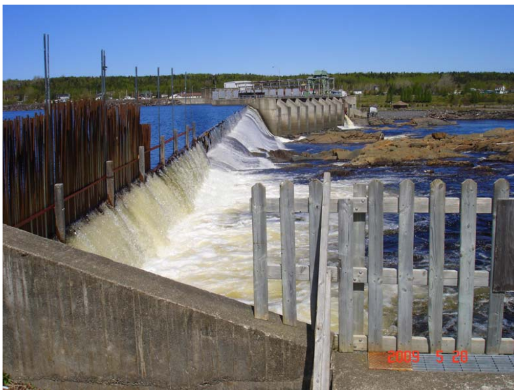
2009 - Downstream of concrete dam near fishway entrance at Pool No. 1. Partially installed steel bar diversion wall constructed over breakaway wall
