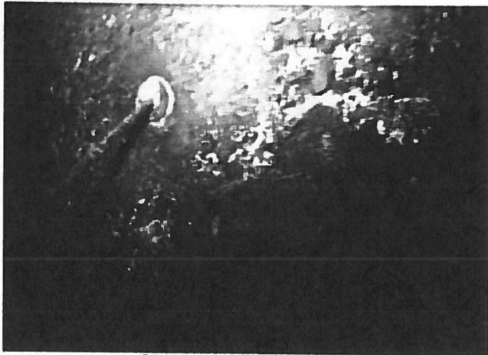
Existing form tie protruding into the pool.
