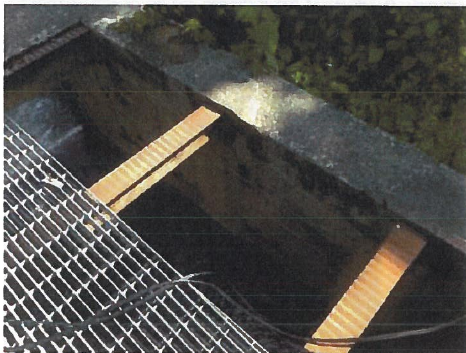
Existing grating with underlying beam supports. Note surface rust on beams and damaged concrete around opening perimeter.
