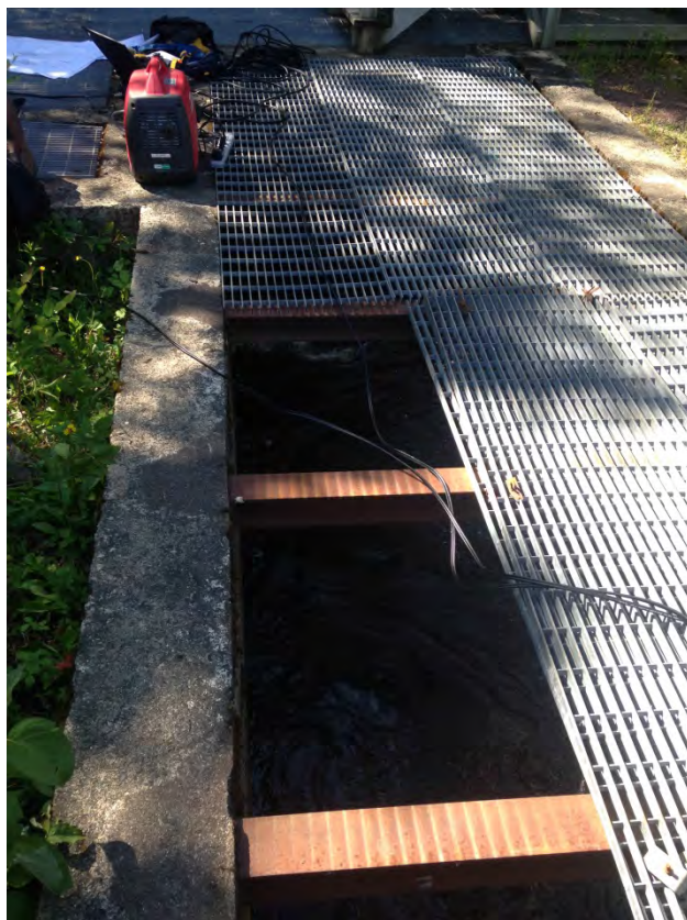
2015 – Pool No. 1 with partial section of grating removed exposing steel supports
