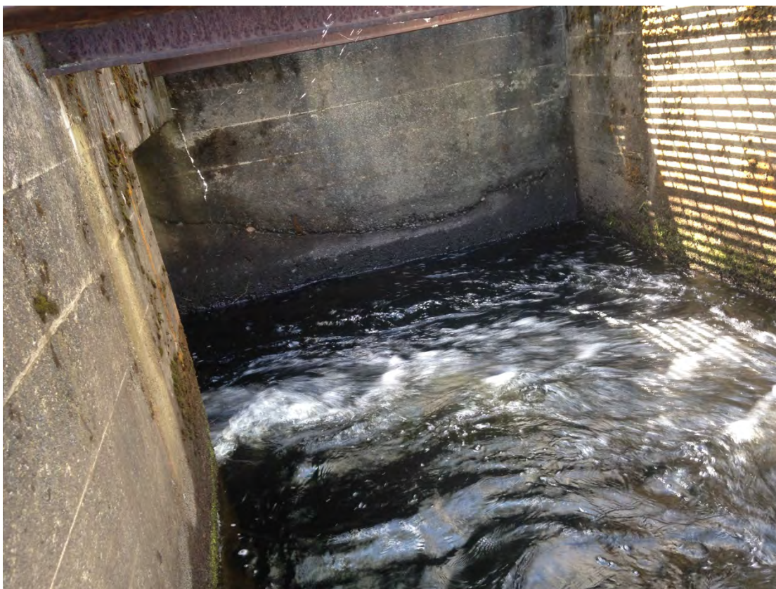
2015 – Concrete deterioration/cracks in far wall
