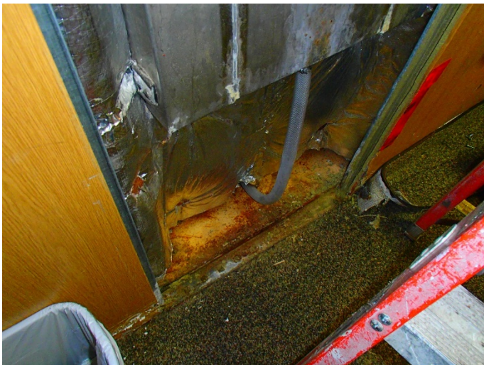
Figure10: Flexible hose connection under reservoir
