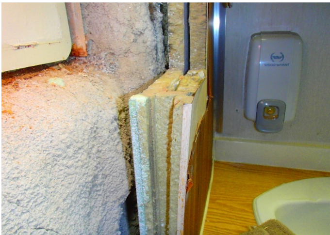
Figure 4: Typical 50mm (2'') Joiner panel
