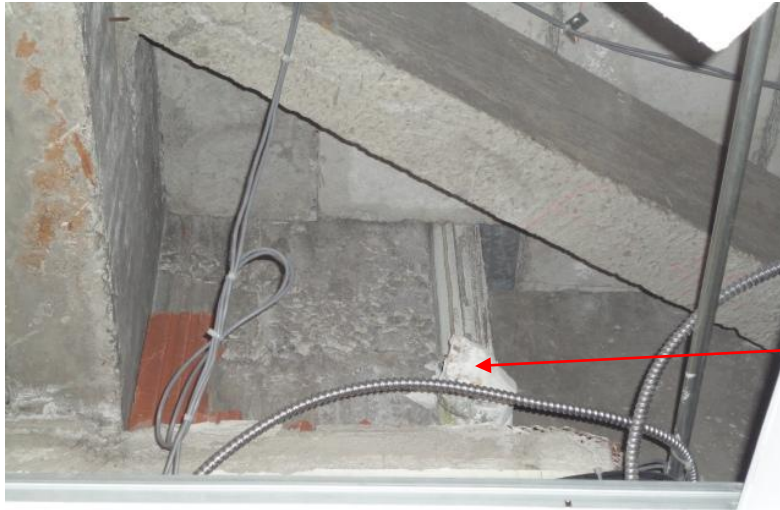
Photograph 5: View of damaged asbestos-containing mechanical pipe fitting insulation observed above ceiling on 5 th floor within closet adjacent to duct and pipe riser.
