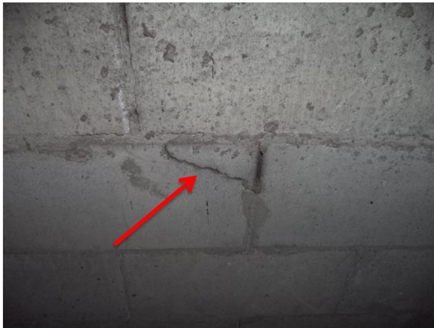
Photo 12: Overview of cracked concrete blocks.
