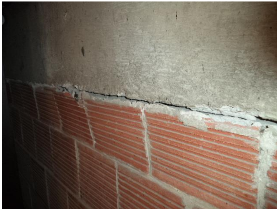
Photo 16: Level 3 loading freight elevator shaft loose clay tiles.
