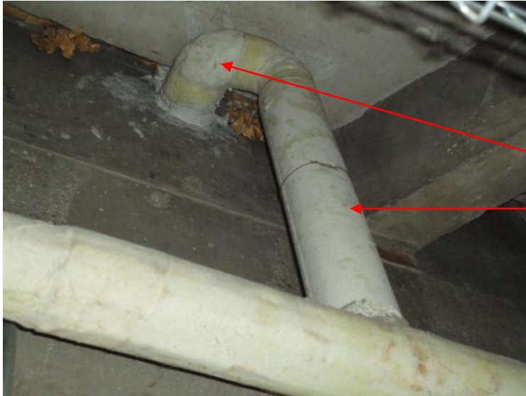
Photograph 1: View of asbestos-containing mechanical pipe fitting and pipe insulation observed on mezzanine within Post Office Work Area.
