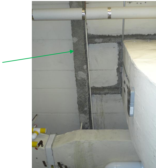
Photograph 8: View of non asbestos sprayed fireproofing and hand patching observed on structural beams within Mechanical Penthouse.
