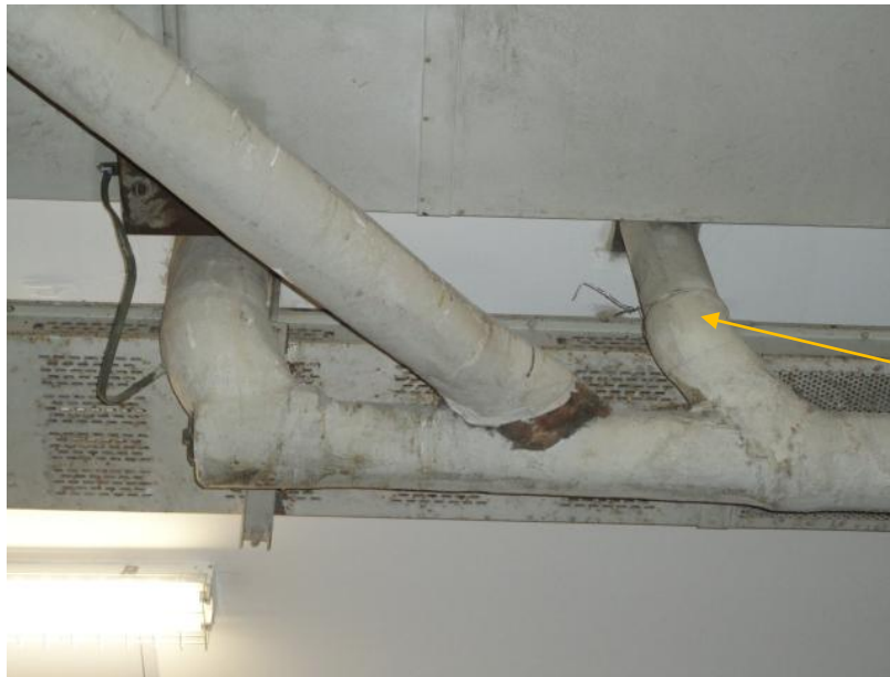
Photograph 12: View of suspect asbestos-containing mechanical pipe fitting insulation observed within the Parking Garage.
