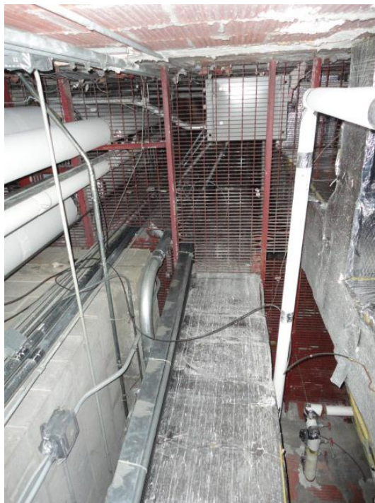
Photograph 10: Typical view of non-asbestos mechanical insulation observed within duct and pipe risers located south of Stairwell E.
