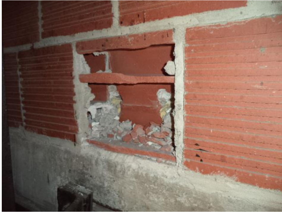
Photo 15: Overview of missing clay tiles throughout the elevator shafts.
