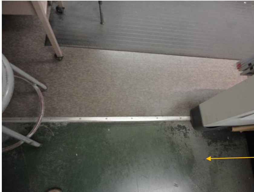
Photograph 13: View of suspect asbestos-containing green flooring observed within the Post Office Work Area.
