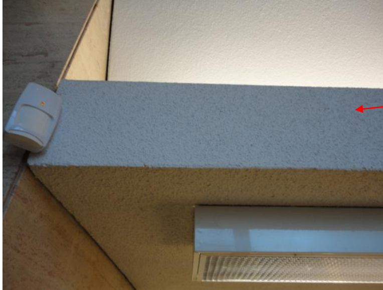
Photograph 3: View of asbestos-containing texture coat observed on ceiling within Post Office.
