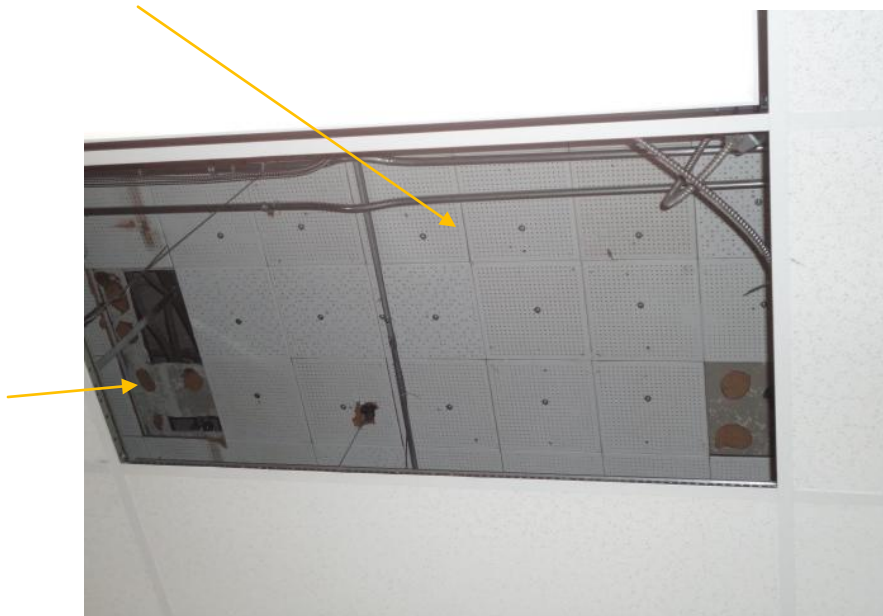
Photograph 14: View of non-asbestos 1x1 ceiling tiles (and associated mastic) observed above lay-in tiles within Post Office Work Area.
