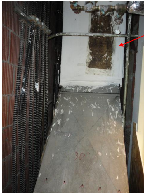
Photograph 4: View of asbestos-containing paper-like duct insulation tape observed to be repaired throughout duct riser adjacent to Stairwell E.
