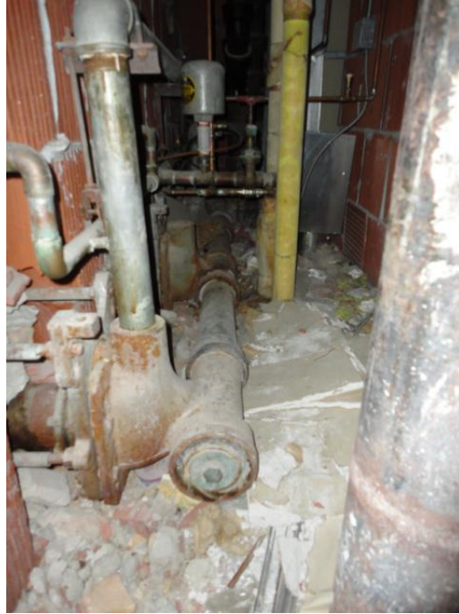
Photograph 11: Typical view of suspect asbestos-containing debris observed within pipe chases within east washrooms.
