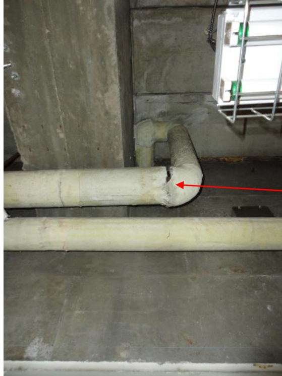
Photograph 2: View of damaged asbestos-containing mechanical pipe fitting insulation observed on mezzanine of Post Office Work Area.
