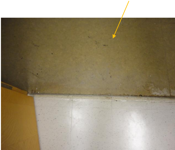
Photograph 15: View of suspect asbestos-containing vinyl sheet flooring observed within closets adjacent to duct and pipe risers within surveyed building.
