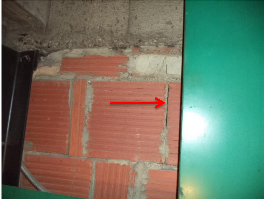
Photo 11: Overview of cracked mortar joints between clay tiles.
