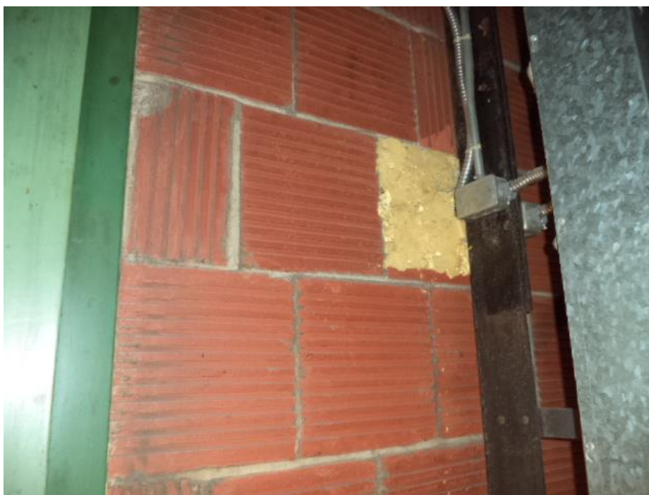
Photo 18: Previous openings filled with firestopping material.
