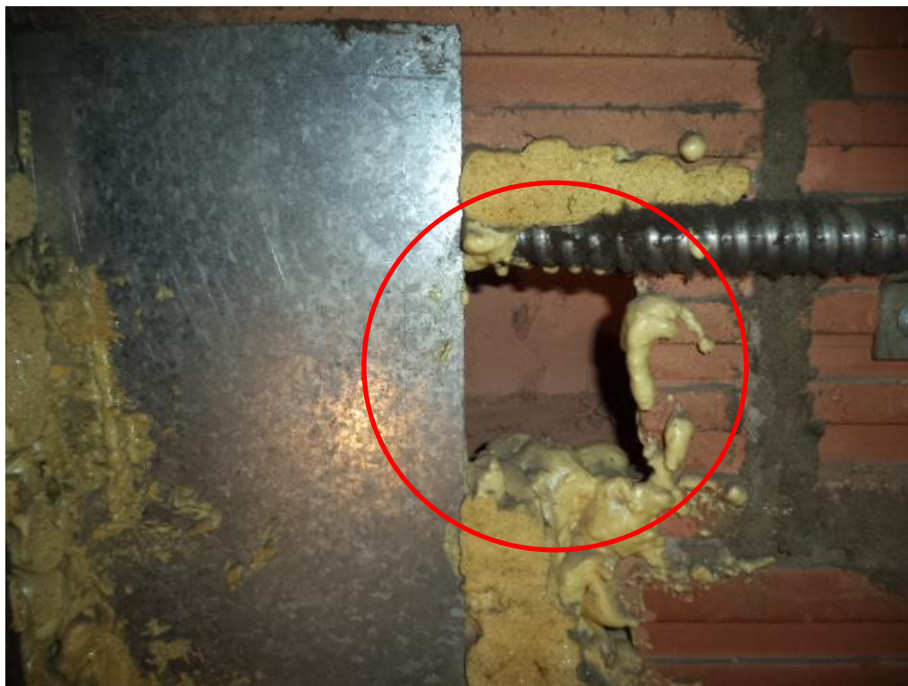
Photo 19: Overview of an area where no fire stopping material was placed.
