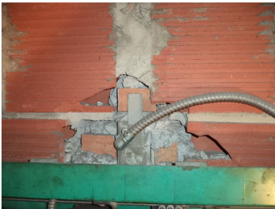
Photo 10: Overview of broken/deteriorated clay block above 10 th level.
