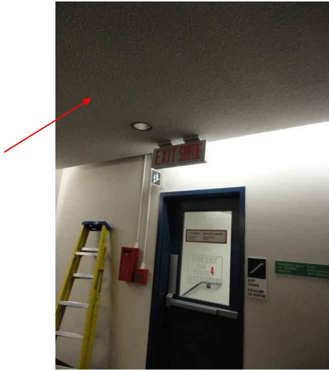
Photograph 7: View of asbestos-containing texture coat observed on 4 th floor Elevator Lobby.
