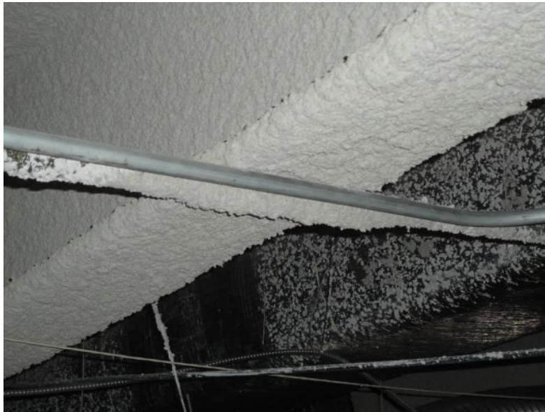
Photograph 9: View of non asbestos sprayed fireproofing observed on structural beams within renovated floors of surveyed building.
