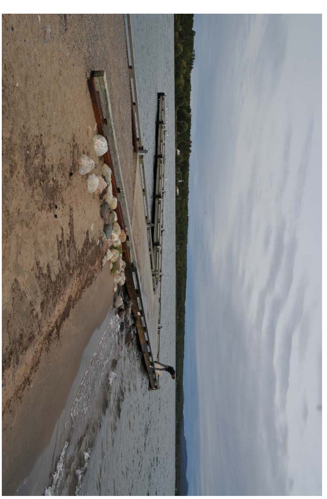
PHOTO OF EXIST ARMOUR STONE PROTECTION SCALE: N/S
