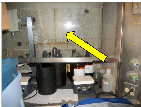
Transite board lining fume hood, Laboratory L530
