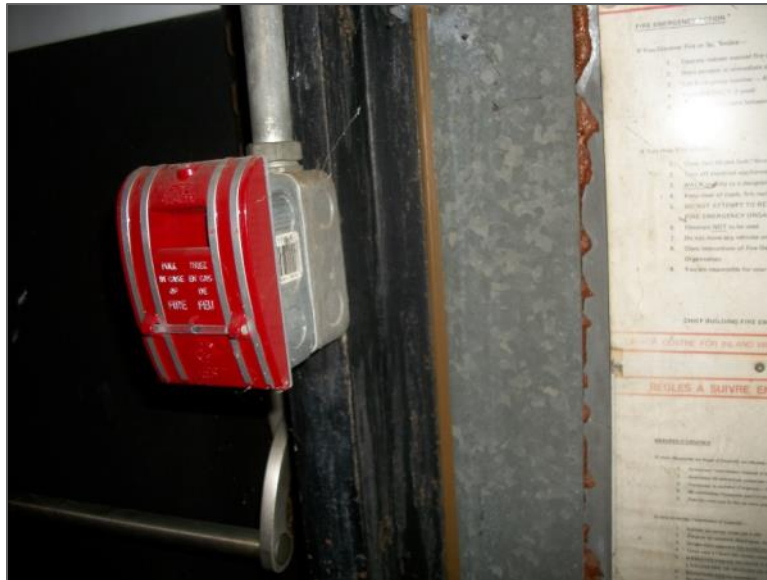
Non-asbestos brown caulking at door frame, WTC Mechanical Penthouse
