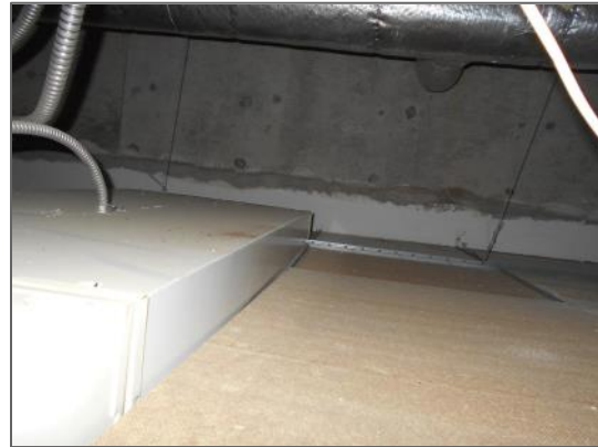
Non-asbestos smooth plaster on exterior wall, Office L529, Fifth Floor
