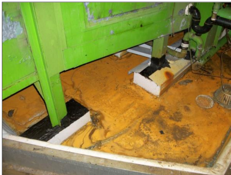
Non-asbestos tar at floor penetrations, R&D Mechanical Penthouse at System 1
