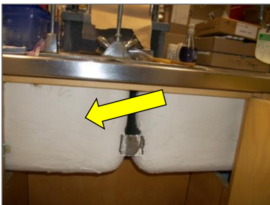
Non-asbestos white sink undercoating, Lab L530
