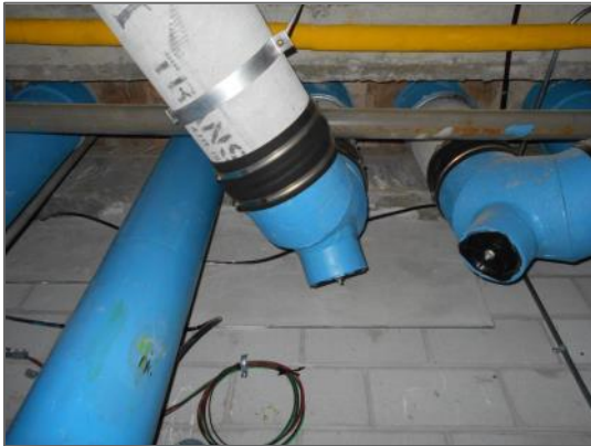
Transite exhaust pipes, Seventh Floor South Service Corridor
