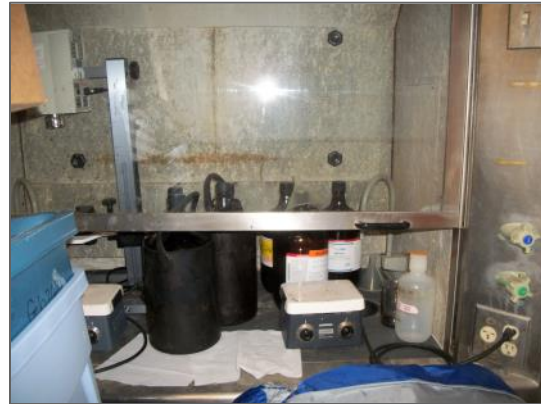
Transite board lining fume hood, Laboratory L530
