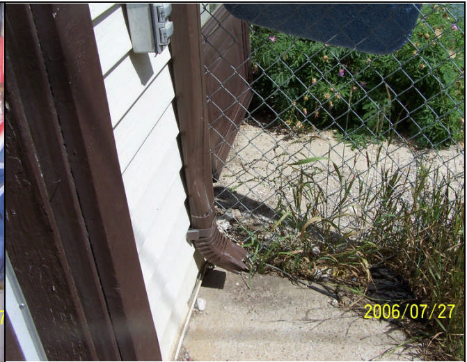
Figure 37: Building Exterior – Eavestrough Drainage Downspout
