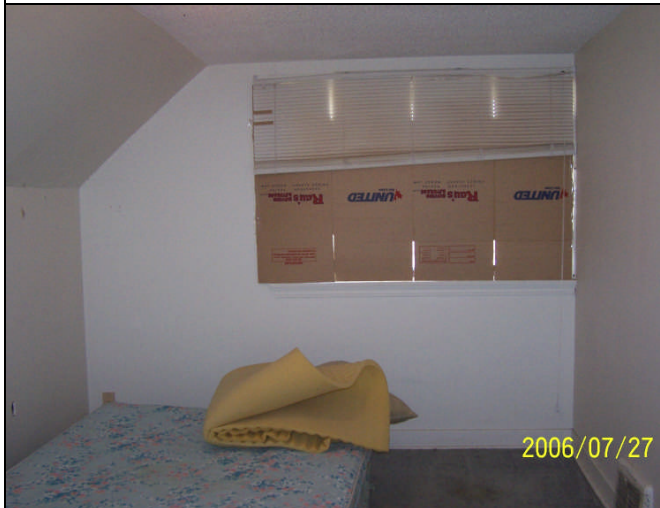
Figure 15: Second Floor Bedroom – Window blocked to prevent cold air entry.
