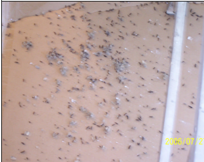
Figure 30: Second Level Hallway – Feces (mouse) fell from Attic onto barrier material when cover over Access Hatch was removed.
