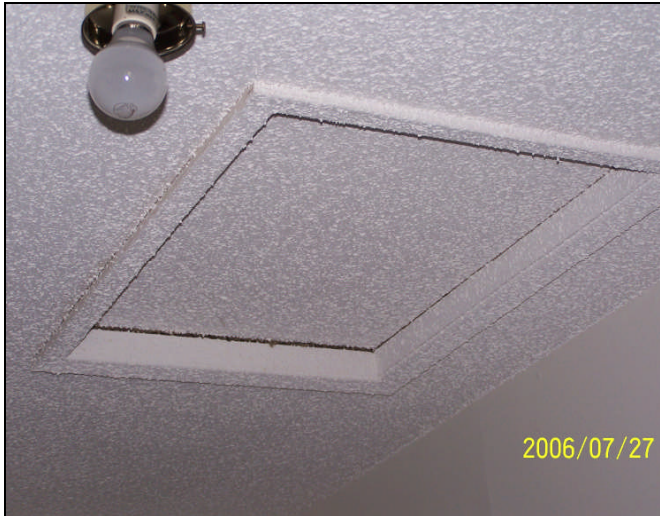
Figure 28: Second Level Hallway – Access Hatch into main Attic area.
