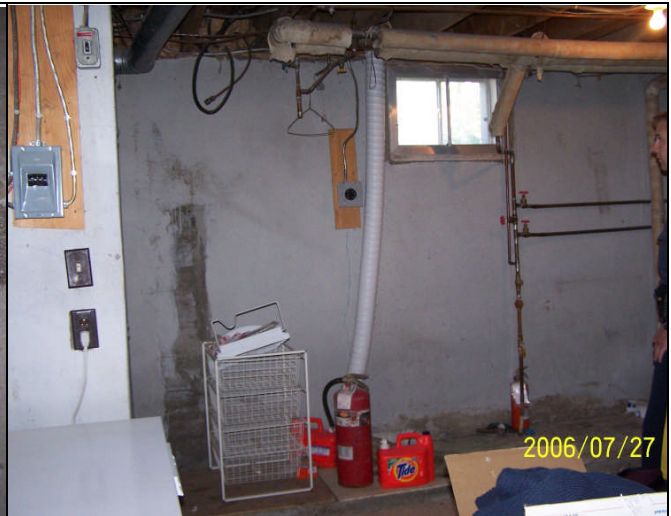
Figure 6: Basement – Former washer/dryer hook-ups
