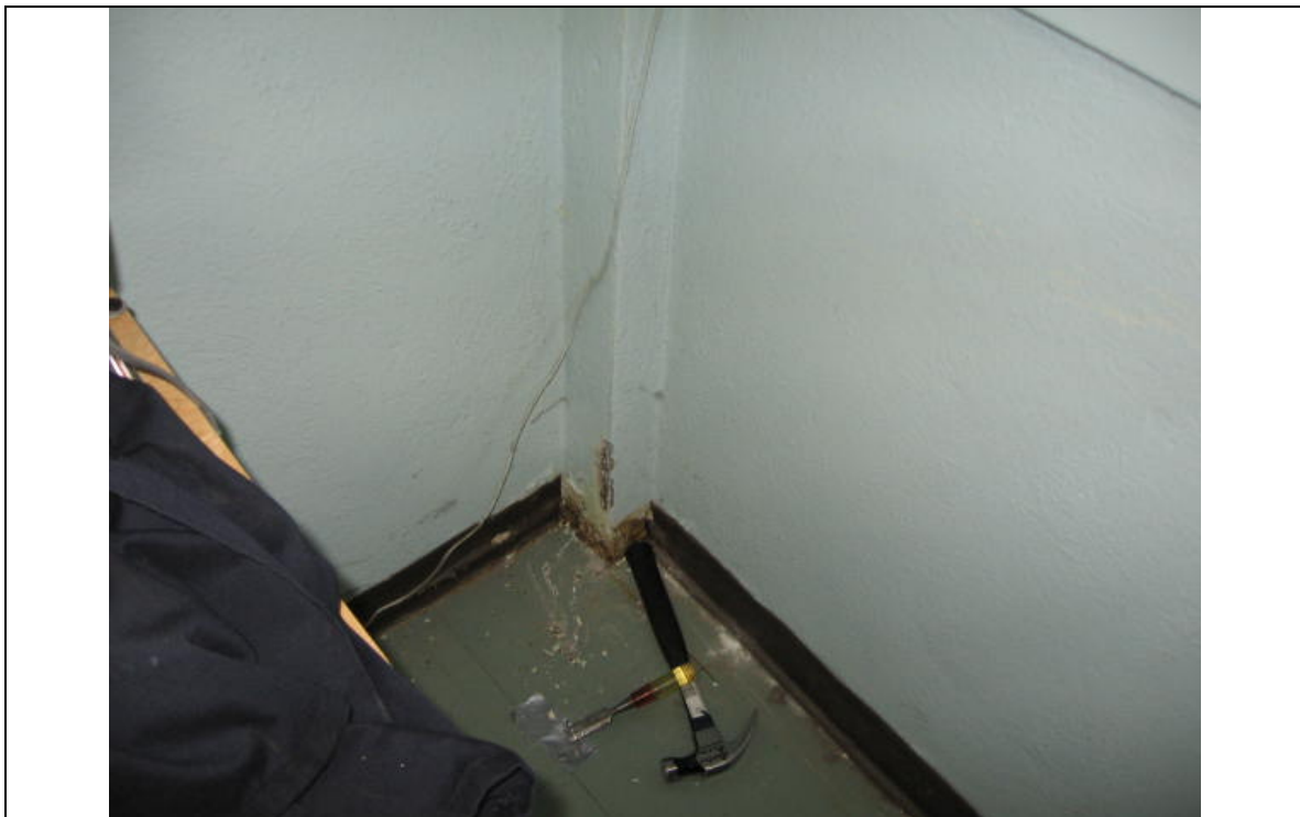
Photograph 18: ACM wall plaster, Room No. SB-1A (Sample No. ACM 50).
