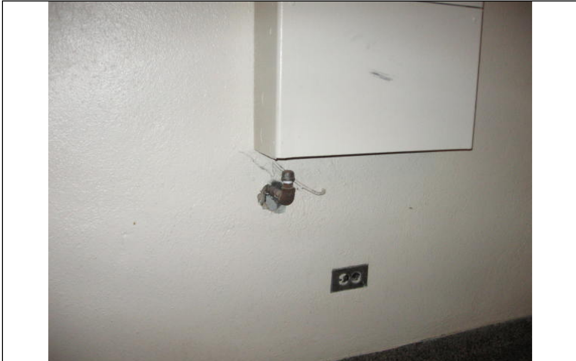
Photograph 19: ACM wall plaster, end of B-level hall (Sample No. ACM 51)
