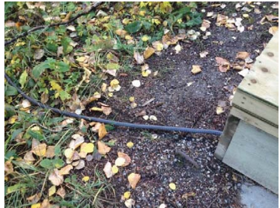
Photograph 4 ↑ Overground Teck Cable from Septic Tank
