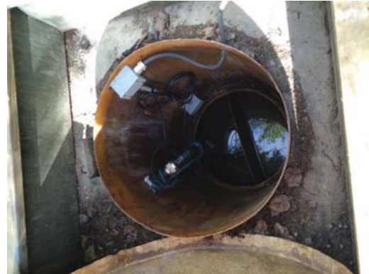
Photograph 2 ↑ Existing Septic Tank and Pump
