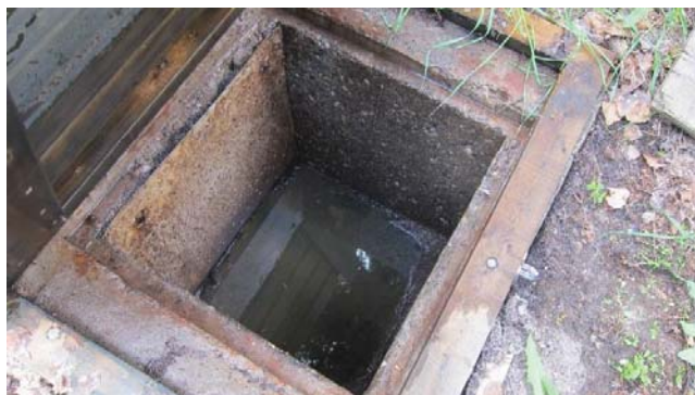
Photograph 3 ↑ Existing Manhole Supplying Septic Field (D/S Tank)
