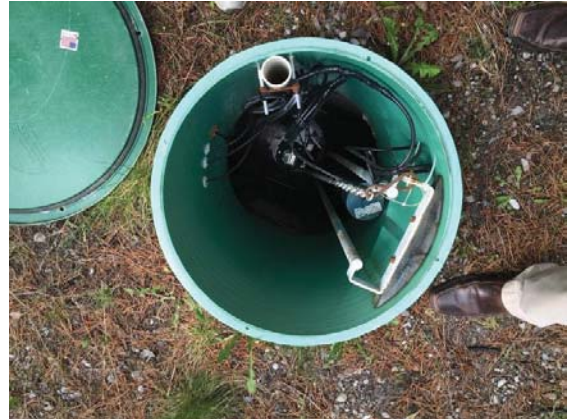
Photograph 2 ↑ Completed Septic Tank Pump in Riser
