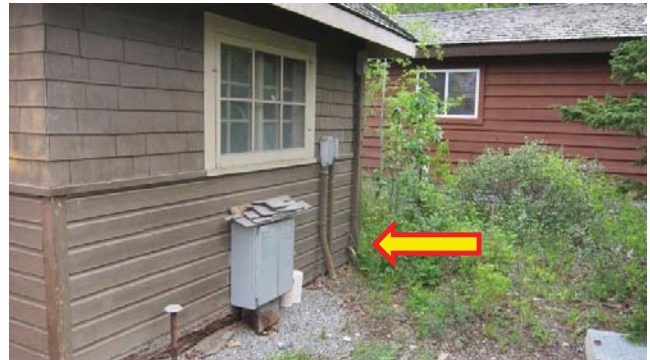
Photograph 8 ↑ Teck Cable Entry into Electrical Building
