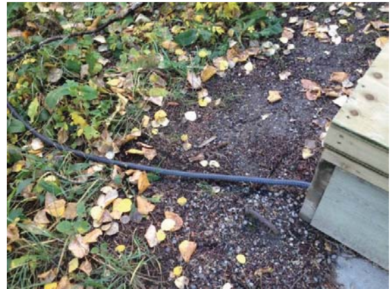
Photograph 4 ↑ Overground Teck Cable from Septic Tank
