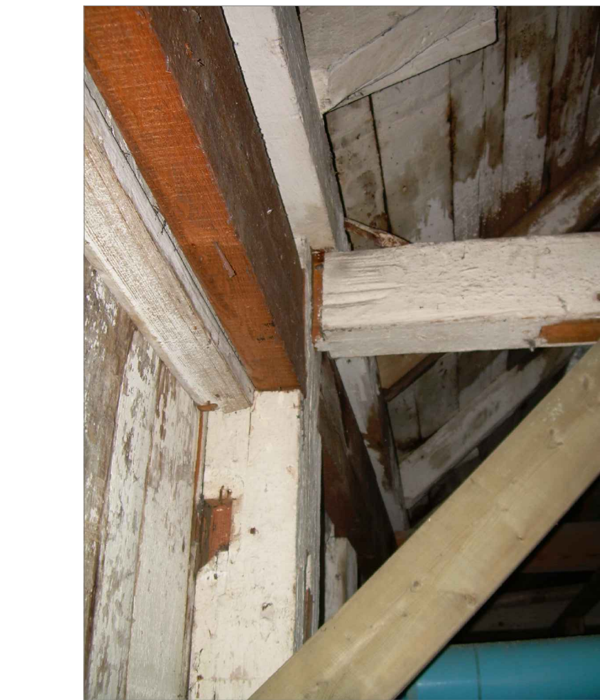
TIE BEAM OUT OF ITS GROOVE ON AXIS 6
