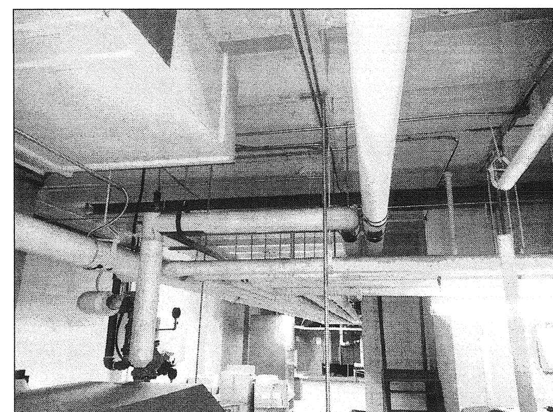
3 EXISTING PENTHOUSE PHOTOGRAPH #2 E208 NOT TO SCALE
