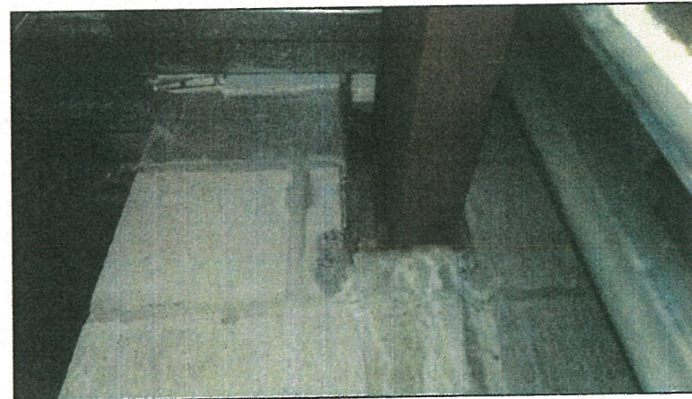
EXISTING BEAM SUPPORT AT SOUTH BLOCK WALL
